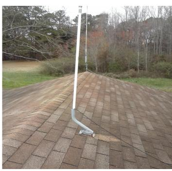
Steve KA4CZL had an old satellite dish mount he wanted to do something with. So he used it to mount a VHF/UHF antenna. Nice job on recycling and using it for amateur radio.
