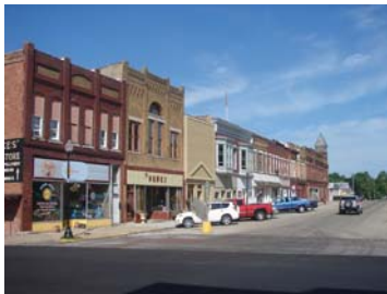
The historic streetscape bordering the town square in Virginia features active commercial buildings.
