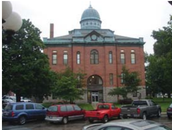
Menard County Courthouse (1896).
