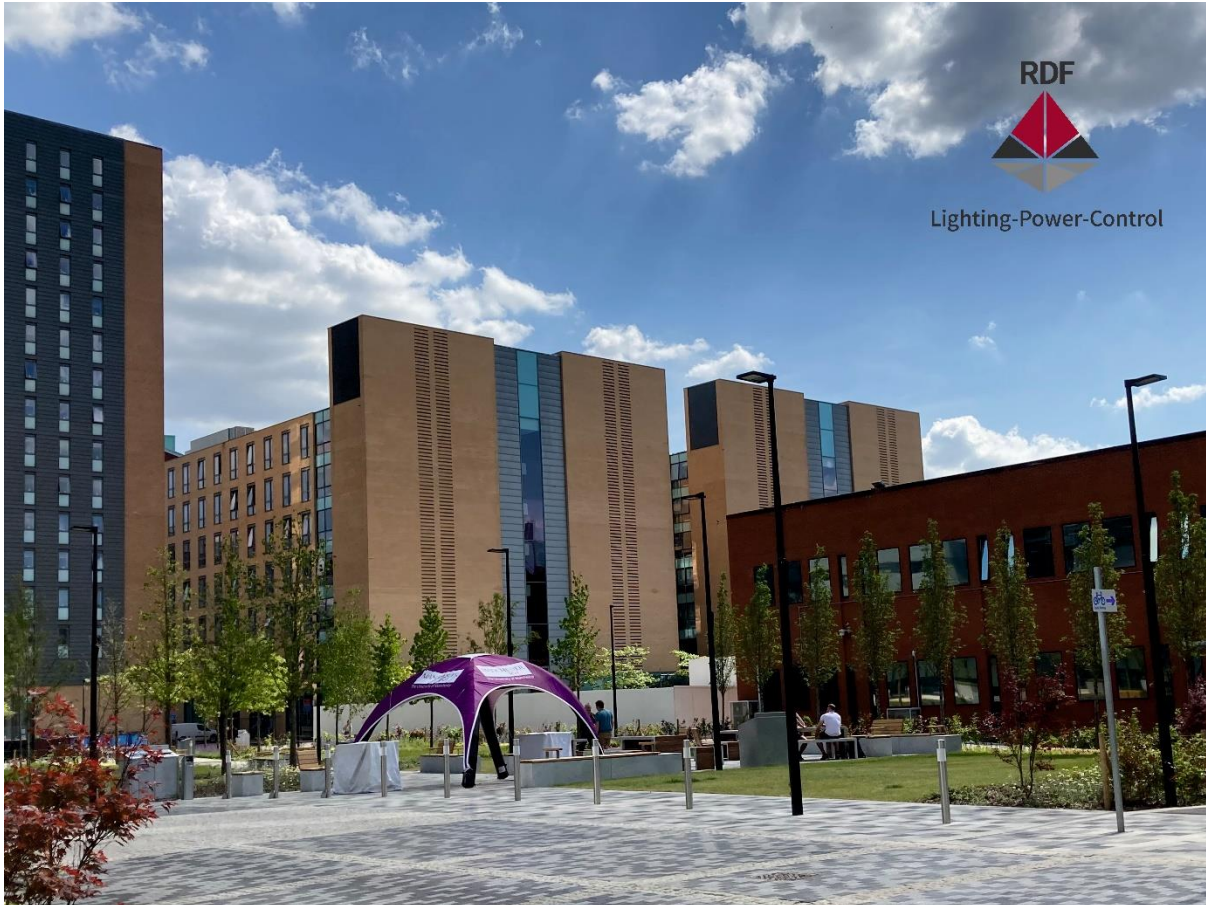
University campus building
