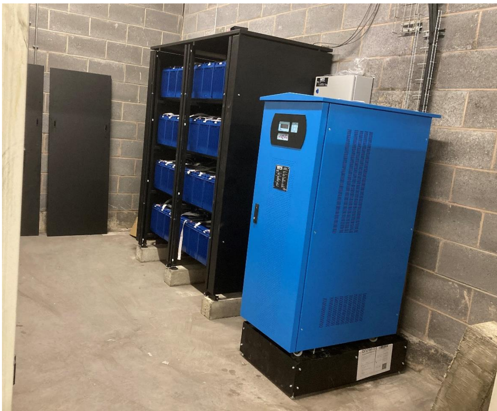
Power Pro 3-Phase inverter and battery rack installed at the University
