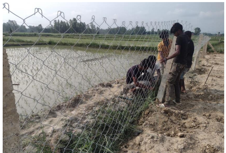
VC-1 fencing being installed. Both the fence material and posts are handmade. The fence has to be made high to exclude deer.
