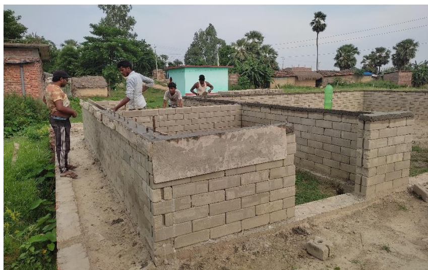
Building works underway at Pasman Tol. Note the use of eco-bricks – bricks that are made using the cold compression of cement and sand.
