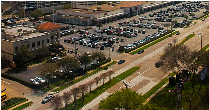
Significant parking restricts access to shopping
