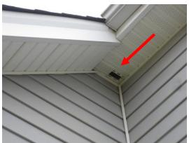
There is a section of the soffit vent missing on the rear left side of structure. This condition may allow rodents and pests to enter and nest in the structure cavity and/or attic. Recommend section be installed by a professional in the business
