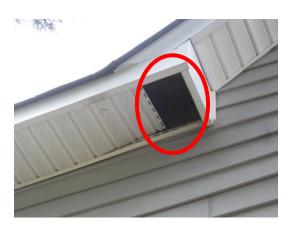
There is a section of the soffit vent screen missing on the right rear side of the property. This condition may allow rodents and pests to enter and nest in the structure cavity and/or attic. Recommend section be installed by a professional in the business
