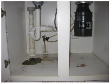
Cabinet below kitchen sink has water stains and bacterial growth. This is possible indication of a prolonged water leak from the drain or water supply. Condition could not be inspected due to lack of water supply to the residence during inspection. Recommend a professional in the business inspects and repair condition
