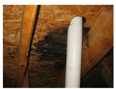
There is bacterial growth noted below the PVC vent in rear of the attic. Condition is indicative of water infiltration from the roof system. It is recommended to have a professional in the business inspect conditions and repair/replace accordingly
