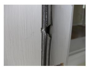
The main door trim is damaged, cracked or frail. Damaged weather seal prevents proper insulation and separation of living space from exterior resulting in added energy usage and possible entry points for rodents and pests. It is recommended for the weather seal of the main entrance door be replaced by a professional in the business
