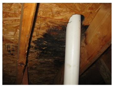
Figure 3: OSB Stains in Attic below Vent Pipe
