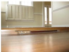
The laminate floor edge between the living and dining room as well as between the kitchen and foyer is damaged. This may result in a tripping hazard and shall be inspected and repaired by a professional in the business
