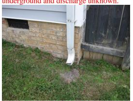
Downspouts are missing splashguards to channel water away from foundation. Water in close proximity to the foundation may result in differential settlement and structural damage. Recommend installing splash guards on all downspouts
