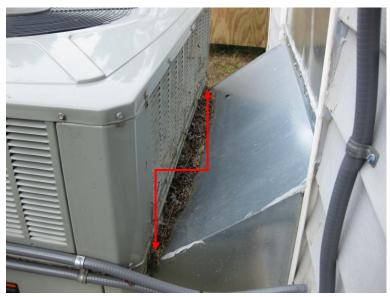
The exterior HVAC system as well as the NG premanufactured fireplace exhaust flue shall be checked and cleaned of dry vegetative debris prior-and-during heating season to prevent spontaneous ignition of dry vegetative debris accumulated above device
