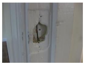
The strike plate of the master bedroom door is missing from the door frame. This condition prevents proper latching of door and results in additional damaging of the door frame. Recommend a strike plate be installed by a professional in the business
