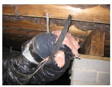
Flexible insulated ducts in crawl space are damaged, sagging or loose from hanger straps and/or separated from the metal distribution boxes. This condition results in inefficient use of the HVAC system preventing proper conditioning of living spaces of the property and increase consumption of energy
