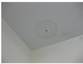
There is a water stain in the rear right corner of the master bedroom walk-in closet. This may be an indication of some water infiltration from the attic. Recommend condition be inspected and repaired by a professional in the business
