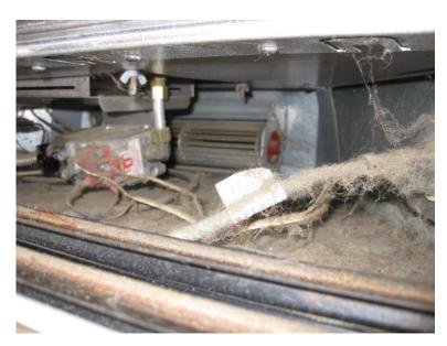
NG fireplace mechanical chamber is dirty and in need of cleaning. Existing condition may result in spontaneous ignition of dust and dirt. It is recommended for the mechanical chamber to be cleaned by a professional in the business before the use of the fireplace
