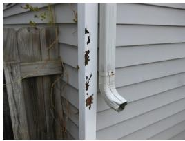
There are sections of the vinyl trim damaged on the rear right side of the property. The picture also illustrates how a downspout discharges about three (3) feet above ground resulting in water being in close proximity to the foundation. Picture also illustrates a shrub growing between vinyl trim and cladding. Unattended, these conditions may result in deterioration of structural components and settlement of foundation
