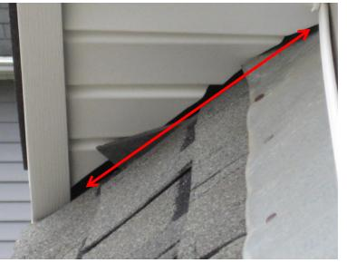
Figure 4: Missing Flashing on Front 'Water-Table'
