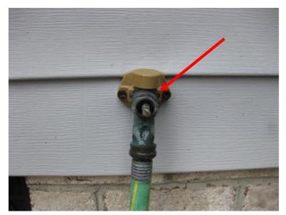
Exterior front water faucet is missing knob making opening and closing the faucet difficult.
