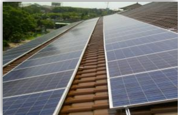
Figure 2. On-grid Installation in
