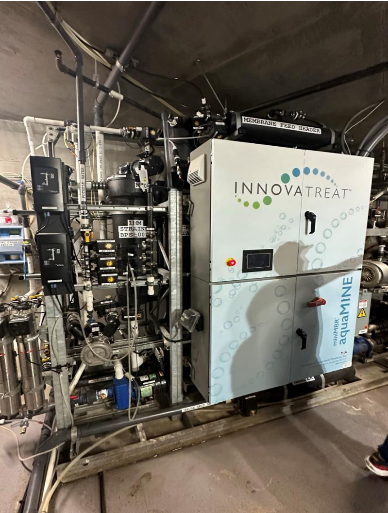
Membrane Filtration Skid
