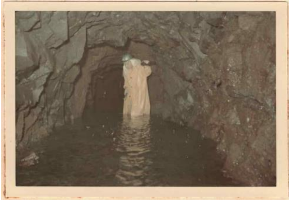
“View looking towards portal at about 1000-feet in Ha'ikū Tunnel showing saturated rock in foreground and dike at STA 9+80” (Bowles, 1969)
