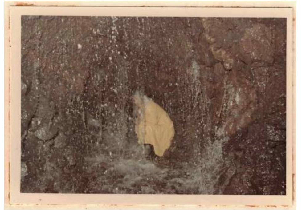
“View of Ha'ikū Tunnel heading, majority of discharge is from drill holes in clinker” (Photograph from Bowles, 1969)
