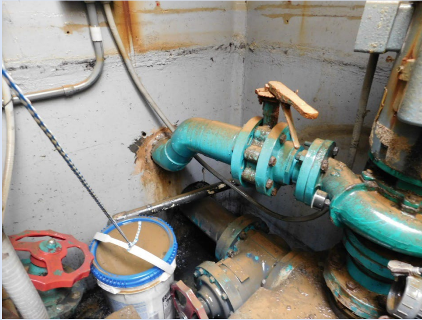
Piping vault wall penetration.
