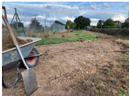
The ground had to be rotavated to clear the grass away.
