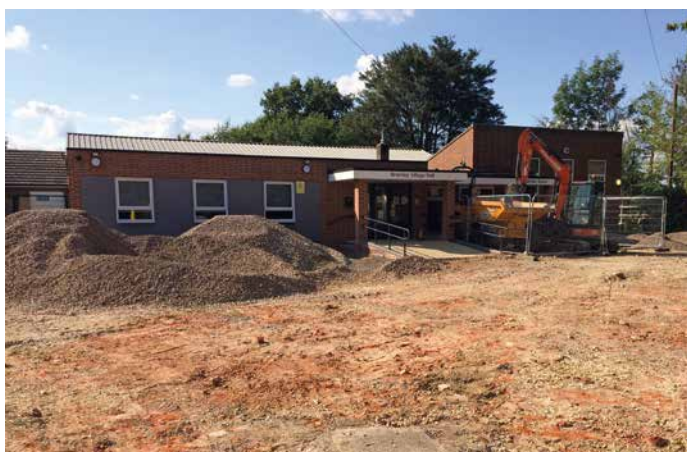
New, washed stone ready for the SuDS
