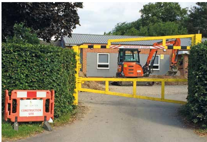
The work begins.....
