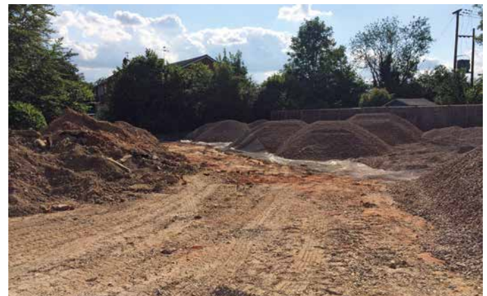
Spoil to the left, new stone to the right
