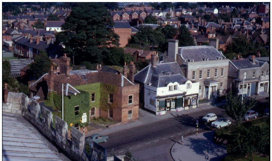
Church Street - all demolished for the new shopping centre
