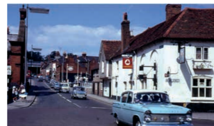
1964 Brook Street Junction – now Churchill Way Dual Carriageway
