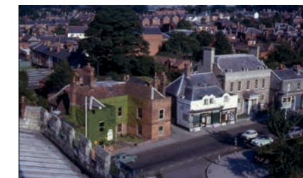
Bottom of Church Street- now all demolished
