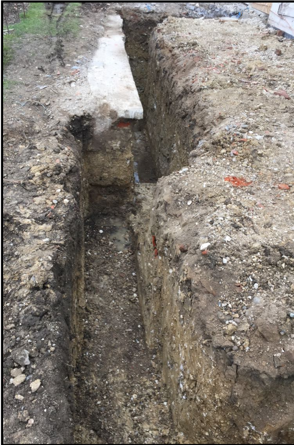
Plate 3. View of Trench 3 & 4 facing south showing foundation of demolished extension (002).
