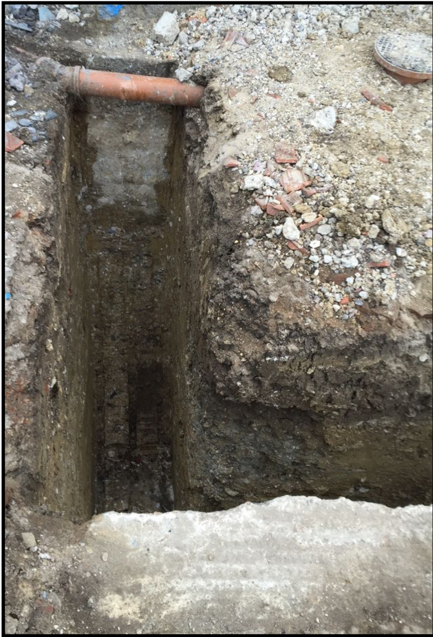
Plate 1. View of Trench 1 facing west showing foundation of existing house (003)
