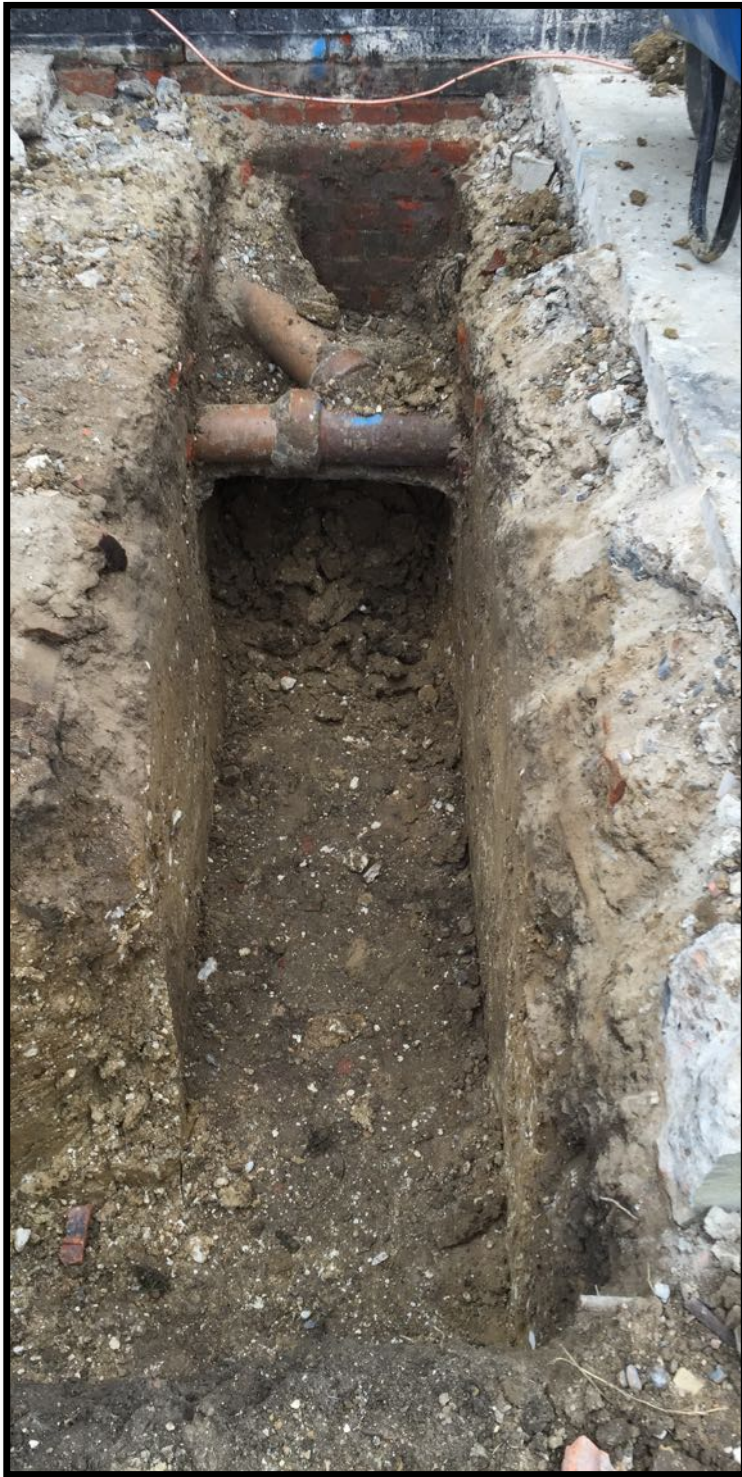
Plate 6, View of Trench 4 facing west showing existing foundation of building (003)
