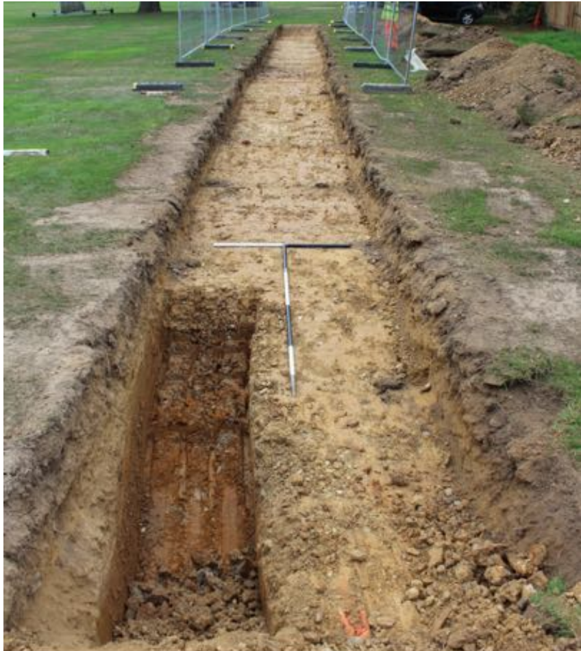
Plate 6: Trench 3 facing northeast
