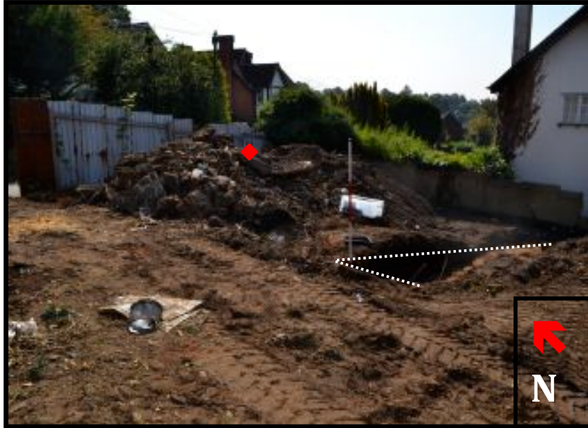
Area 1 viewed facing East with Trial Trench 1 and East spoil heap ◆ in view
