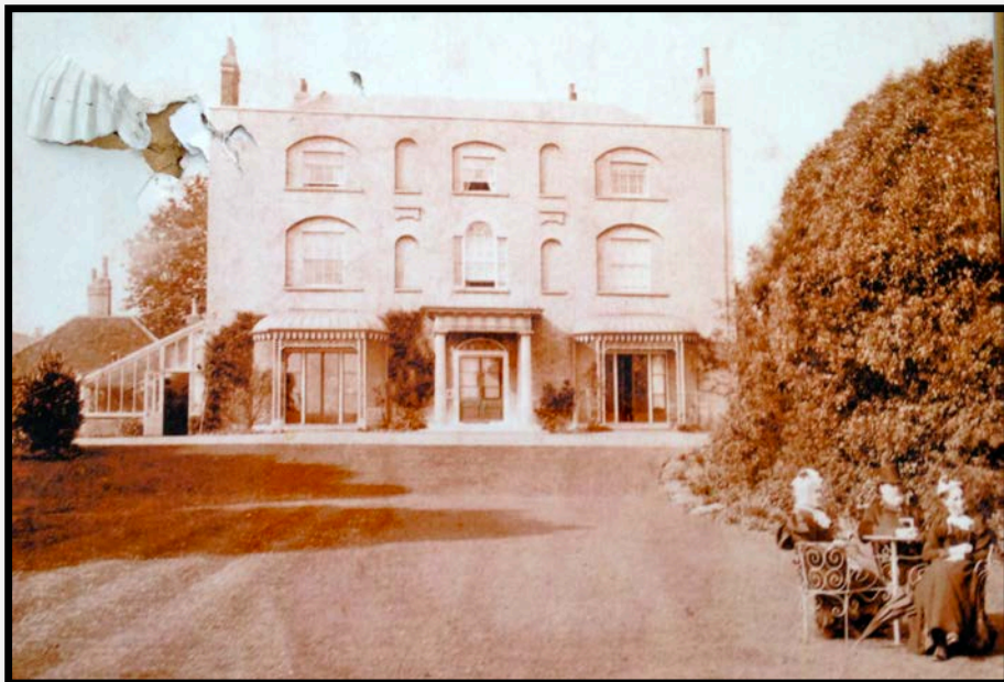
Fig.48. Rear of house C18th/19 th showing conservatory to the West elevation
