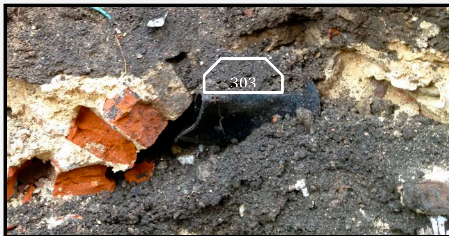
Fig.41. Remains of damaged Victorian arched drainage culvert filled with modern rubbish.
