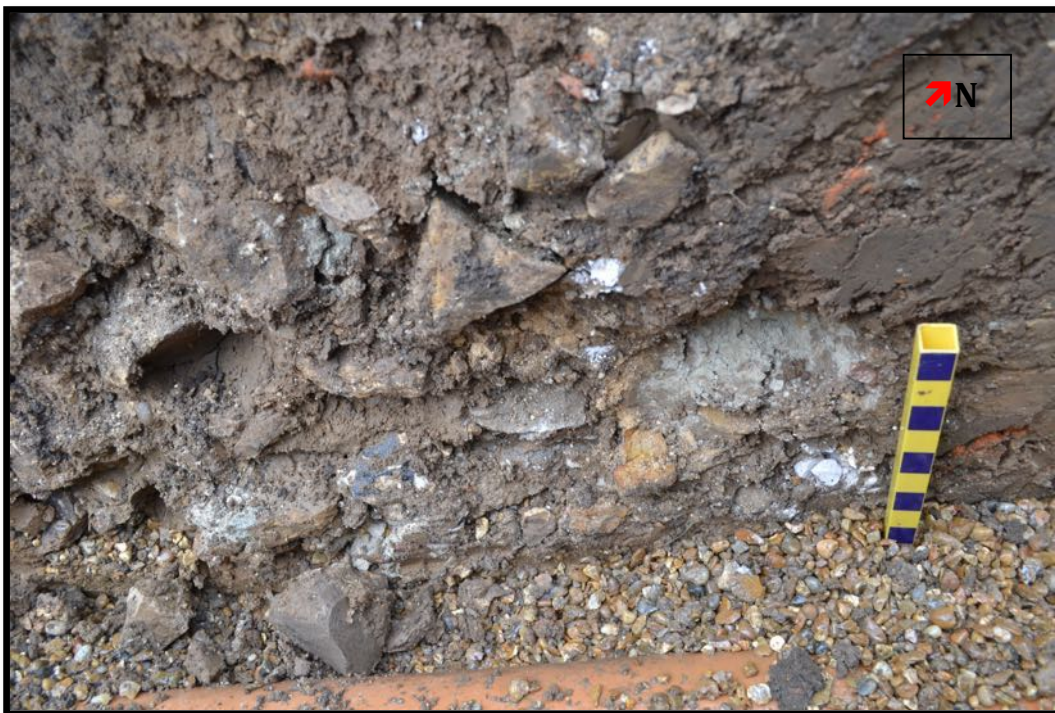
Plate 9. Drainage Trench 3 - Debris (310) viewed in west section
