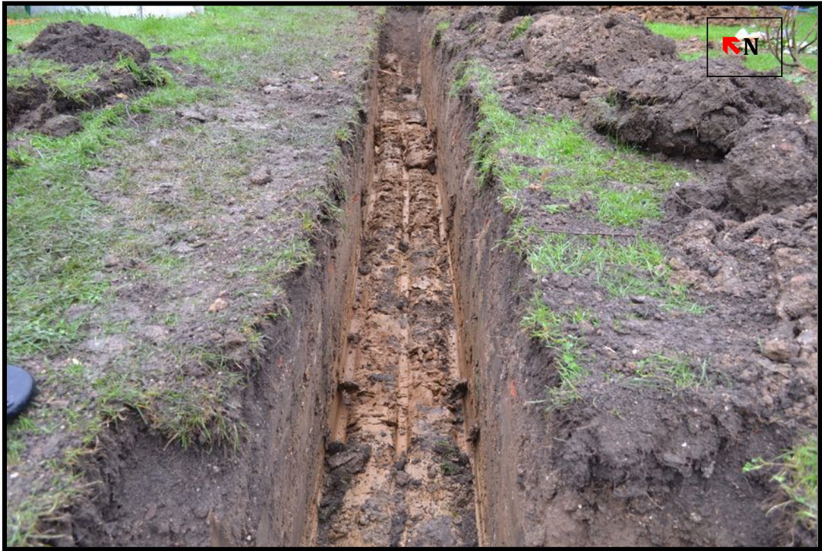
Plate 13. Drainage Trench 4 Facing North
