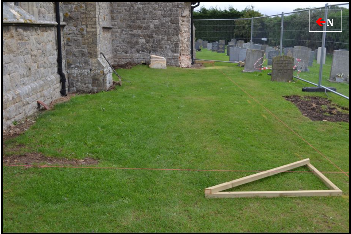
Plate 2. General View of Site Facing East – Trench 1 & 2 set out.
