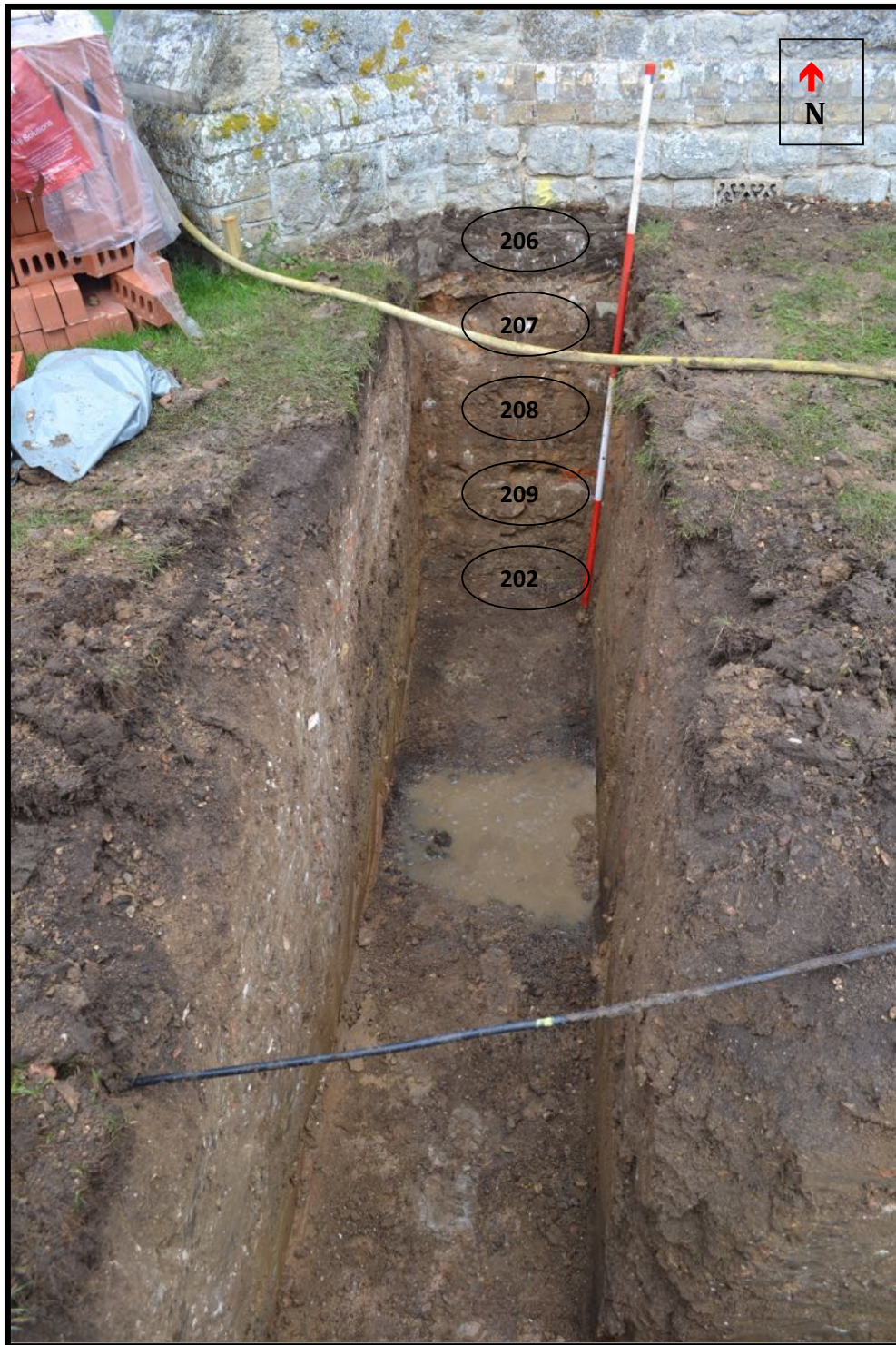
Plate 5. Foundation Trench 2 Facing North – Church foundation
