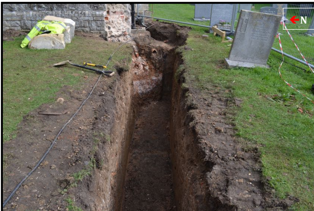
Plate 3. Foundation Trench 1 Facing East – Buttress foundation and drainage pipe
