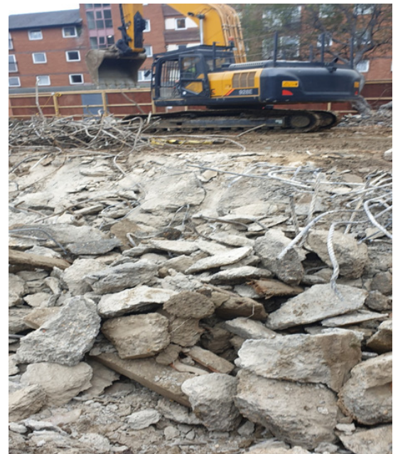
Breaking Out Ground Floor Slab
