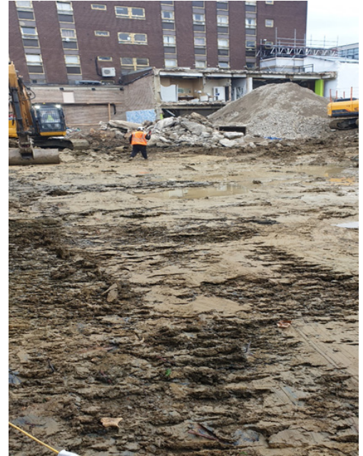
Excavation For Piling Mat
