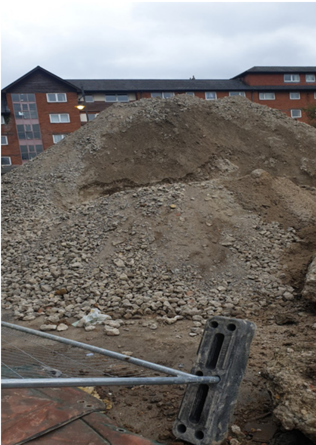
Demolition waste recycled for piling mat
