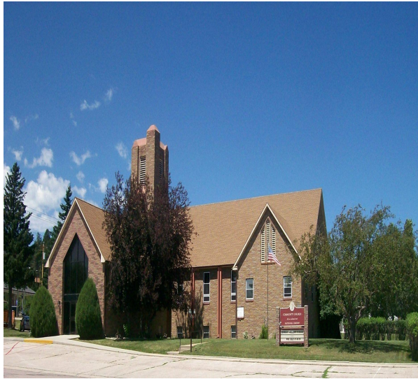
Church Building - Exterior
