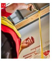
1.2 Check at least three height dimensions - both jambs and in the centre of the opening.
