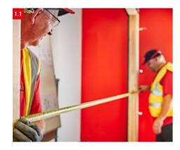
Measure the frame and opening (before removal of an existing frame if it is a refurbishment) and check at least three dimensions horizontally
