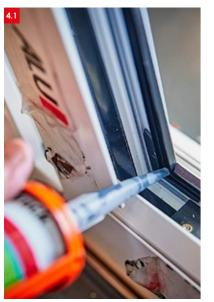
Check the captive glazing gasket to ensure it has been fully fitted with no gaps at the corners then seal the corners with a butyl based sealant.
