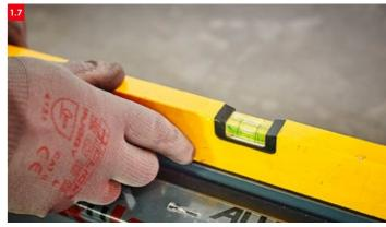
Recheck to ensure the cill is level and proceed to fix to substrate. Remember "check twice, fix once".
