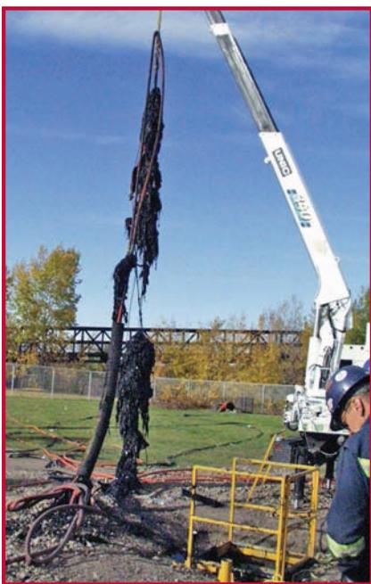
**The 28-foot length of fibrous debris completely free of the manhole.**
