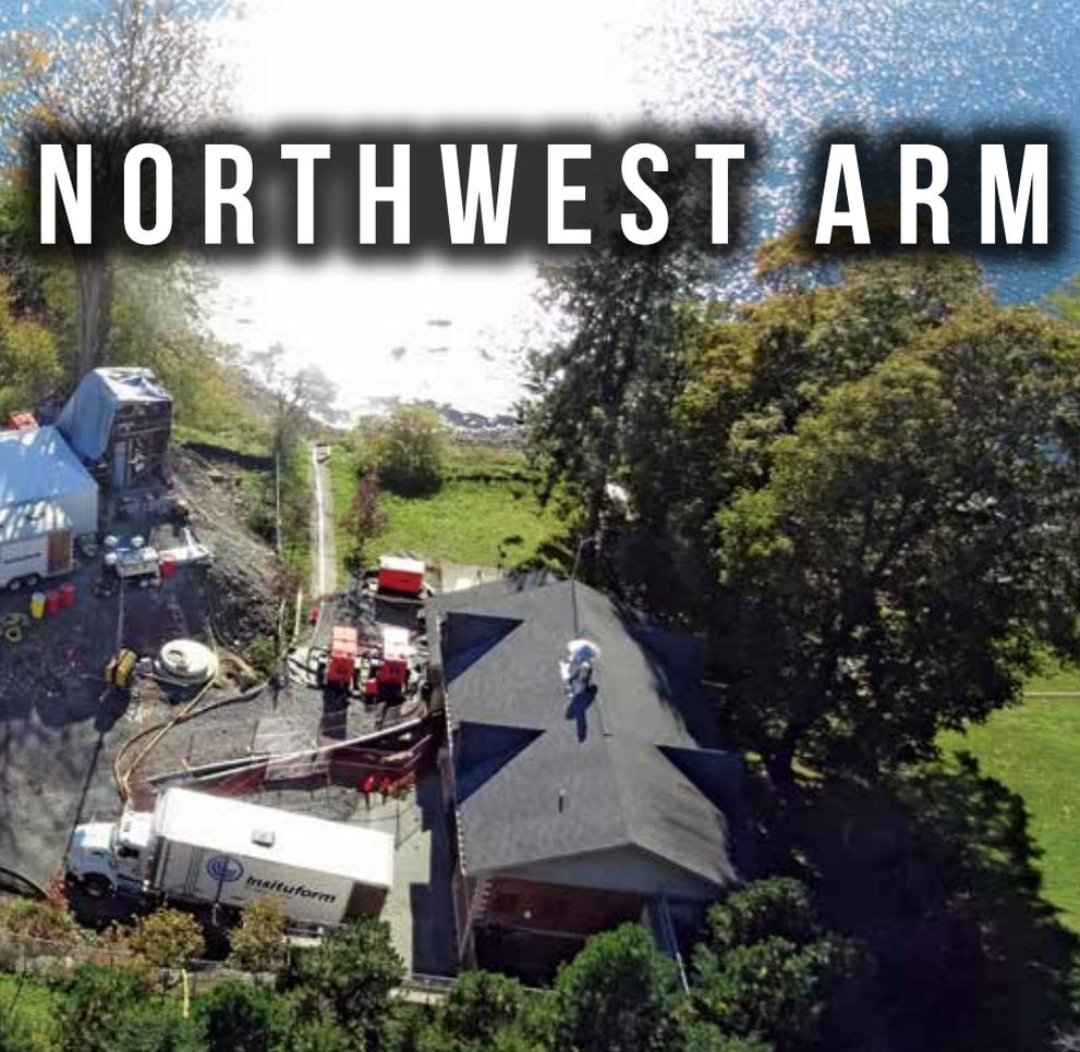
of the pipe and limited work space along the Arm, Insituform CIPP proved to be the best product and method.
