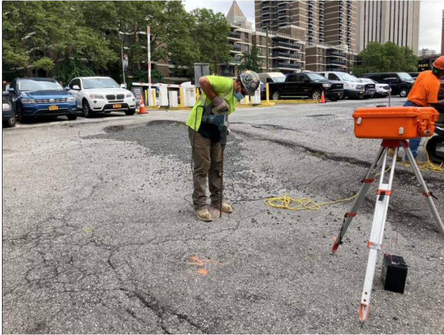
Photo 1: AARCO advancing a handheld hammer drill into a suspected void space (facing west)
