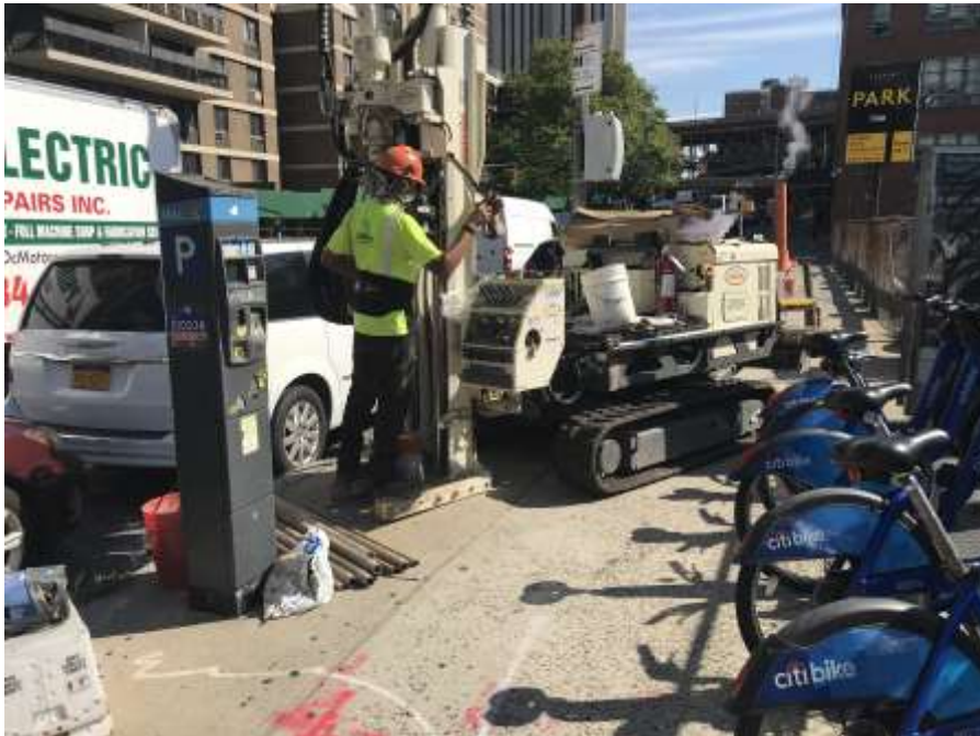
Photo 4: AARCO advancing boring SB39 (facing east)
