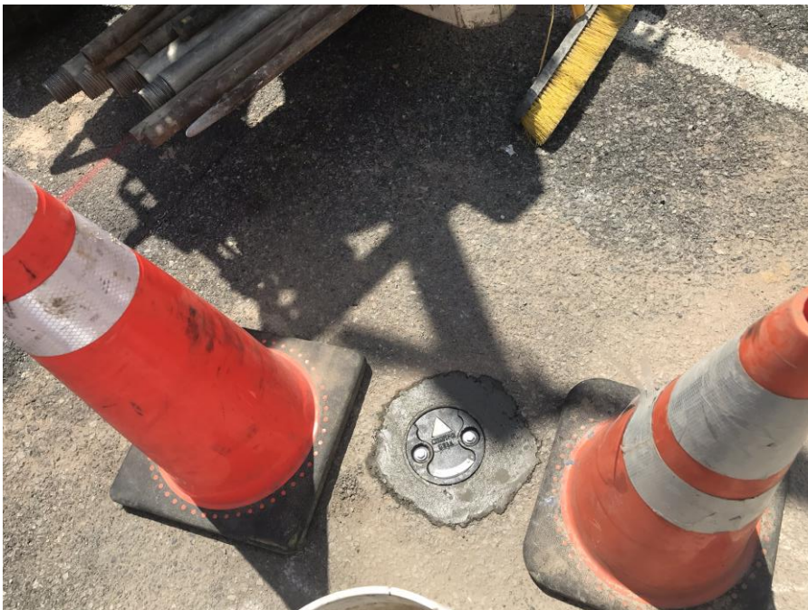
Photo 2: Monitoring well MW25 installed by AARCO
