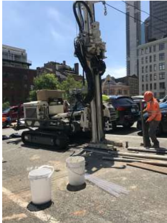
Photo 1: AARCO advancing soil boring SB4W1 (facing southwest)
