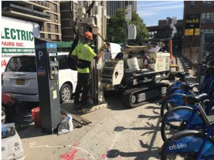
Photo 4: AARCO advancing boring SB39 (facing east)
