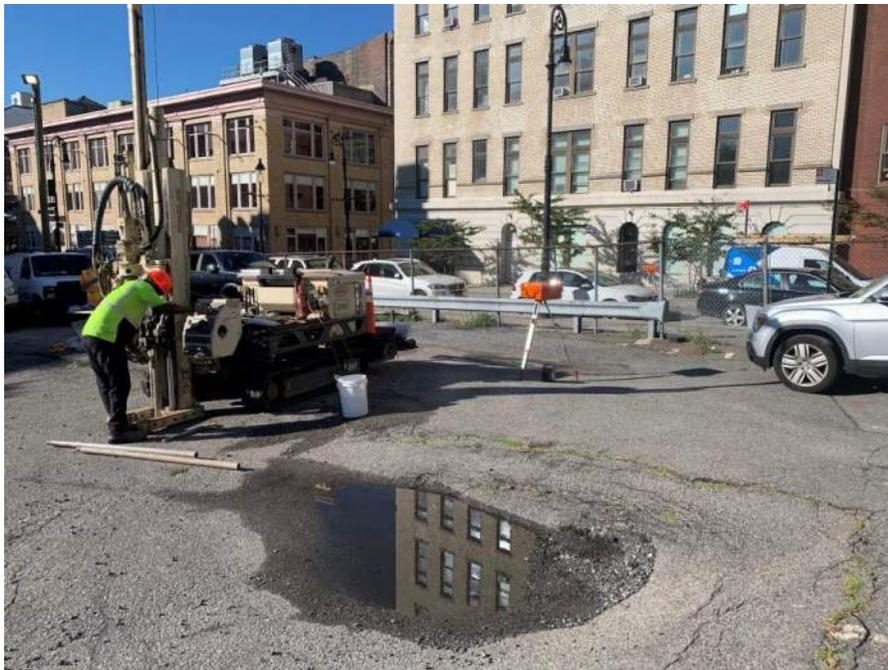
Photo 2: Perimeter CAMP station WZ-1 and off-site CAMP station PM-2 along Beekman Street during the drilling of boring SB37 (facing southwest)
