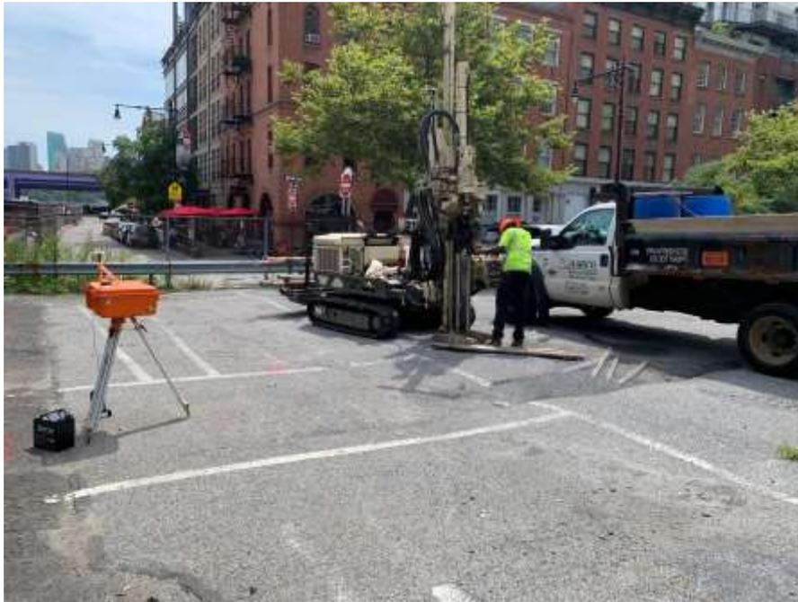
Photo 3: AARCO drilling boring SB32 (facing southeast)
