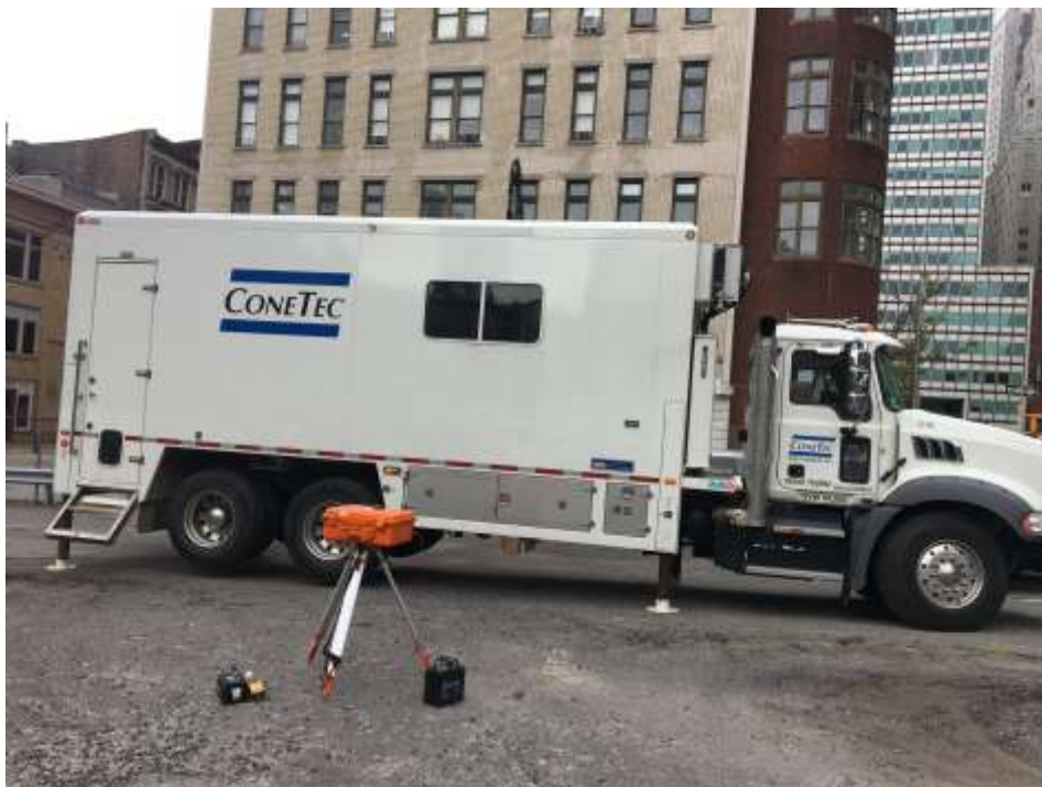
Photo 2: View of ConeTec testing at SCPT-7.
