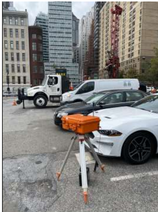
Photo 1: View of Warren George, Inc. predrilling CPT location CPT-17 (facing southwest).
