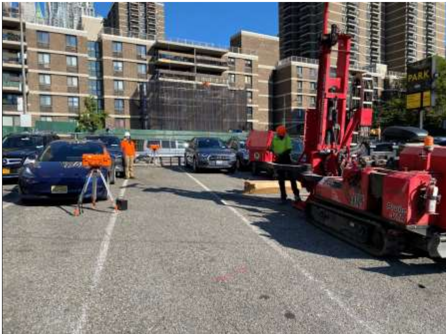
Photo 2: CAMP station WZ-1 and perimeter CAMP station PM-4 along Pearl Street during the drilling of boring SB36 (facing northwest)
