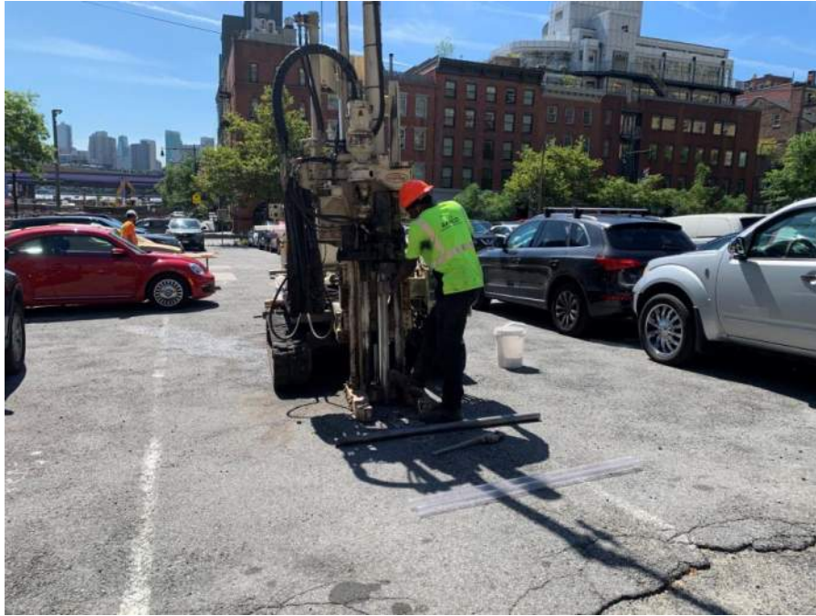
Photo 3: AARCO drilling boring SB30 (facing southeast)
