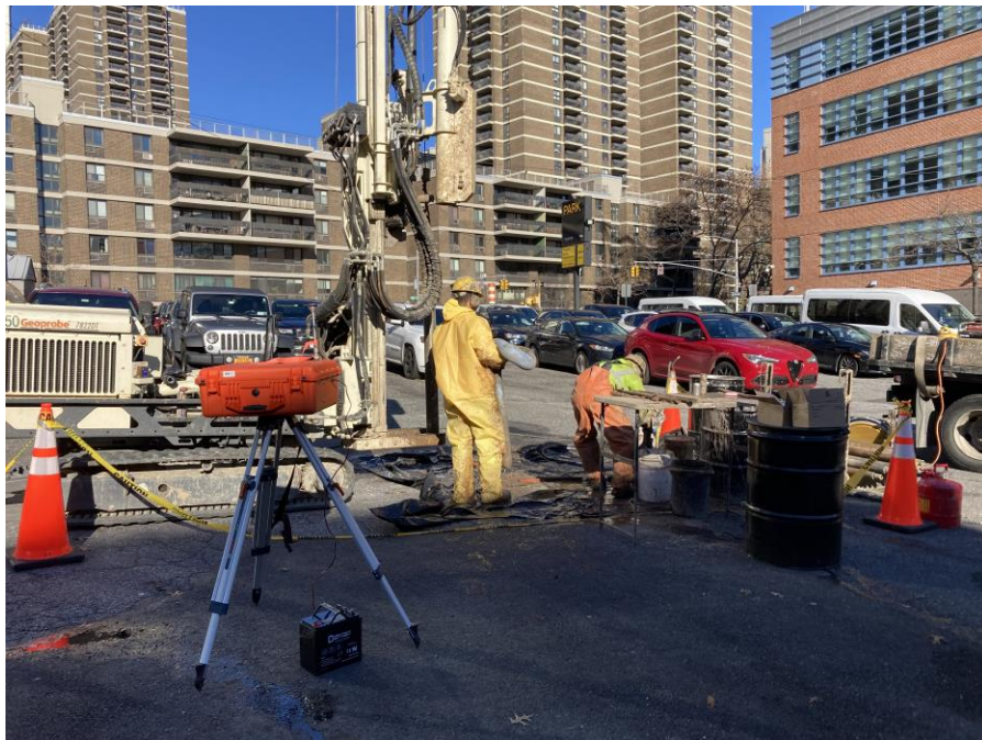
Photo 2: View of AARCO drilling at LB-13 (facing north).
