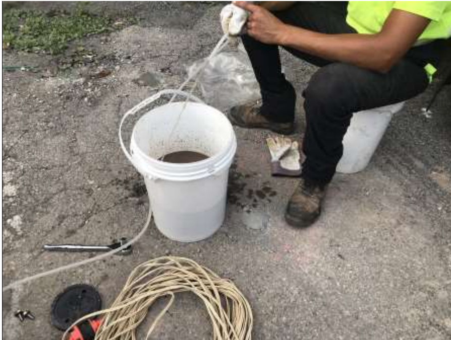
Photo 1: AARCO developing monitoring well MW17 in the southern part of the site (facing south)
