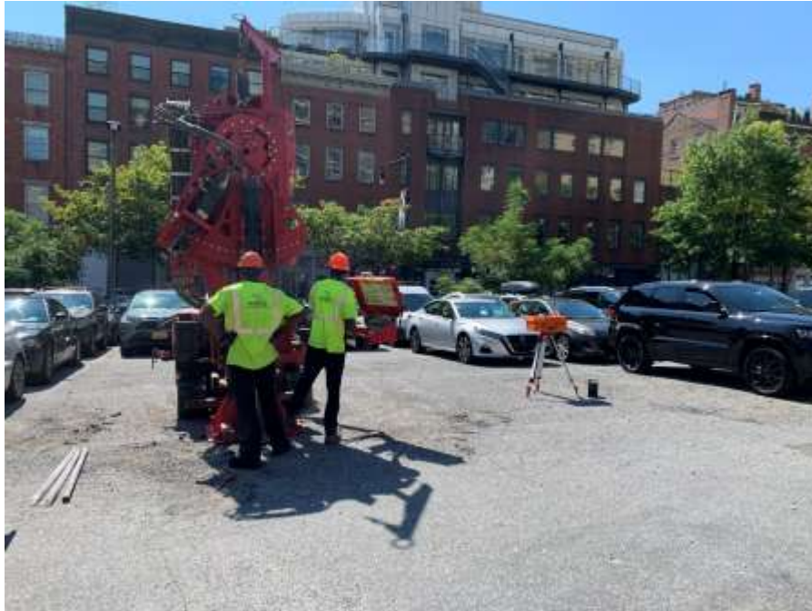
Photo 3: AARCO drilling boring SB26 (facing southeast)
