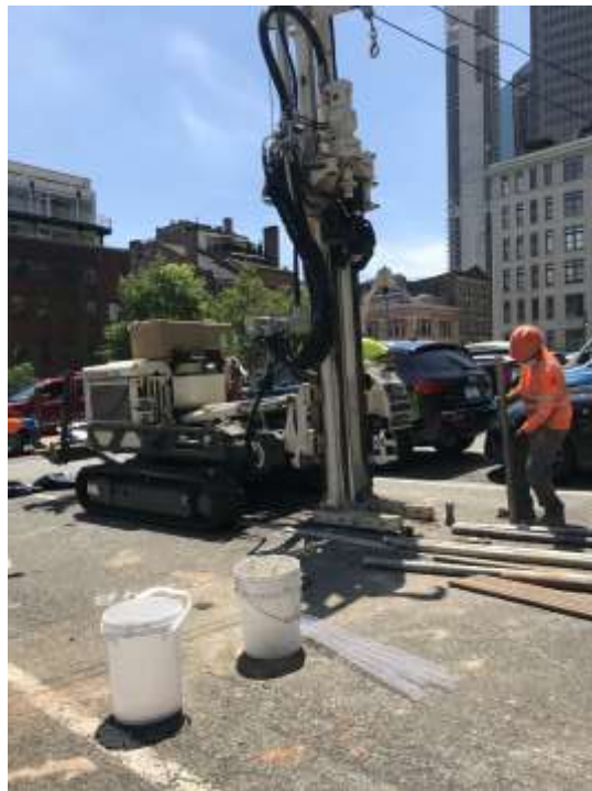
Photo 1: AARCO advancing soil boring SB4W1 (facing southwest)
