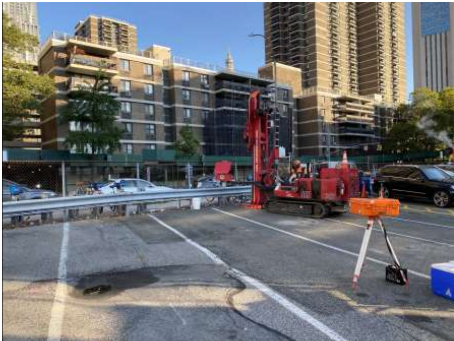
Photo 2: Perimeter CAMP station WZ-1 and off-site CAMP station PM-4 along Pearl Street during the drilling of boring SB4N3 (facing north)
