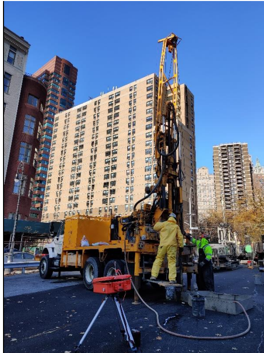
Photo 1: View of AARCO drilling LB-10 (facing northwest).
