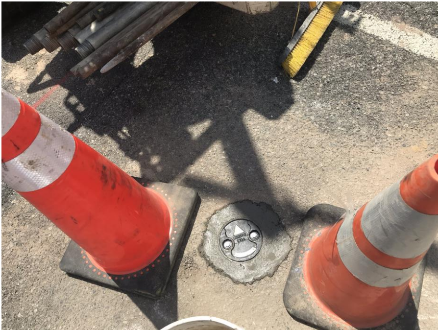
Photo 2: Monitoring well MW25 installed by AARCO
