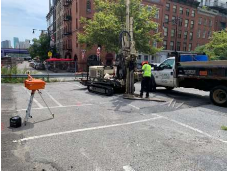
Photo 3: AARCO drilling boring SB32 (facing southeast)
