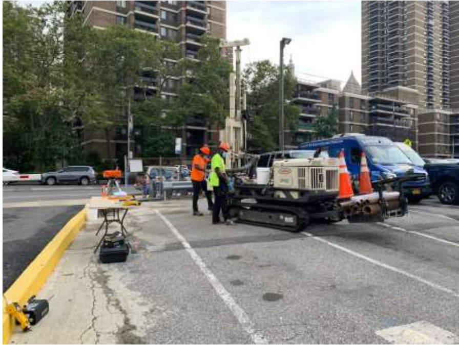
Photo 3: AARCO drilling boring SB15 (facing northwest).
