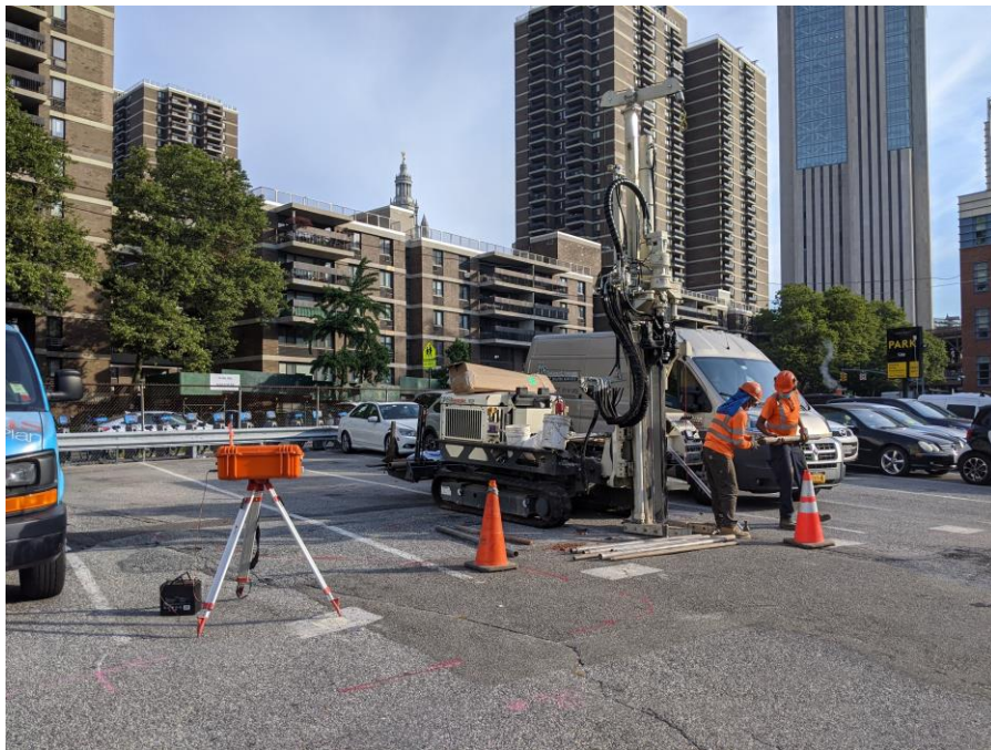
Photo 1: AARCO advancing soil boring SB20 in the northern part of the site (facing north)
