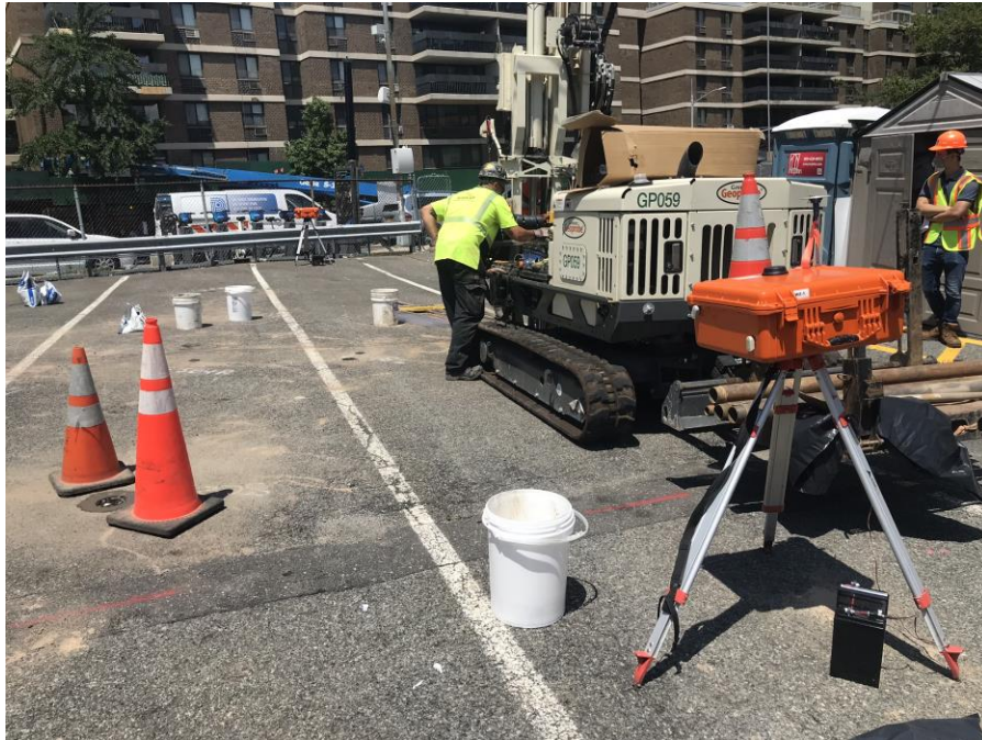
Photo 1: AARCO advancing soil boring SB4E2 in the northern part of the site (facing north)
