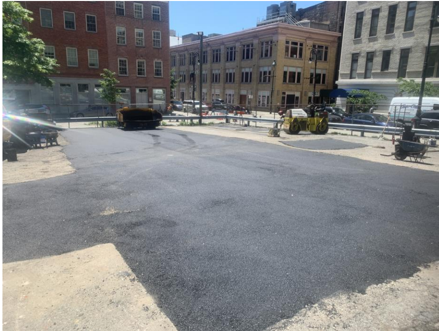
Photo 1: View of the infilled depressed areas near the corner of Water Street and Beekman Street at the end of the day (facing project southwest)
