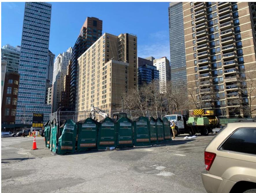
Photo 2: View of typical work zone fencing with chain-link fence and Echo Barrier H9™ acoustic curtains (facing northwest).
