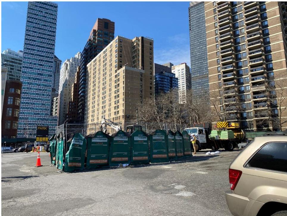
**Photo 2:** Work zone fencing with chain-link fence and Echo Barrier H9™ acoustic curtains (facing northwest) (02/12/2022)
