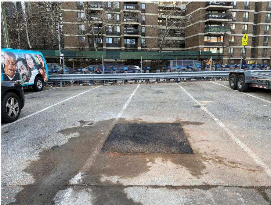
Photo 4: View of test pit TP05, restored to the surrounding grade using cold patch asphalt (facing north).
