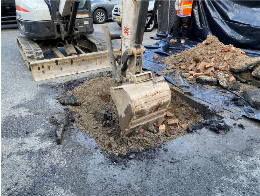
Photo 3: View of AARCO excavating test pit TP03 and stockpiling excavated soil/fill on polyethylene sheeting (facing southeast).
