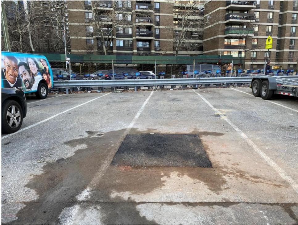
**Photo 15:** View of test pit TP05, restored to match the surrounding grade surface using cold patch asphalt (facing north) (02/12/2022)
