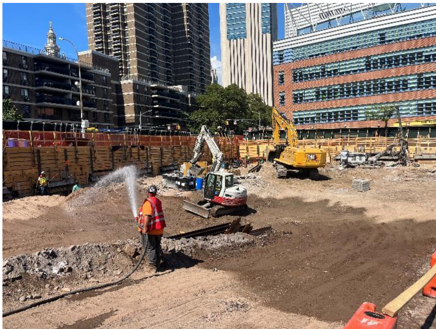
Photo 2: CCJV spraying water to mitigate fugitive dust migration (facing north)
