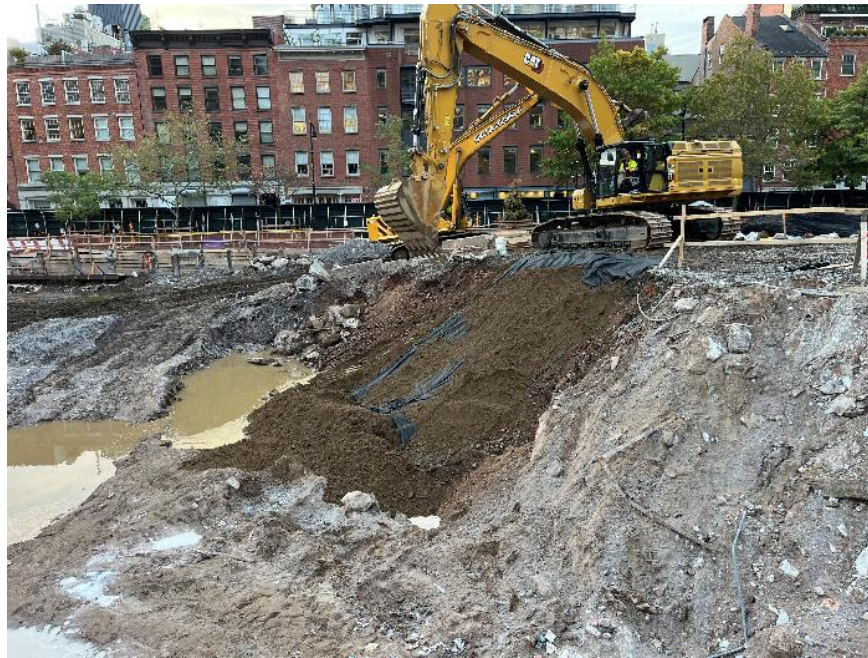
Photo 1: CCJV installing a temporary cover, consisting of imported general fill underlain by geotextile filter fabric, in the northwestern part of the site (facing south)
