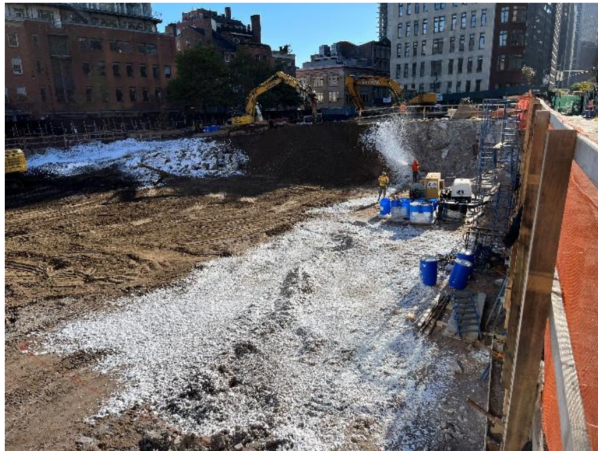
Photo 2: CCJV applying Atmos® AC-645 dust/vapor suppressing foam to exposed soil/fill for the temporary overnight cover (facing southwest)
