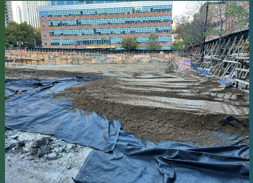
Installation of the Temporary Cover
