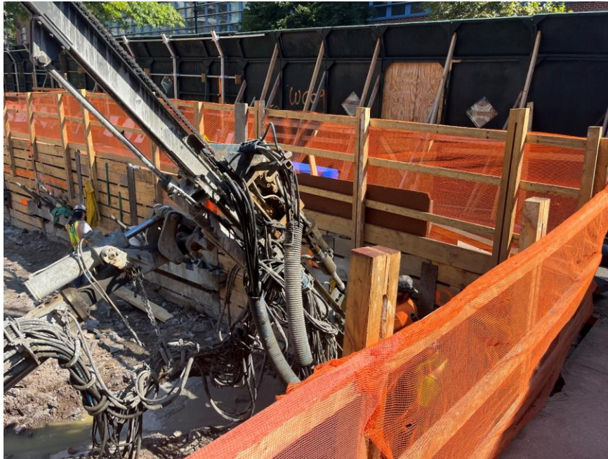
Photo 1: CCJV installing a tieback rod along the eastern boundary of the site (Peck Slip) (facing northeast)
