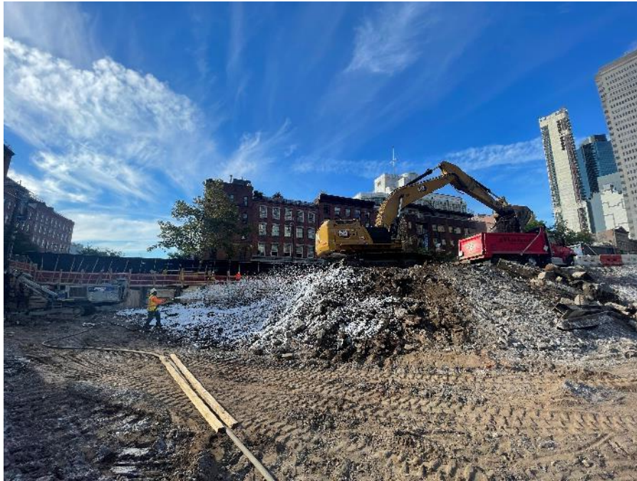
Photo 1: CCJV loading excavated soil/fill for off-site disposal (facing south)
