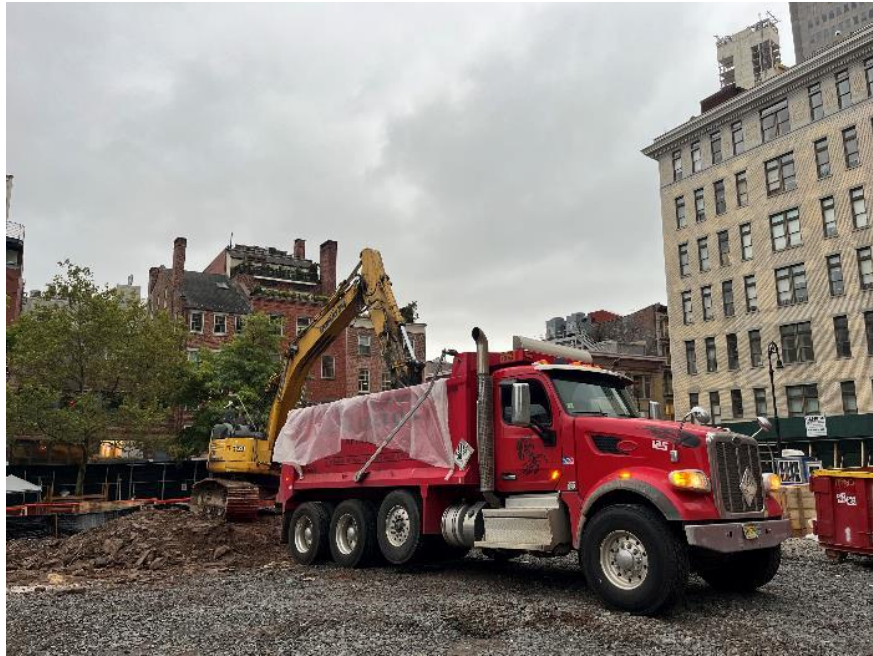
Photo 1: CCJV exporting hazardous lead-impacted soil/fill into tri-axle trucks for off-site disposal (facing southwest)
