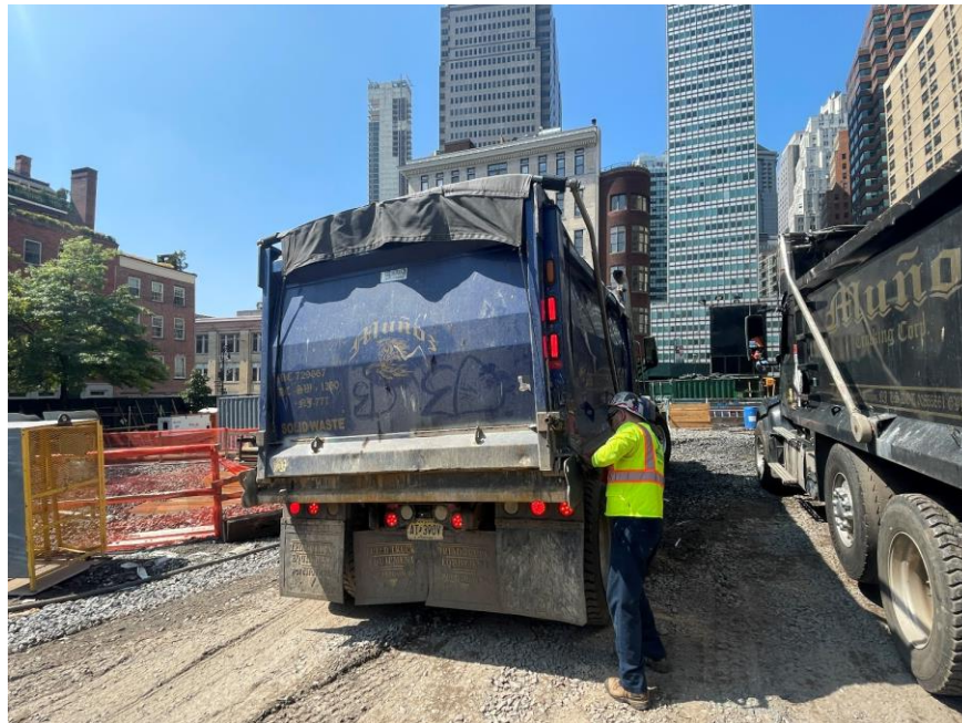
Photo 2: CCJV securing a tight-fitting cover to a loaded dump truck prior to exiting the site (facing west)
