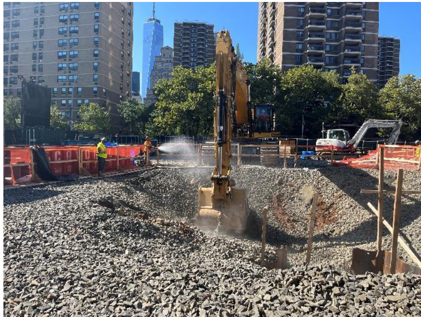
Photo 2: CCJV grading previously backfilled stone to create a staging area for temporary stockpiling of excavated soil/fill (facing north).
