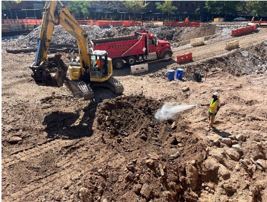
Photo 1: CCJV excavating non-hazardous soil/fill while spraying Mercon-X mercury suppressing foam (facing south)
