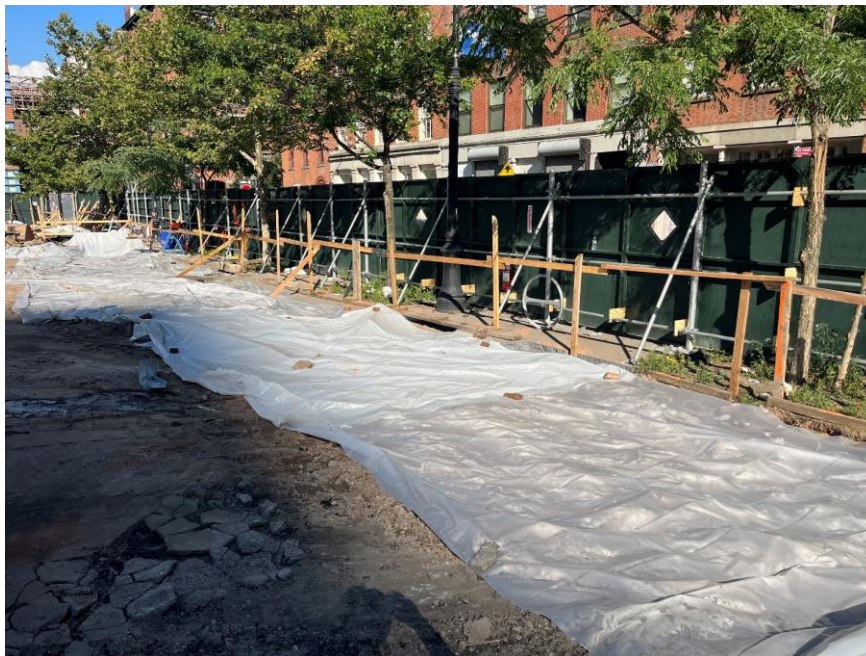
Photo 2: Exposed soil/fill covered with polyethylene sheeting along the southern site boundary (facing southeast)
