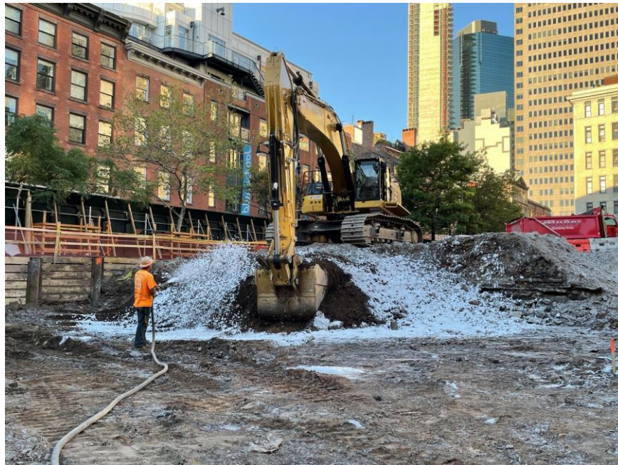
Photo 2: CCJV applying Atmos® AC-645 dust/vapor suppressing foam to exposed soil/fill during excavation in the south-central part of the site (facing southwest).
