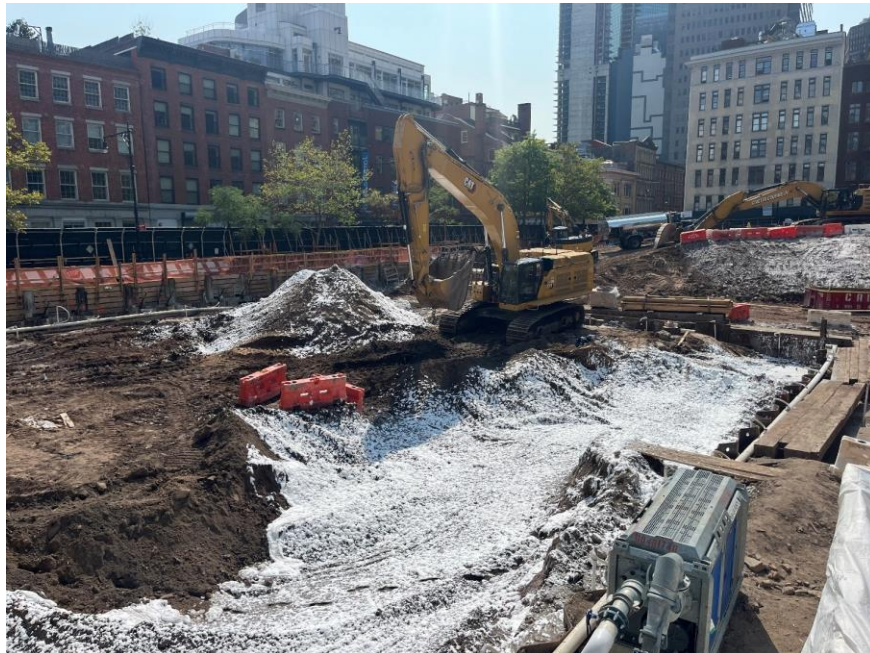
Photo 1: CCJV excavating soil/fill in the southeastern part of the site and actively applying Atmos® AC-645 dust/vapor suppressing foam (facing southwest)
