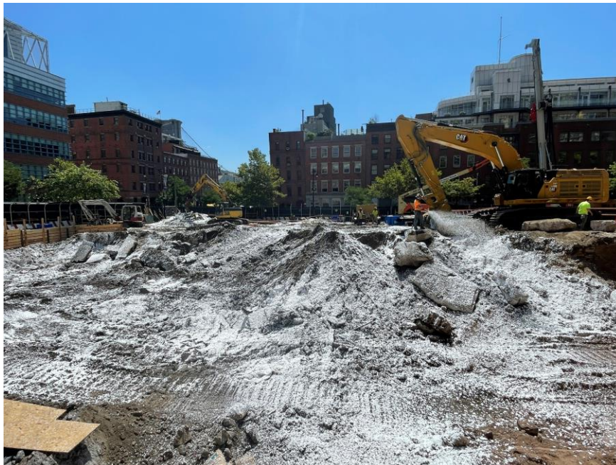
Photo 2: CCJV applying Atmos® AC-645 dust/vapor suppressing foam to exposed soil/fill in the eastern part of the site (facing west)
