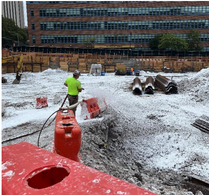
Photo 1: CCJV applying Atmos® AC-645 dust/vapor suppressing foam to exposed soil/fill across the site (facing east)
