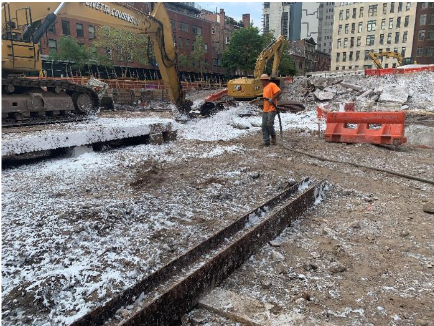
Photo 1: CCJV applying Atmos® AC-645 dust/vapor suppressing foam to exposed soil/fill across the site (facing southwest).
