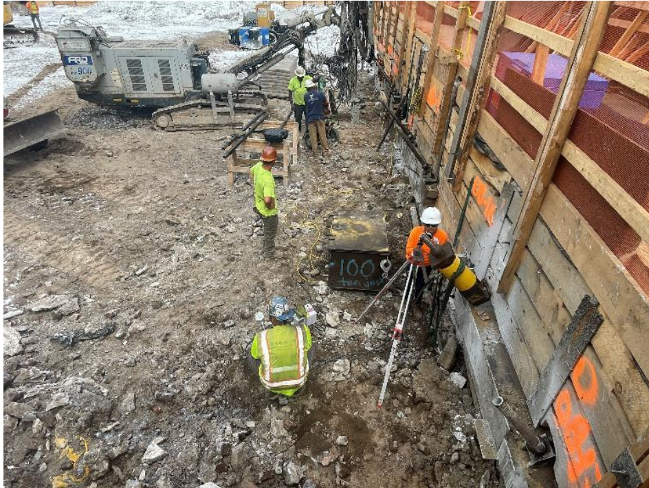
Photo 1: CCJV performing tieback testing along eastern site boundary (facing north)
