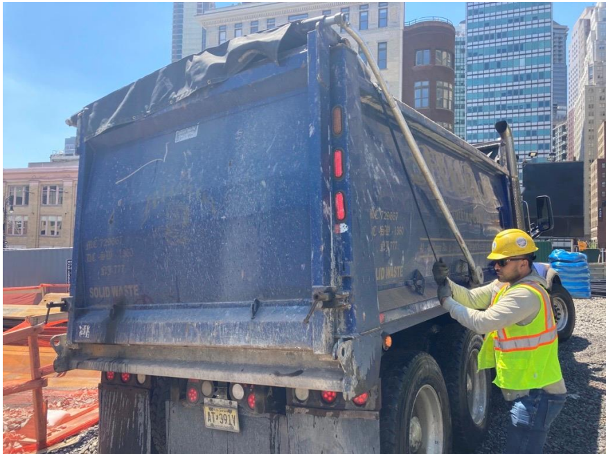
Photo 3: CCJV securing a tight-fitting cover to a loaded dump truck prior to exiting the site (facing west)
