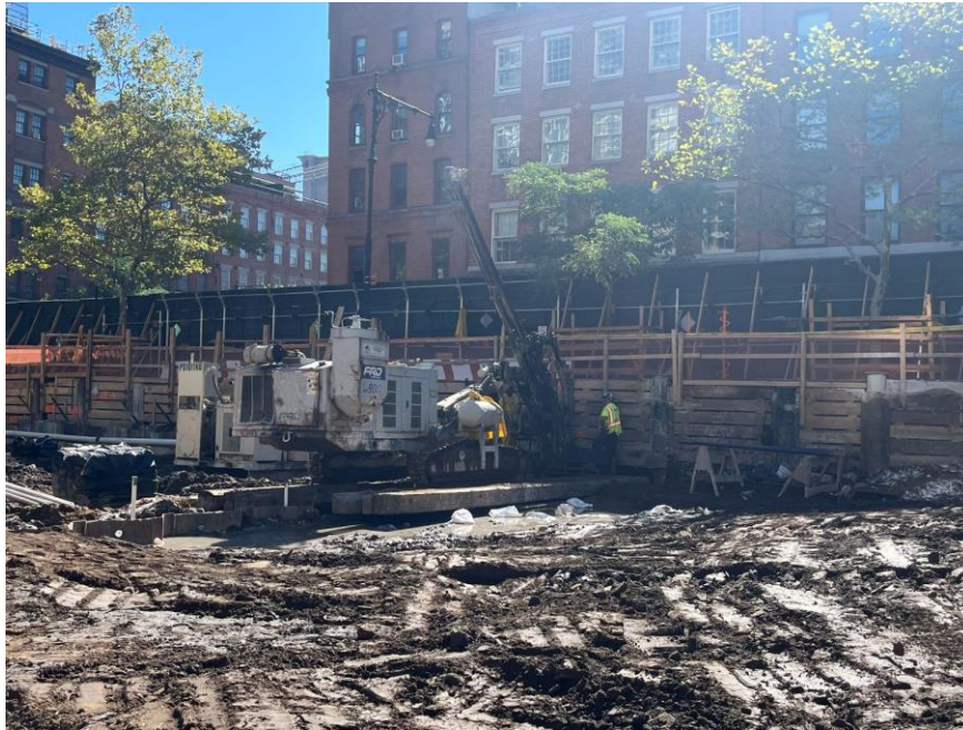
Photo 1: CCJV installing a tie-back along the southern boundary of the site (facing south)
