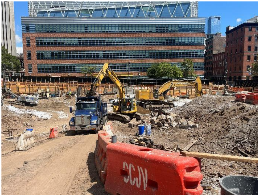
Photo 2: CCJV loading C&D for off-site disposal (facing northeast)
