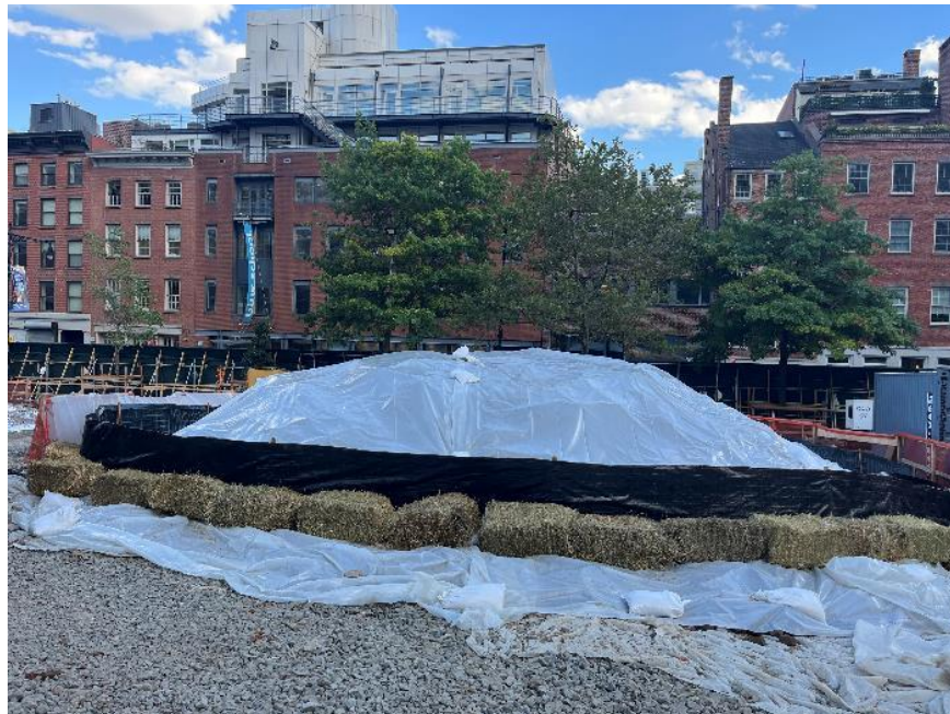
Photo 2: Excavated soil/fill temporarily stockpiled on polyethylene sheeting in the southwestern part of the site (facing south).
