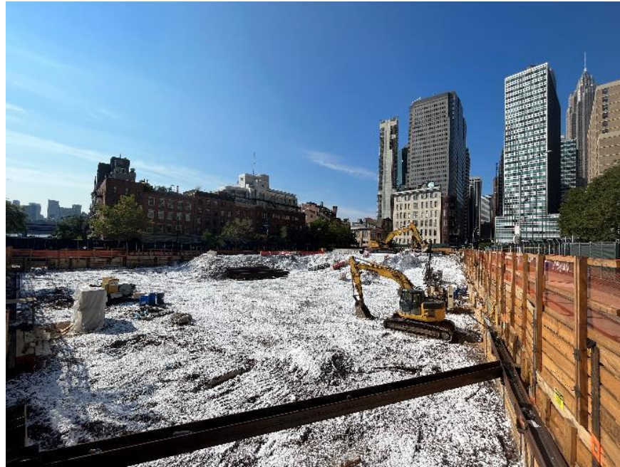
Photo 1: Atmos® AC-645 dust/vapor suppressing foam applied to exposed soil/fill across the site (facing west)
