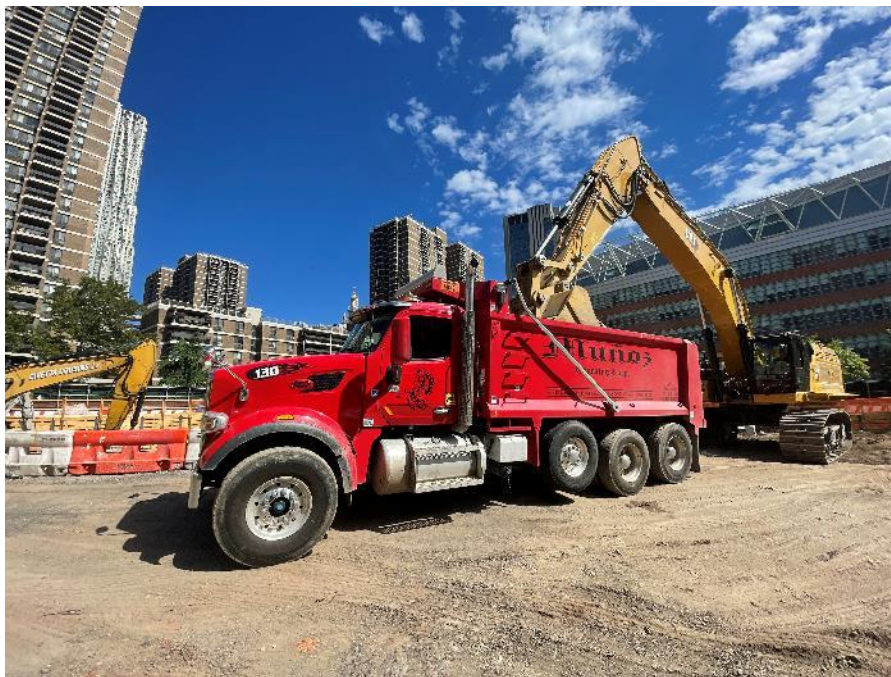
Photo 2: CCJV loading excavated soil/fill for off-site disposal (facing north)
