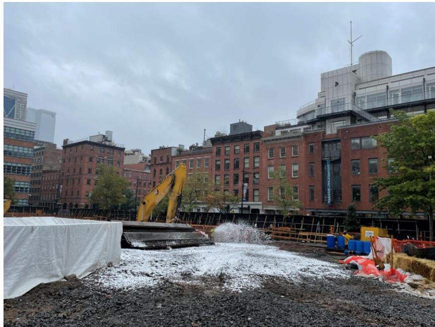
Photo 2: CCJV applying Atmos® AC-645 dust/vapor suppressing foam to exposed soil/fill at the end of the work day (facing southeast).
