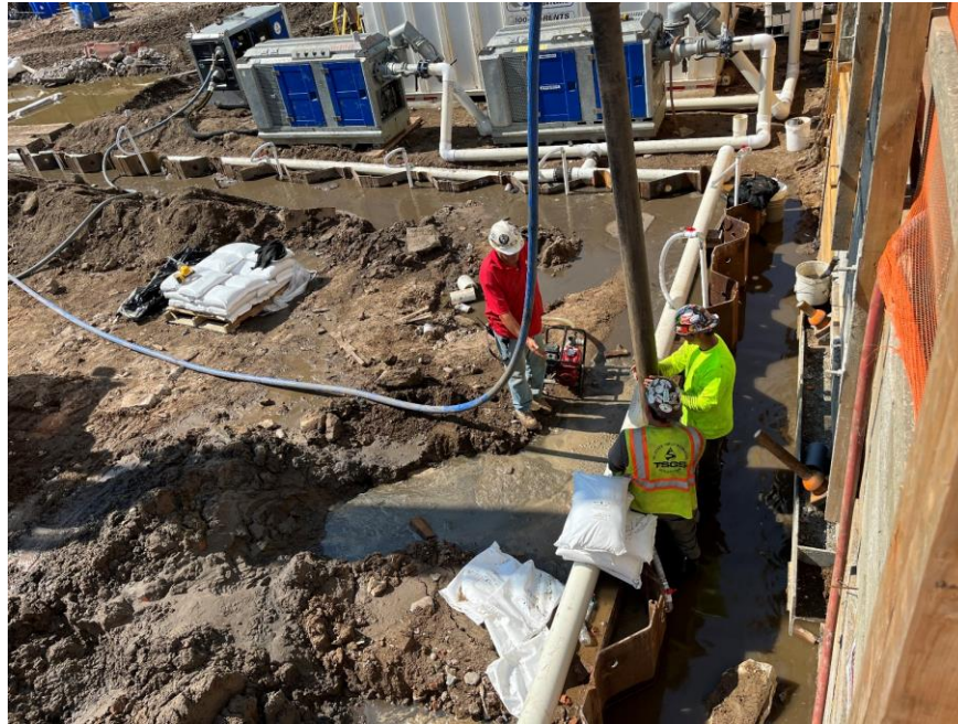
Photo 1: CCJV installing a dewatering well in the southeastern part of the site (facing northwest)
