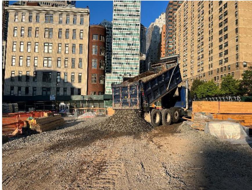
Photo 1: CCJV importing 1.5-inch clean bluestone to the site for tracking pad maintenance (facing west)
