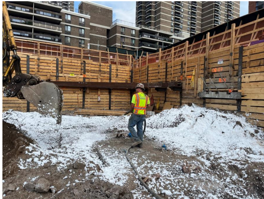
Photo 1: CCJV excavating non-hazardous soil/fill in the northeastern part of the site and actively applying Atmos® AC-645 dust/vapor suppressing foam (facing northeast)
