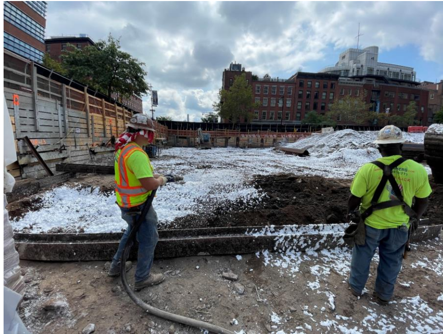
Photo 1: CCJV actively applying Atmos® AC-645 dust/vapor suppressing foam during excavation in the northeastern part of the site (facing south)
