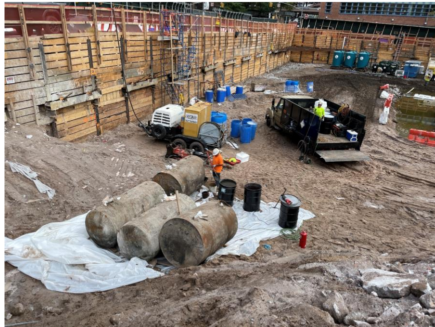
Photo 2: Brookside Environmental cleaning previously removed USTs in preparation for off-site disposal (facing northeast)
