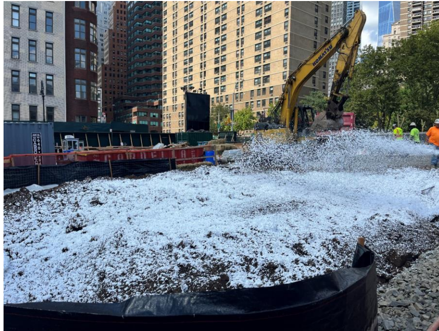
Photo 1: CCJV actively applying Atmos® AC-645 dust/vapor suppressing foam to stockpiled soil/fill during excavation (facing northwest).
