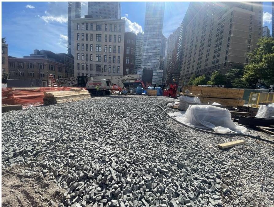
Photo 2: View of tracking pad following import and grading of 1.5-inch stone (facing west)
