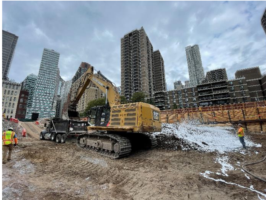
Photo 1: CCJV loading non-hazardous soil/fill into trucks for off-site disposal (facing north)
