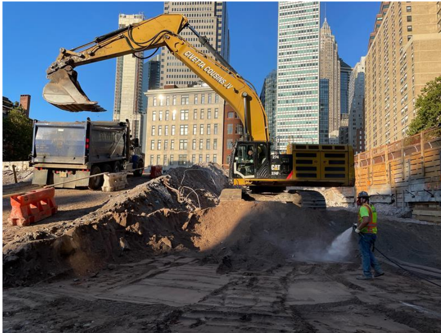
Photo 1: CCJV loading non-hazardous soil/fill into trucks for off-site disposal (facing southwest)
