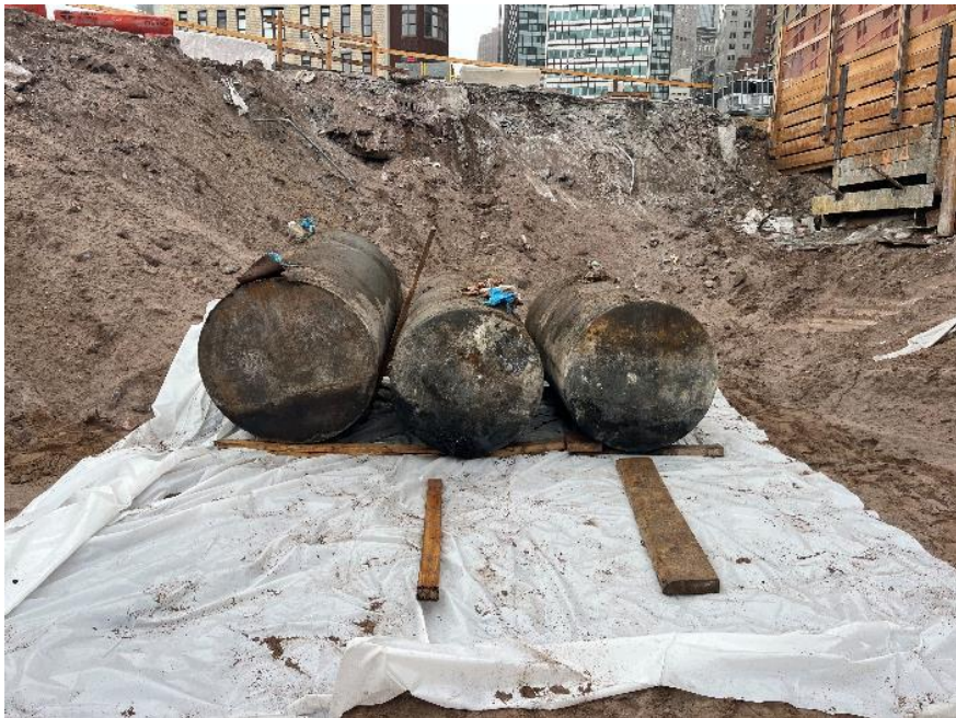
Photo 2: USTs placed on polyethylene sheeting in preparation for additional cleaning and off-site disposal (facing west)
