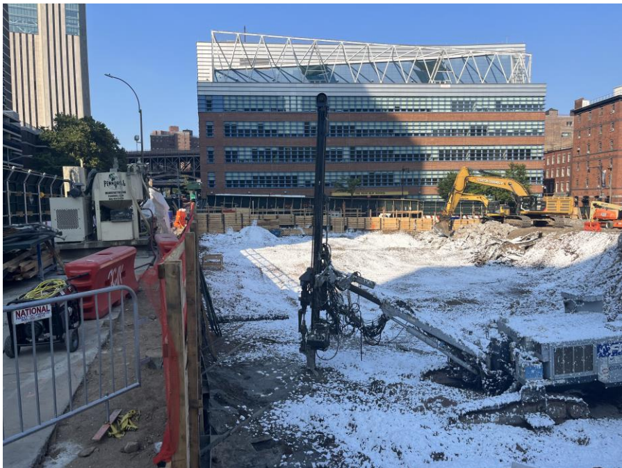
Photo 2: Atmos ® AC-645 dust/vapor suppressing foam applied to exposed soil/fill in the northeastern part of the site (facing east)
