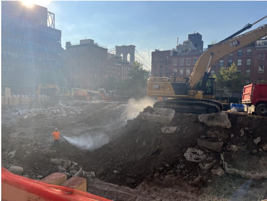
Photo 1: CCJV applying Mercon-X ® during excavation activities in the east-central part of the site (facing southeast)
