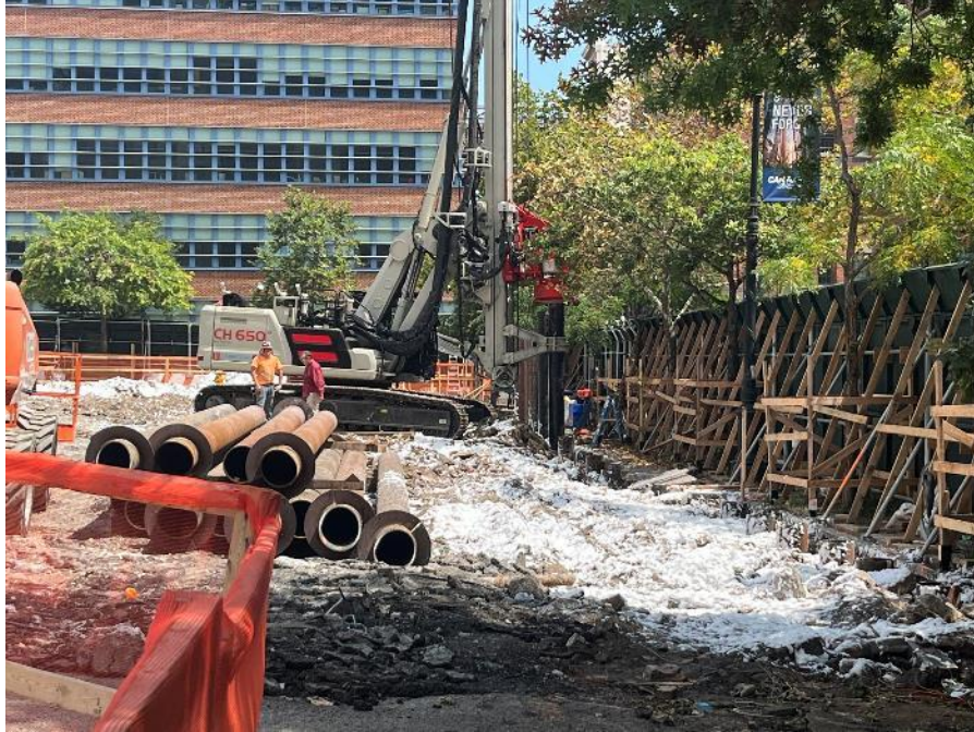
Photo 1: CCJV installing SOE soldier piles along the south perimeter of the site (facing east)
