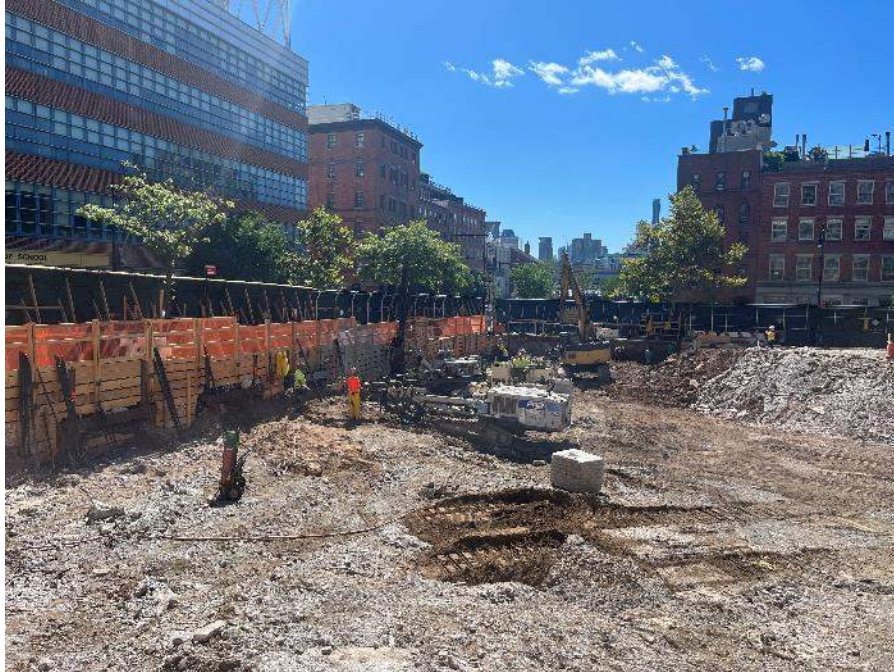
Photo 1: CCJV installing tiebacks for SOE installation along the eastern site boundary (facing southeast).
