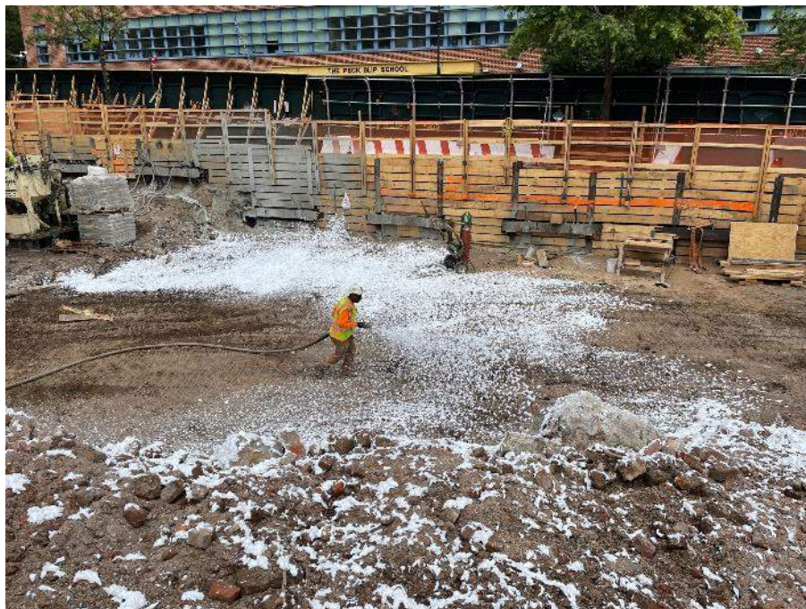
Photo 2: CCJV covering exposed soil with Atmos foam at the end of the day (facing east)
