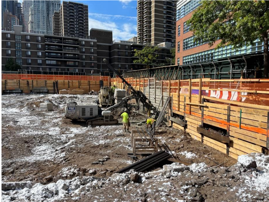
Photo 1: CCJV installing tie-back rods in the eastern site boundary of the site (facing northeast)
