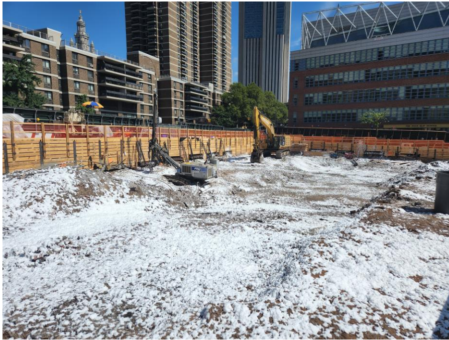
Photo 1: Atmos® AC-645 dust/vapor suppressing foam re-applied to exposed soil/fill in the eastern part of the site (facing northeast)
