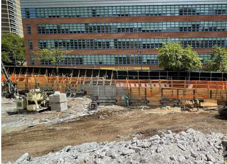
Photo 1: CCJV testing tiebacks and welding braces for SOE installation along the eastern site boundary (facing east).
