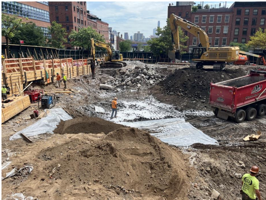
Photo 2: CCJV excavating in the eastern portion of the site (facing southeast)
