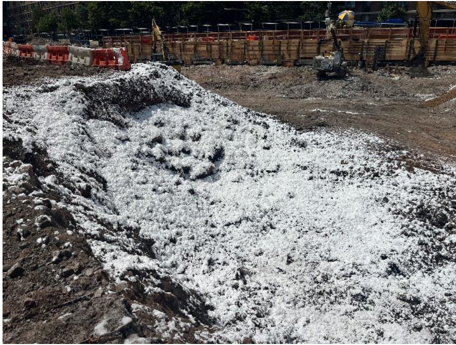
Photo 1: View of ATMOS foam at applied to a petroleum contaminated soil/fill excavation (facing northwest)
