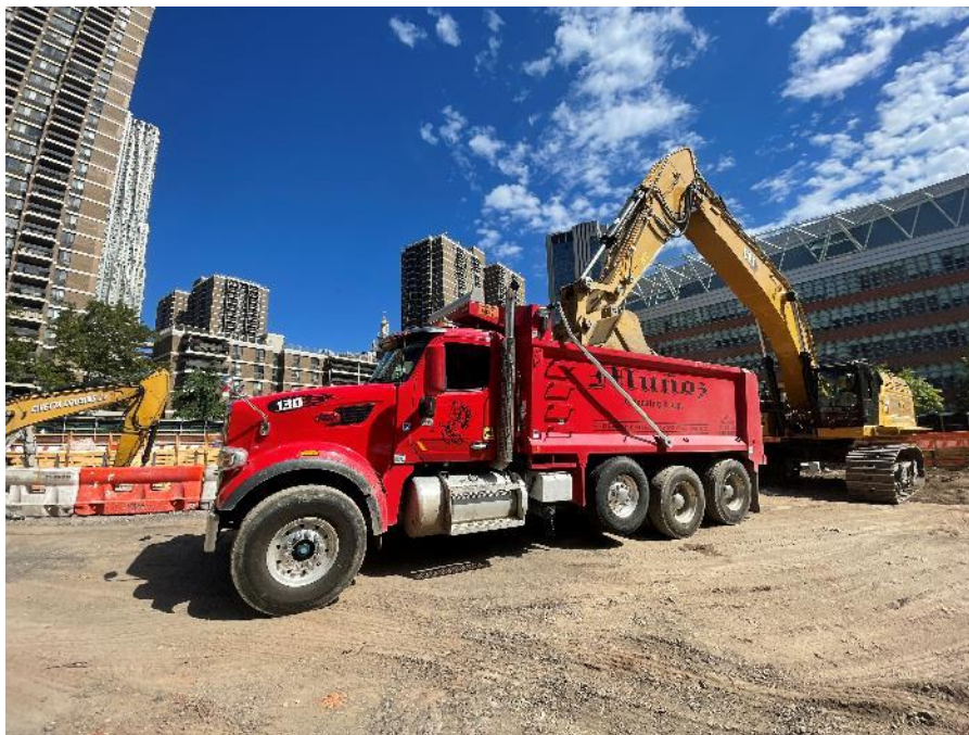
Photo 2: CCJV loading excavated soil/fill for off-site disposal (facing north)
