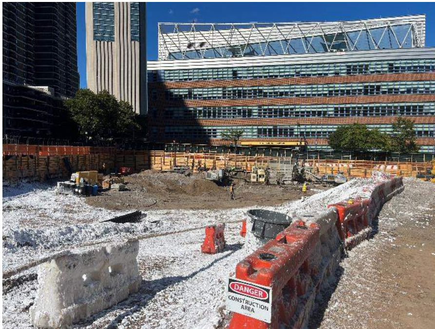
Photo 2: CCJV covering exposed soil with Atmos foam at the end of the day (facing northeast)
