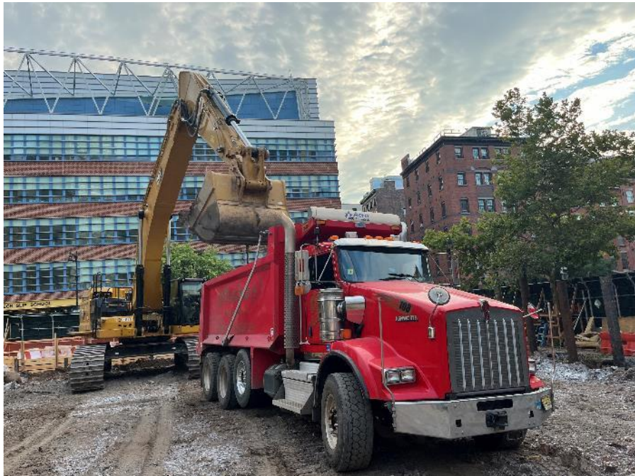
Photo 2: CCJV live-loading petroleum contaminated soil/fill into permitted tri-axial trucks in the southeastern part of the site (facing east)
