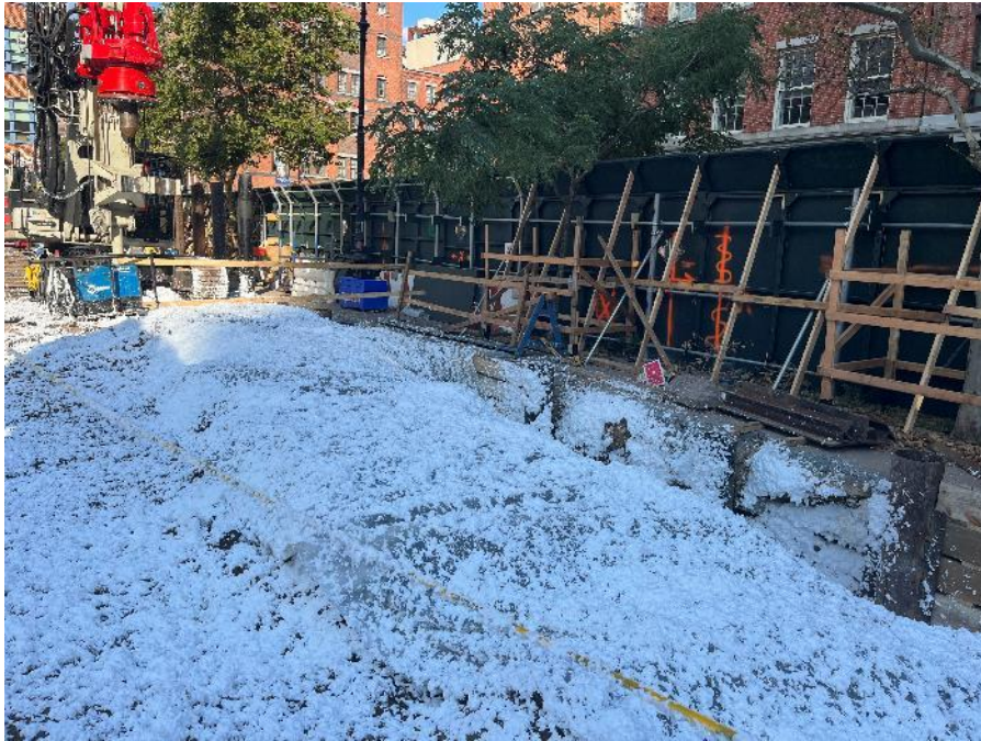
Photo 1: View of Atmos foam on top of polyethylene sheeting applied to previously excavated hazardous-lead soil/fill (facing southeast)
