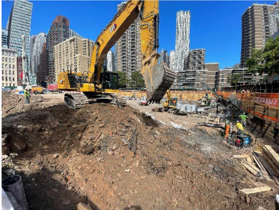
Photo 1: CCJV excavating soil/fill within waste characterization cell WC09 (facing northwest)
