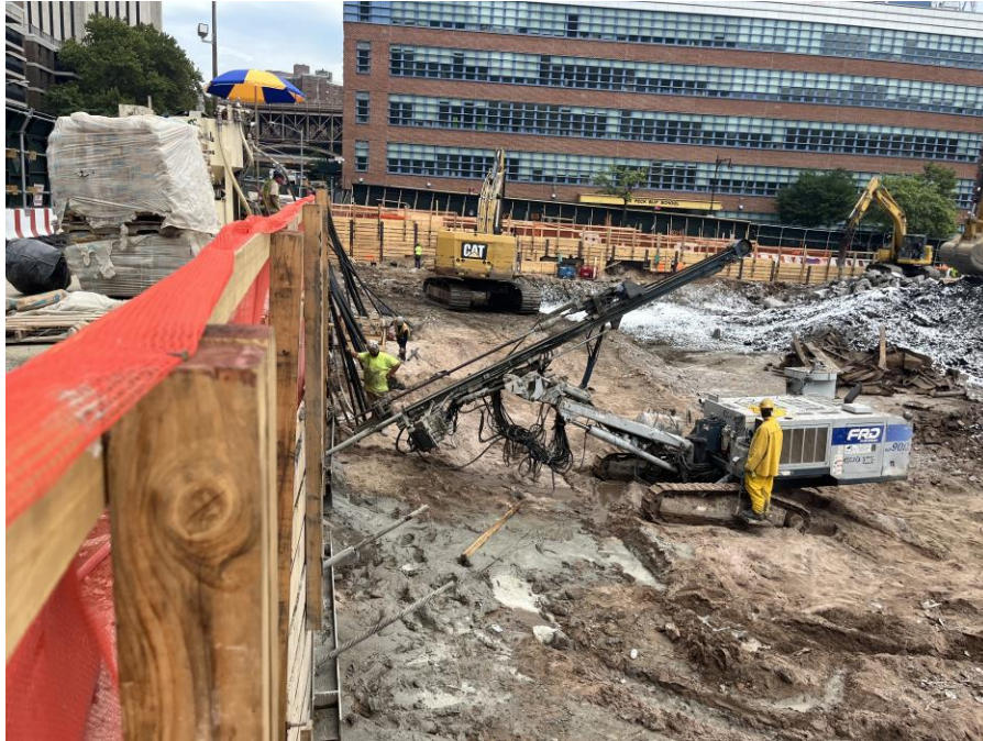
Photo 1: CCJV installing tiebacks along the north perimeter of the site (facing east)
