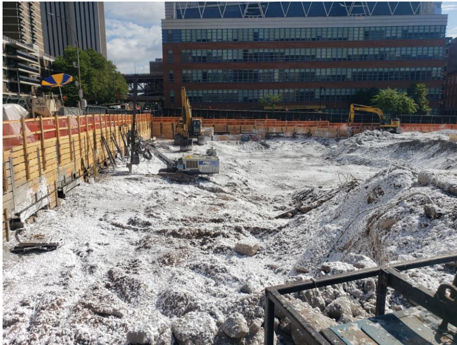
Photo 1: Atmos® AC-645 dust/vapor suppressing foam re-applied to exposed soil/fill in the eastern part of the site (facing north)
