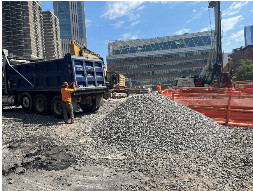
Photo 1: CCJV importing 1.5-inch clean bluestone to extend the truck tracking pad in the northwestern part of the site (facing east)
