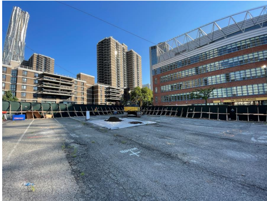
Photo 1: View of CCJV excavating a test pit in the northeastern part of the site and temporarily stockpiling excavated soil/fill on polyethylene sheeting (facing northeast)
