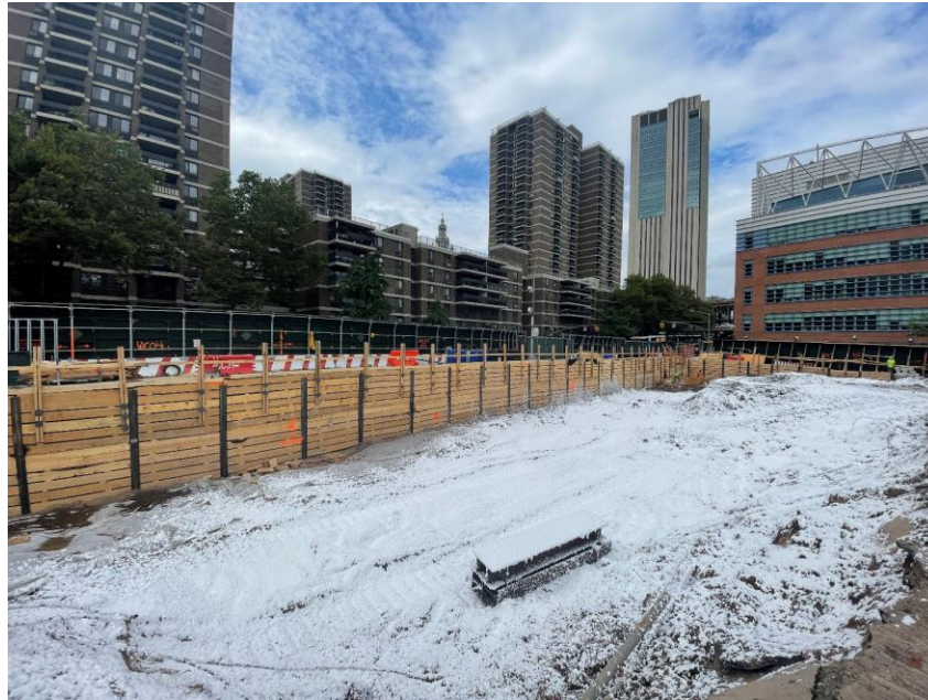
Photo 1: SOE lagging installation progress and Atmos® AC-645 dust/vapor suppressing foam applied to exposed soil/fill in the north-central and northeastern parts of the site (facing northeast)
