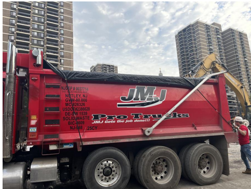
Photo 3: CCJV covering a tri-axle dump truck prior to exiting the site (facing northeast)
