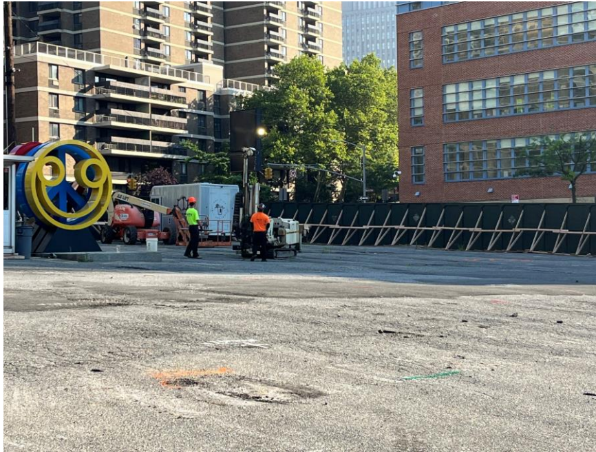
Photo 1: View of Lakewood advancing a soil boring in the northeastern part of the site (facing northeast).
