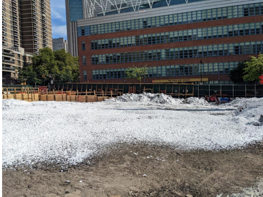
Photo 1: Atmos® AC-645 dust/vapor suppressing foam re-applied to exposed soil/fill in the eastern part of the site (facing east)
