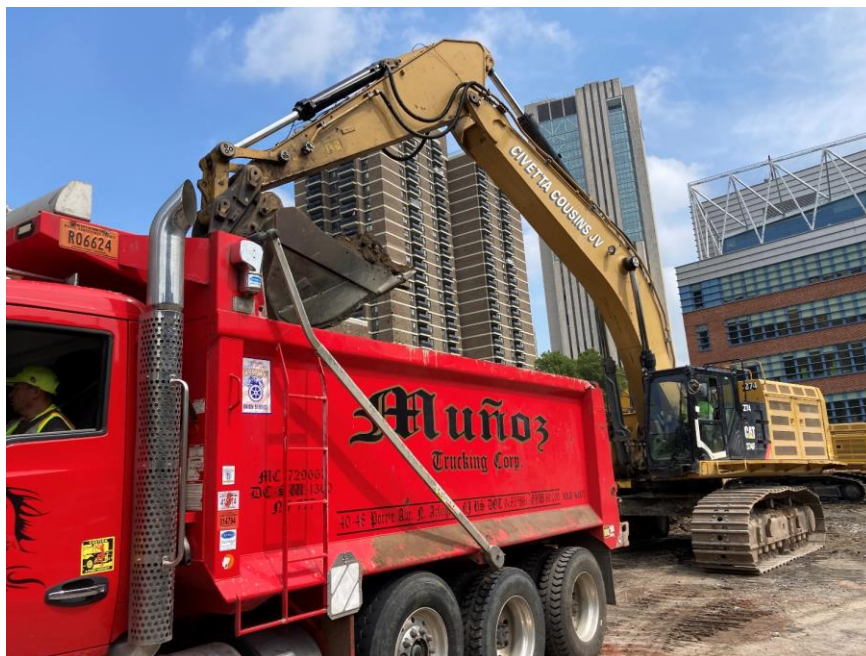
Photo 2: CCJV loading a dump truck with excavated non-hazardous soil/fill for off-site disposal (facing northeast)
