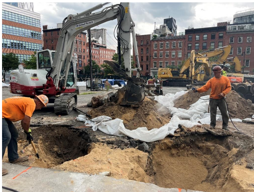
Photo 2: CCJV excavating a test pit along the northern boundary of the site and applying Mercon-X ® to the excavated soil/fill (facing south)
