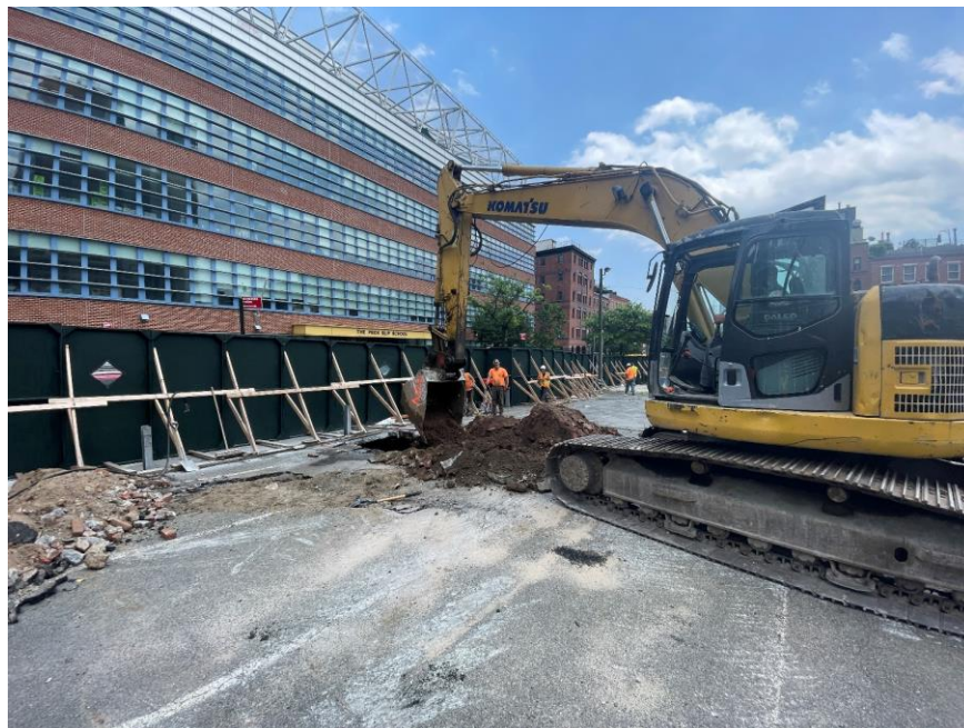
Photo 2: View of CCJV temporarily backfilling a test pit using previously excavated soil/fill (facing southeast).
