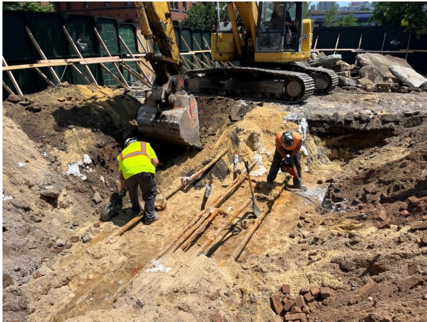
Photo 2: CCJV exposing the concrete-encased USTs and associated piping in the eastern part of the site (facing southeast)
