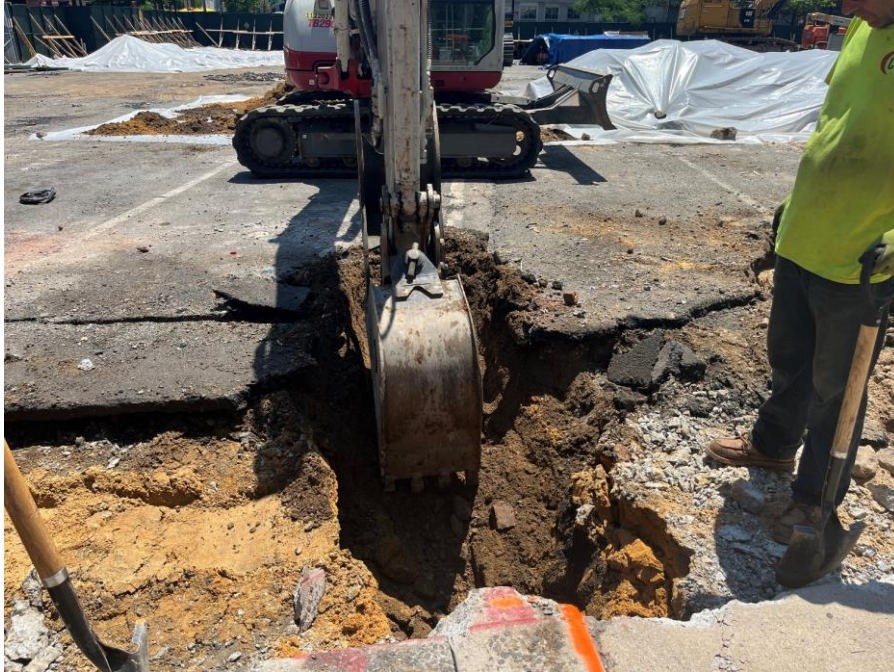
Photo 1: CCJV excavating a test pit along the northern boundary of the site (facing south)
