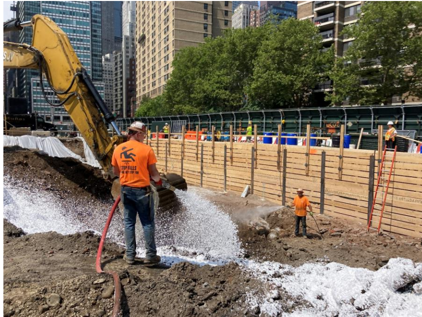
Photo 1: CCJV actively applying Mercon-X® and Atmos® AC-645 dust/vapor suppressing foam to exposed soil/fill during excavation in the north-central part of the site (facing northwest)
