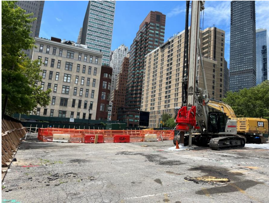
Photo1: General view of the site (facing northwest).
