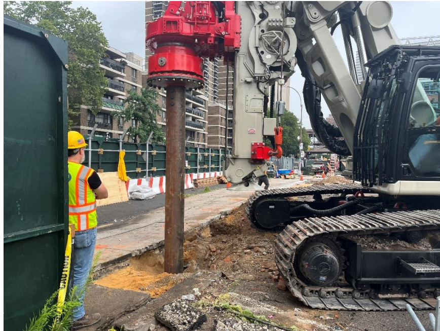
Photo 1: CCJV installing a SOE soldier pile along the northern boundary of the site (facing northeast)
