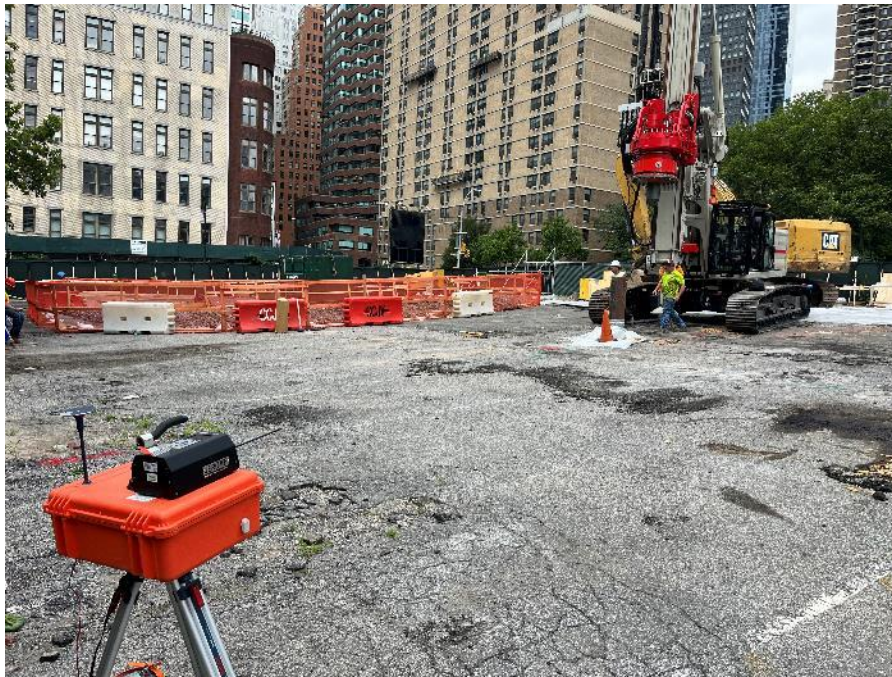
Photo 1: View of CCJV preparing to remove a test displacement soldier pile in the central part of the site (facing northwest).
