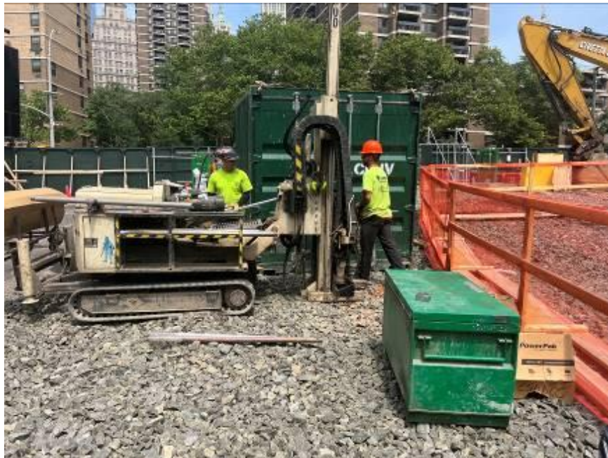
Photo 2: View of Lakewood advancing a soil boring in the west-central part of the site (facing north).
