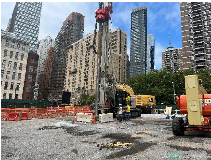
Photo 2: View of CCJV reinstalling a test displacement soldier pile in preparation for support-of-excavation installation (facing northwest).
