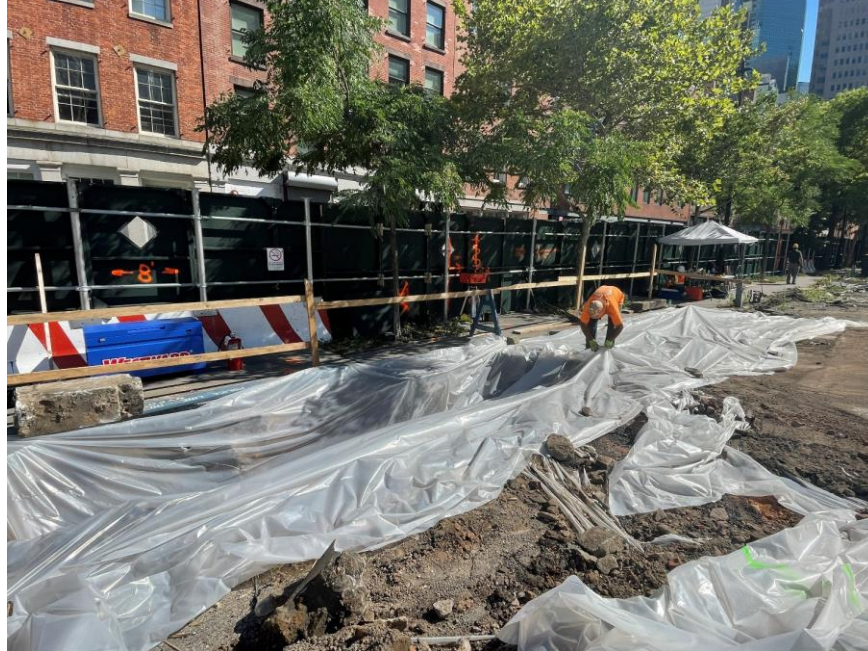
Photo 1: CCJV covering exposed soil/fill with polyethylene sheeting along the southern boundary of the site (facing southwest)
