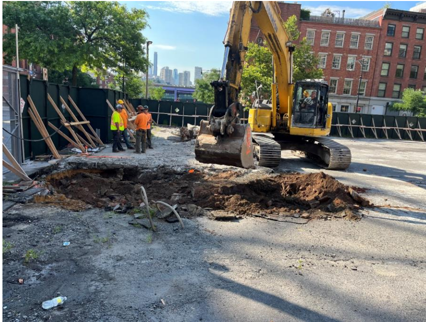
Photo 1: CCJV excavating test pit TP04 in the eastern part of the site (facing south)
