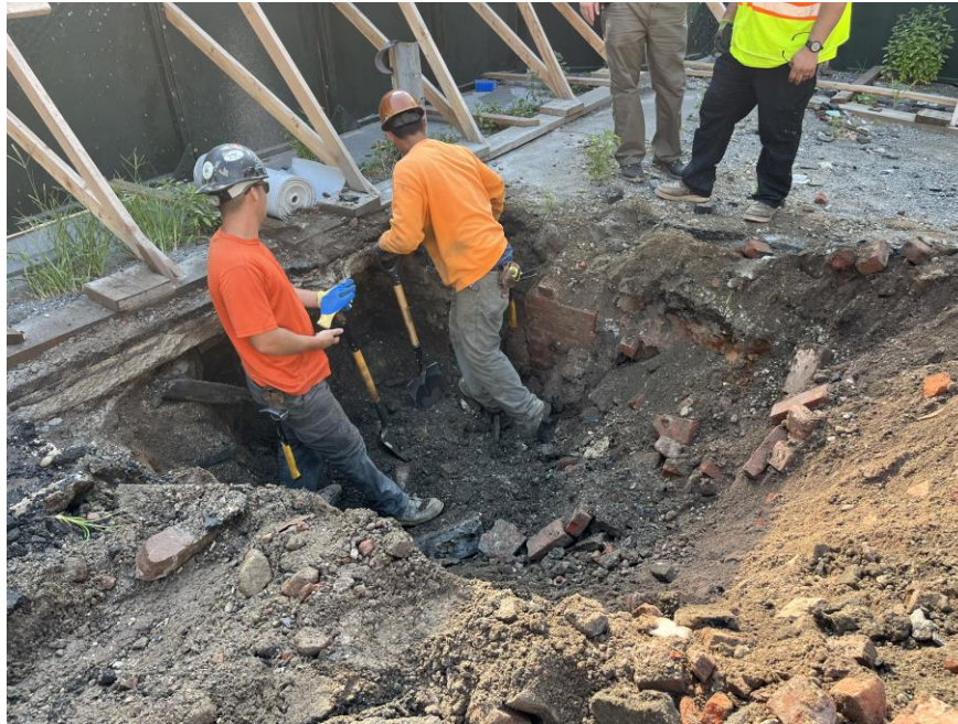
Photo 1: CCJV excavating test pit TP06 in the southeastern part of the site (facing southeast)
