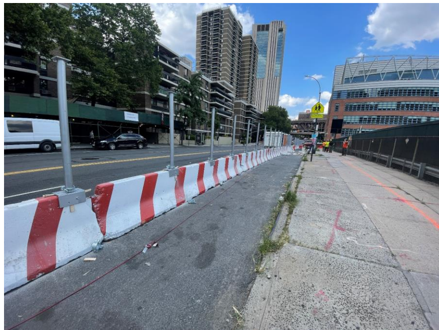
Photo 4: Concrete jersey barriers installed along Pearl Street, immediately north of the site (facing east)
