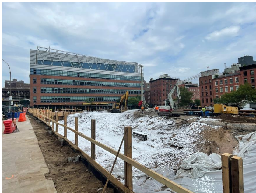
Photo 2: Backfilled general fill behind previously installed timber lagging along the northern site boundary (facing southeast)
