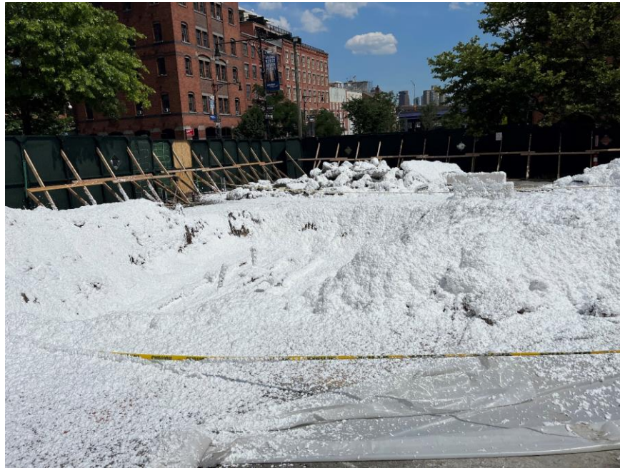
Photo 3: View of exposed soil/fill covered with Atmos® AC-645 dust/vapor suppressing foam at the end of the work day (facing southeast).
