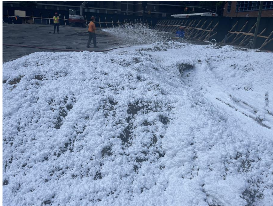
Photo 3: CCJV applying Atmos® AC-645 dust/vapor suppressing foam to areas of exposed soil/fill at the end of the work day (facing north)
