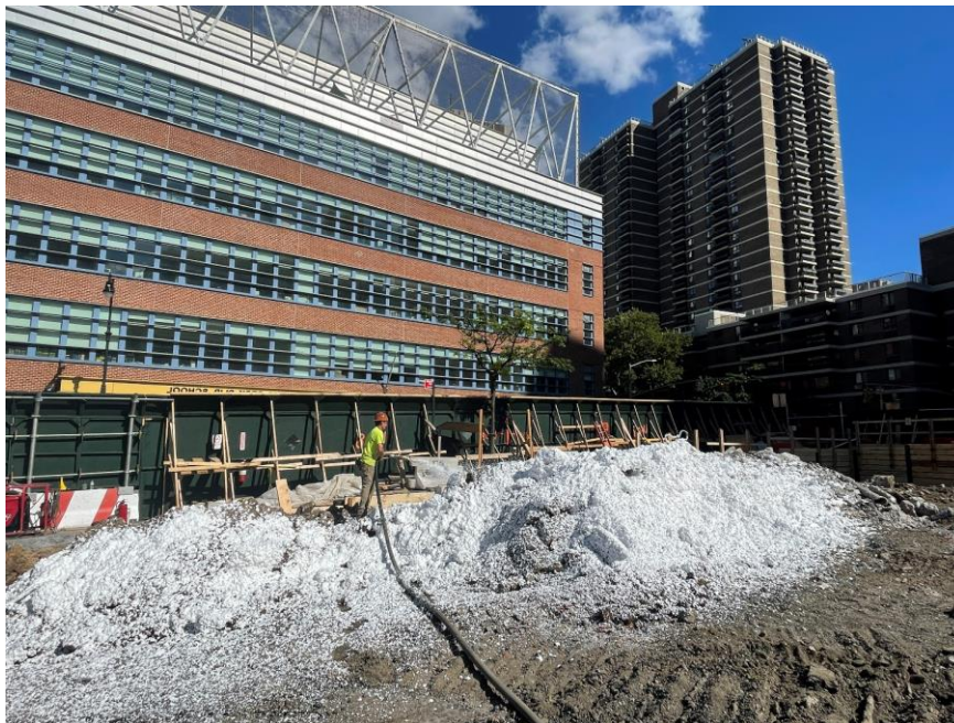
Photo 2: CCJV applying Atmos® AC-645 dust/vapor suppressing foam to exposed soil/fill and stockpiles in the southeastern part of the site (facing southeast)
