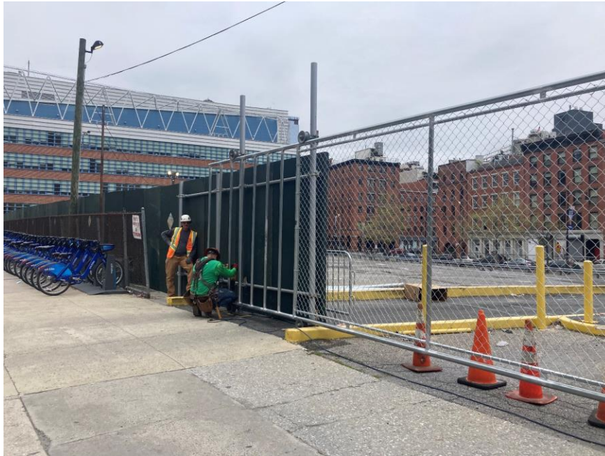
Photo 1: View of perimeter construction fencing installed along the northern boundary of the site (facing southeast).
