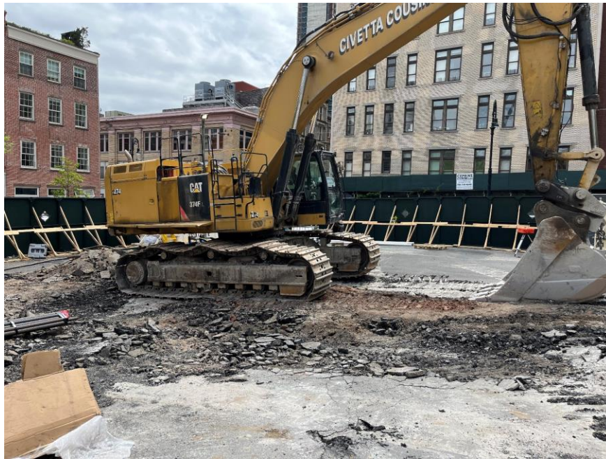
Photo 1: CCJV removing the asphalt cover in the southwestern portion of the site (facing southwest)
