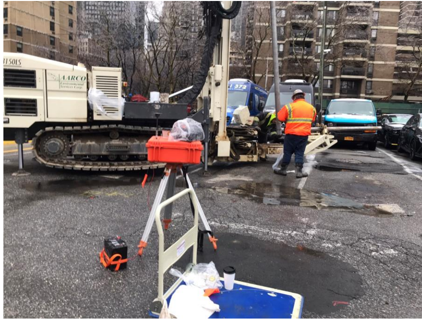
Photo 1: View of AARCO advancing a soil boring in the northwest part of the site (facing north).
