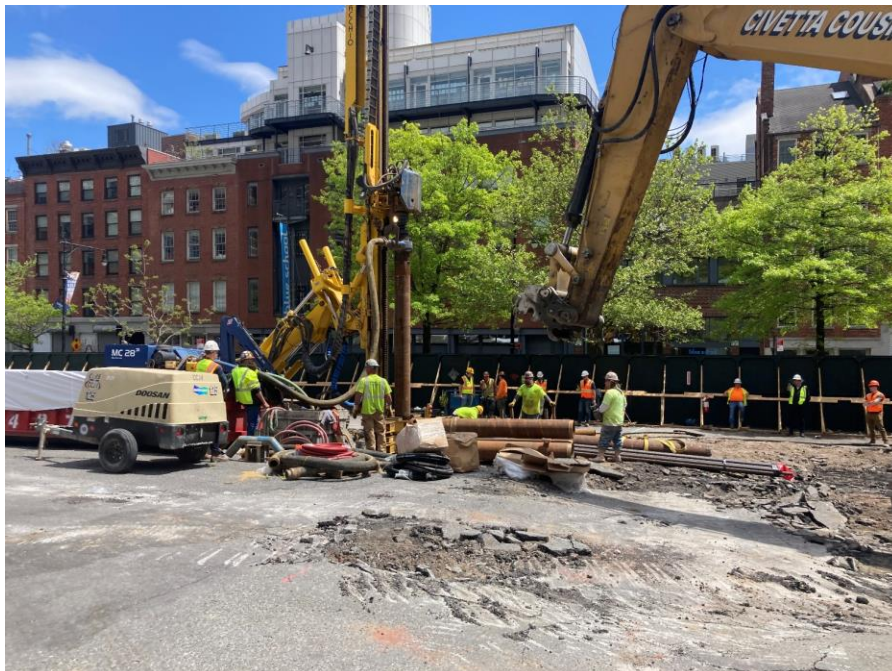
Photo 2: CCJV advancing a pile in the southwestern portion of the site (facing south)
