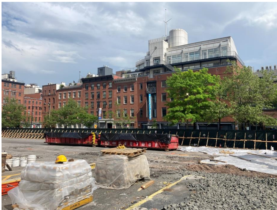
Photo 2: View of covered roll-off containers and polyethylene sheeting atop the excavation area in the southwestern portion of the site (facing southwest).
