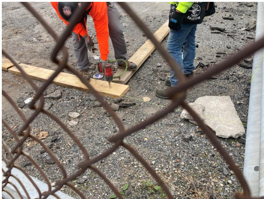
Photo 2: View of UBS drilling 4-inch-long bolts into the ground surface for perimeter construction fencing installation (facing north)
