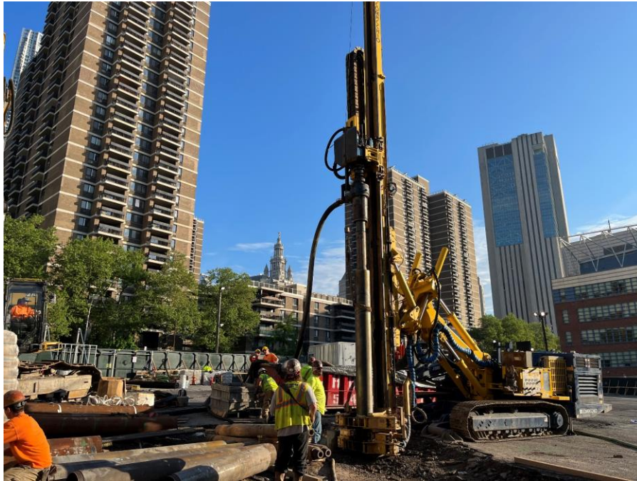
Photo 1: View of CCJV advancing a foundation pile in the southwestern portion of the site (facing northeast).
