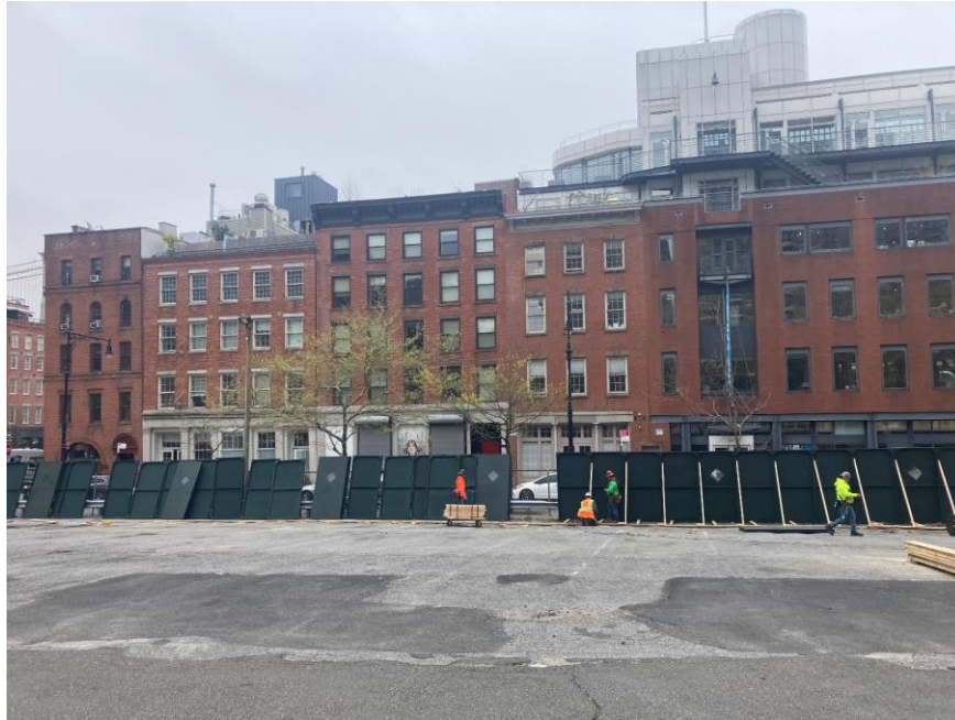
Photo 1: View of perimeter construction fencing being installed along the southern boundary of the site (facing south).
