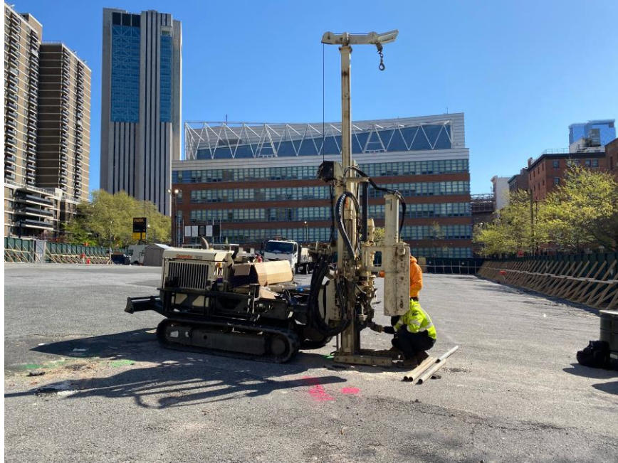
Photo 1: View of AARCO advancing a delineation soil boring in the southwestern portion of the site (facing east).
