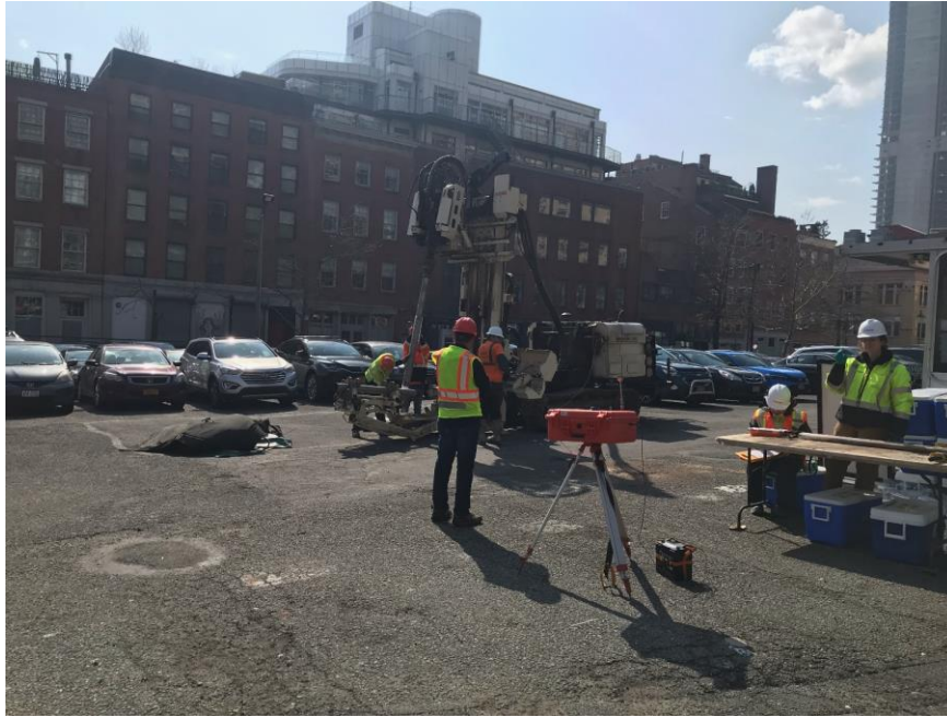
Photo 1: View of AARCO advancing a soil boring in the central part of the site (facing southwest).
