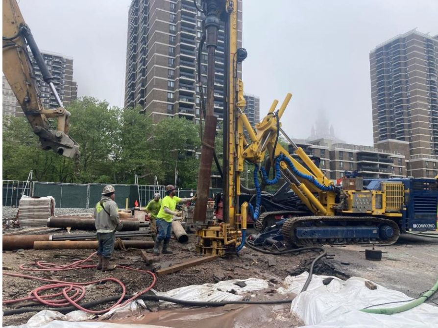
Photo 1: View of CCJV advancing a foundation pile in the southwestern portion of the site (facing southwest)
