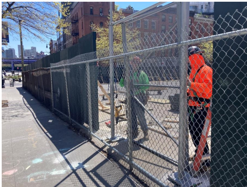
Photo 2: View of perimeter fencing installation along Peck Slip (facing southwest).
