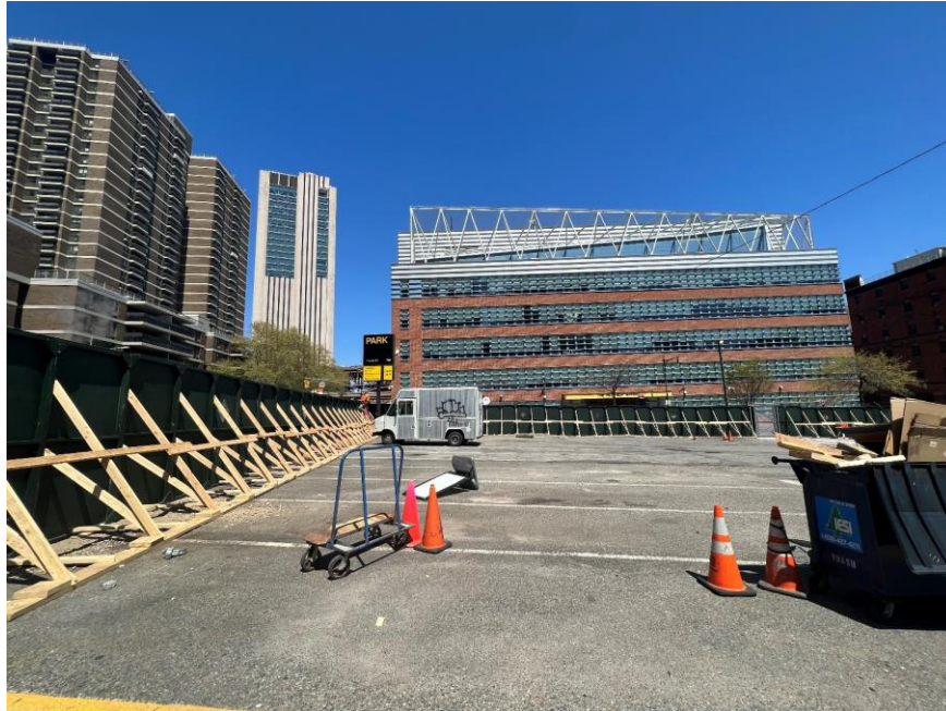
Photo 1: View of the perimeter construction fence installed along Pearl Street and Peck Slip (facing east).
