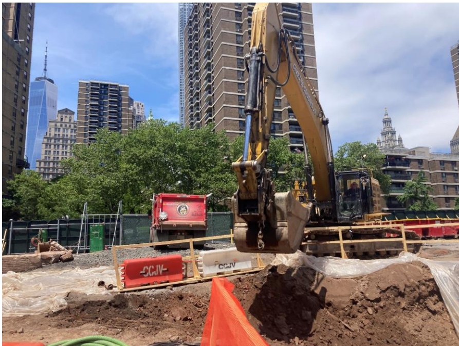
Photo 2: View of CCJV excavating hazardous lead-impacted soil/fill along the northern berm of the work area in the southwestern portion of the site (facing north)
