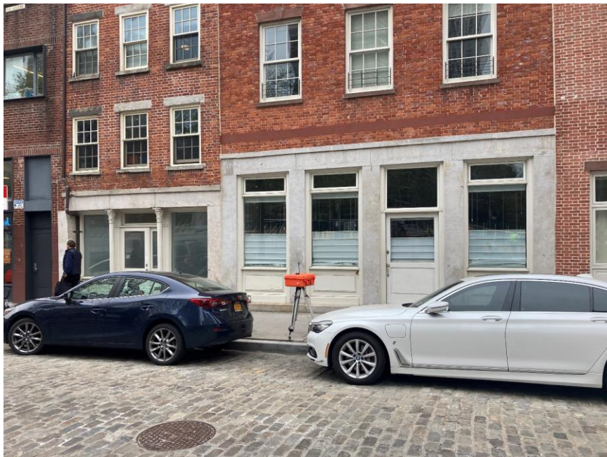
Photo 2: View of perimeter CAMP station PM-3, relocated to the southern sidewalk of Water Street (facing south)
