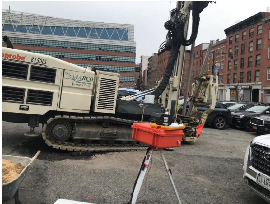
Photo 1: View of AARCO advancing a soil boring in the southeast part of the site (facing south).
