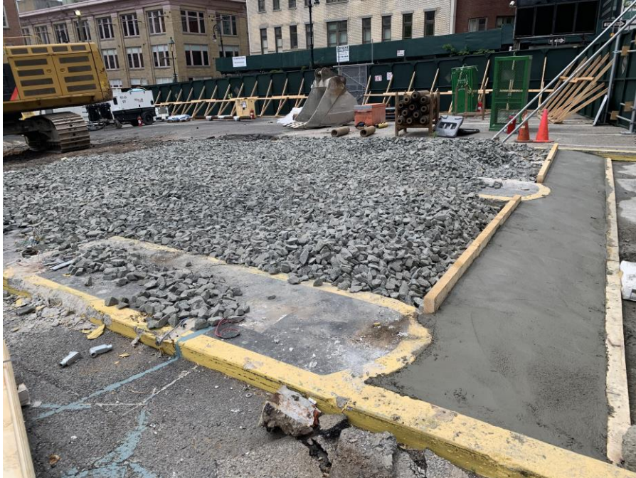
Photo 1: View of concrete placed along the northern edge of the tracking pad (facing southwest).
