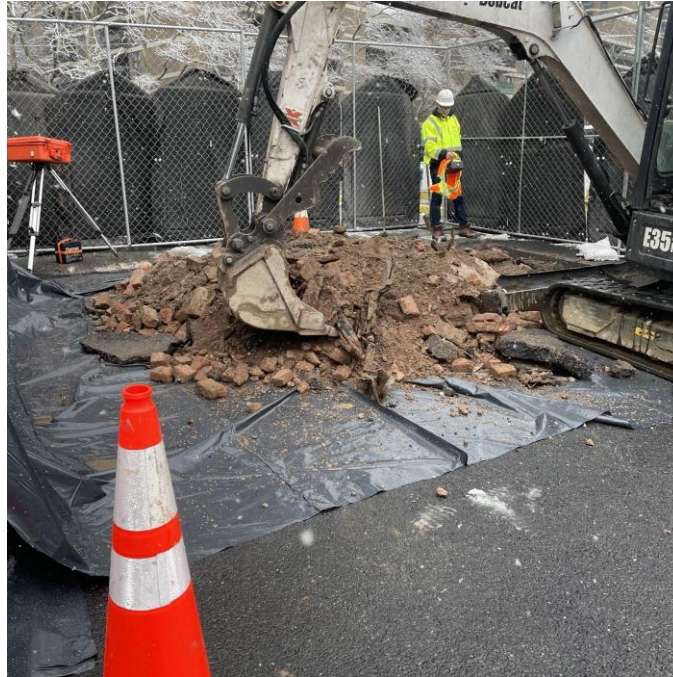
Photo 3: View of Jerome® J505 screening during backfilling of Test Pit TP04 (facing north)
