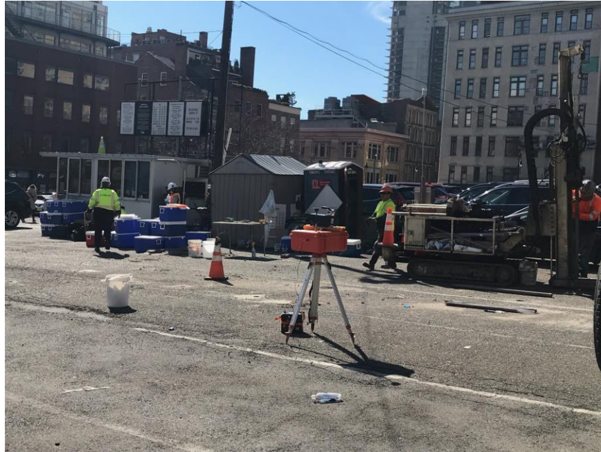
Photo 3: View of work zone air monitoring station WZ-1, placed downwind of drilling activities (facing southwest).
