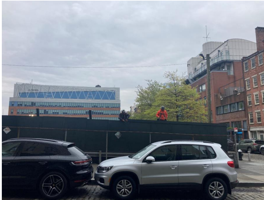
Photo 1: UBS installing wooden trim to the construction fence along Beekman Street (facing east).
