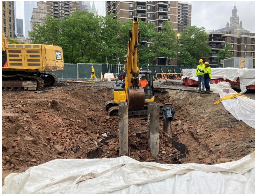
Photo 1: View of CCJV excavating hazardous lead-impacted soil/fill between previously installed foundation piles (facing north)
