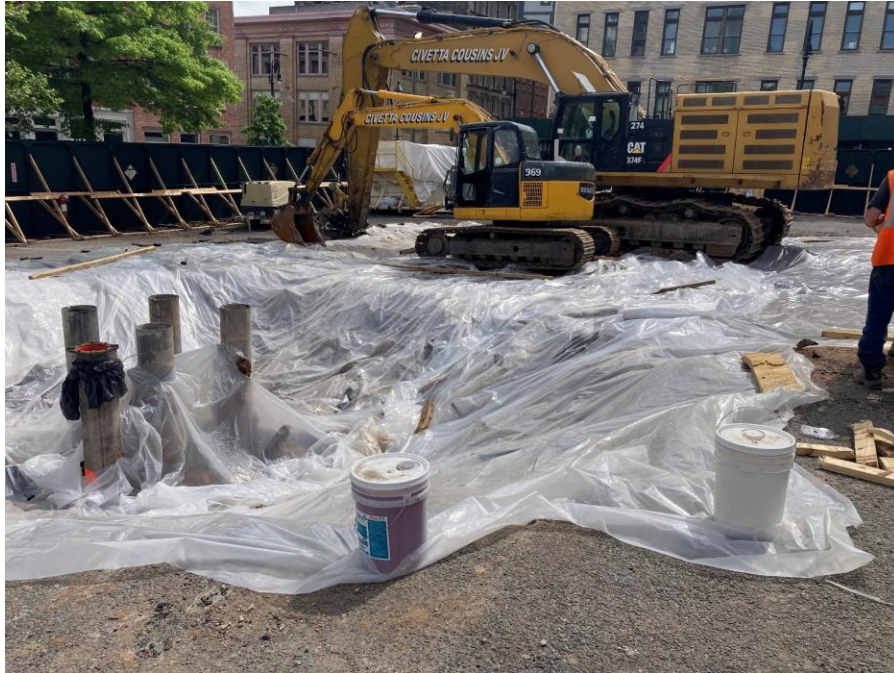
Photo 3: View of CCJV covering exposed soil/fill with polyethylene sheeting at the end of the work day (facing southwest)
