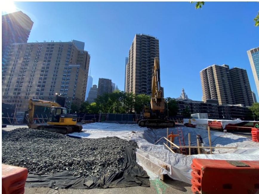
Photo 2: View of exposed soil/fill covered with polyethylene sheeting at the end of the work day (facing south)
