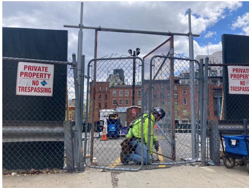
Photo 1: View of perimeter construction fencing being installed along the northern boundary the site (facing south).
