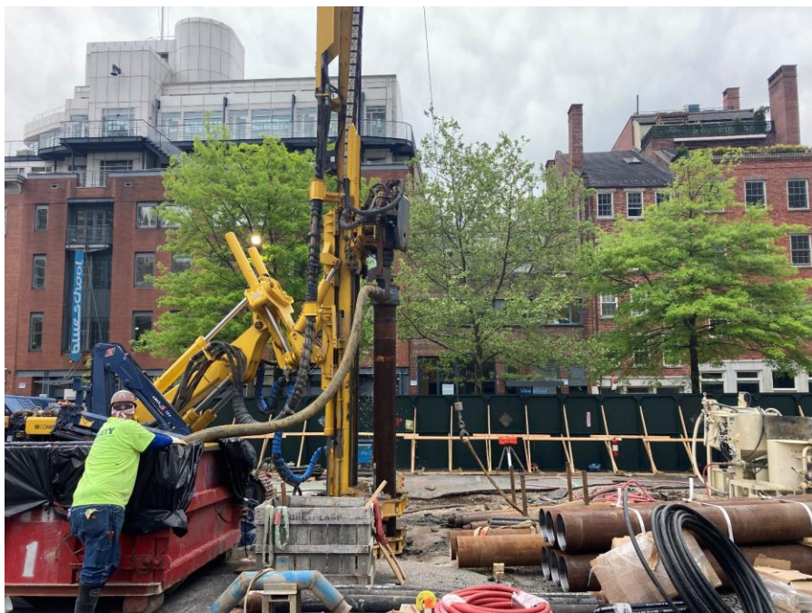
Photo 2: View of CCJV advancing a pile in the southwestern portion of the site (facing south)
