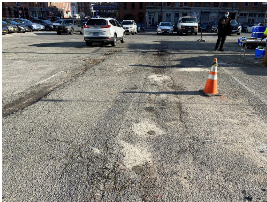
Photo 4: View of soil borings restored to surface grade with clean sand and concrete (facing south).
