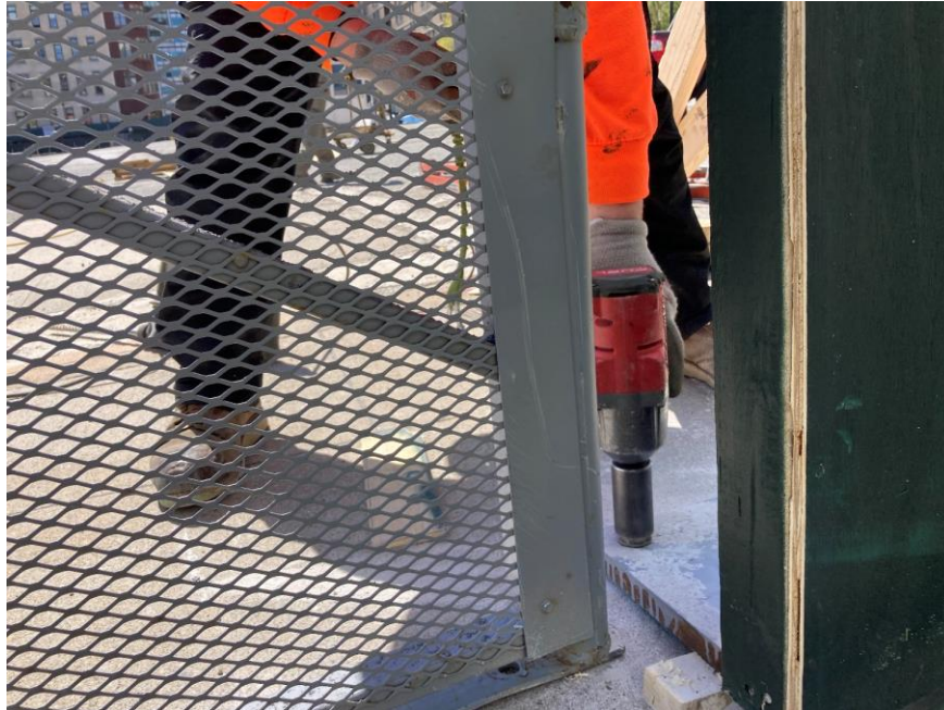
Photo 1: View installing 4-inch long bolts along the northern boundary the site (facing west).
