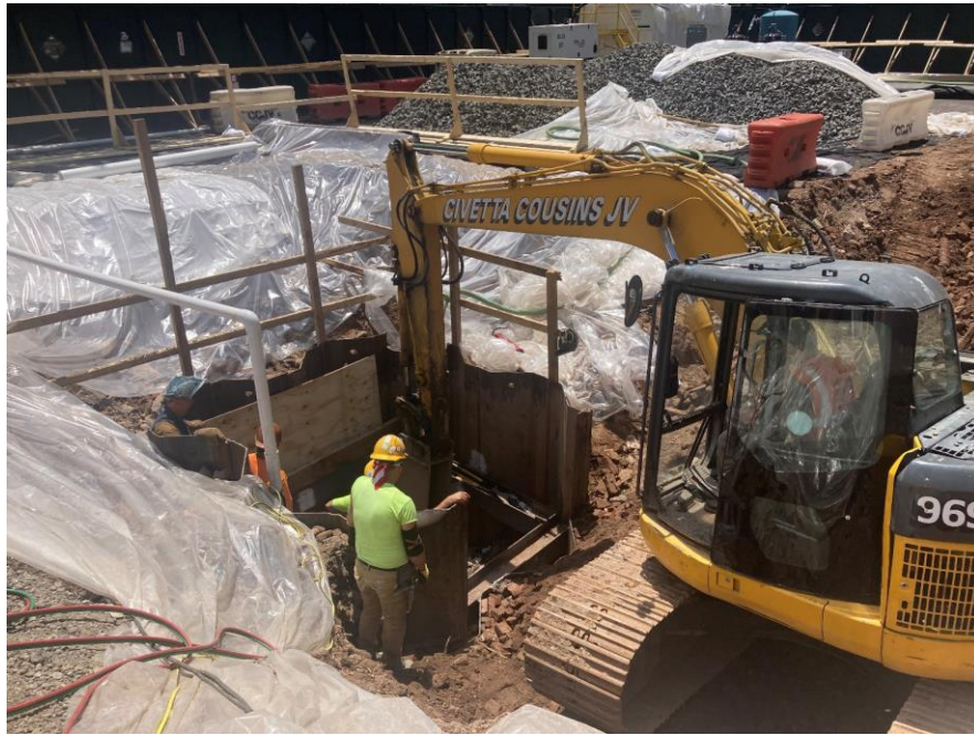
Photo 1: View CCJV excavating soil/fill between previously installed foundation piles in the southwestern portion of the site (facing southwest)
