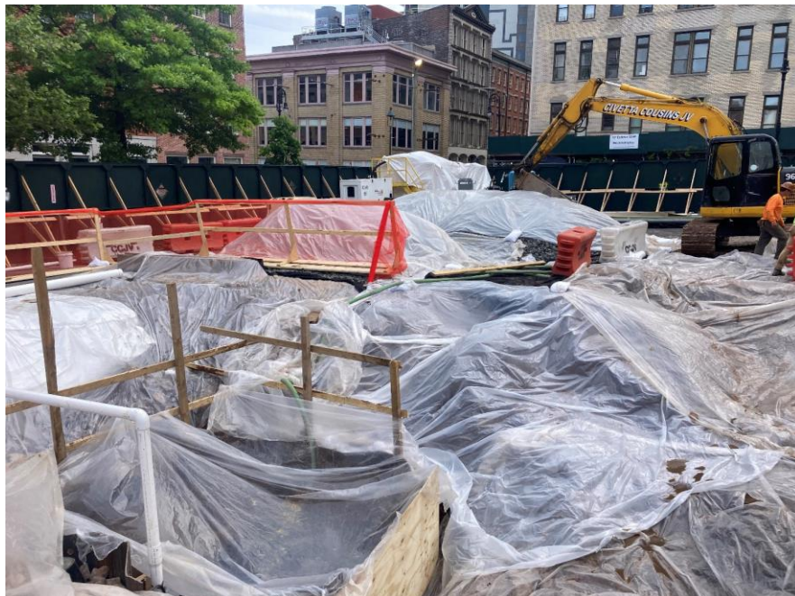
Photo 2: View of exposed soil/fill and imported virgin stone stockpiles covered at end of day (facing southwest).
