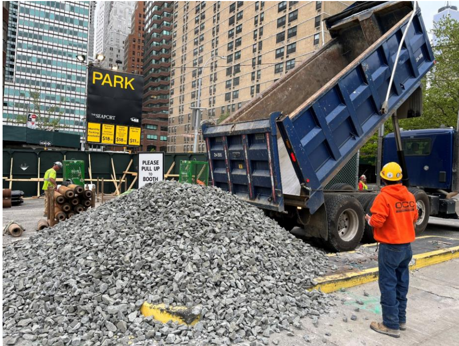
Photo 1: CCJV importing one truckload of 2.5-inch virgin stone for installation of a tracking pad in the northwestern portion of the site (facing northwest)
