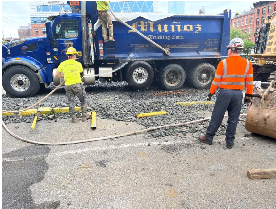
Photo 1: View of CCJV washing a truck prior to exiting the site (facing east)
