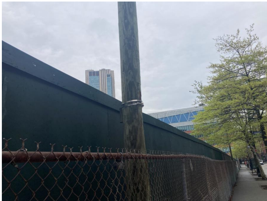
Photo 2: View of the completed perimeter construction fence along Water Street (facing east).
