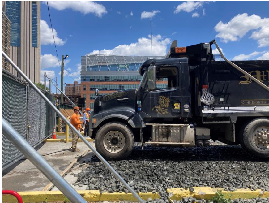
Photo 3: View of CCJV washing a truck prior to exiting the site (facing east).
