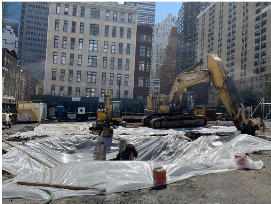
Photo 2: View of the covered excavation area at the end of the work day (facing south)
