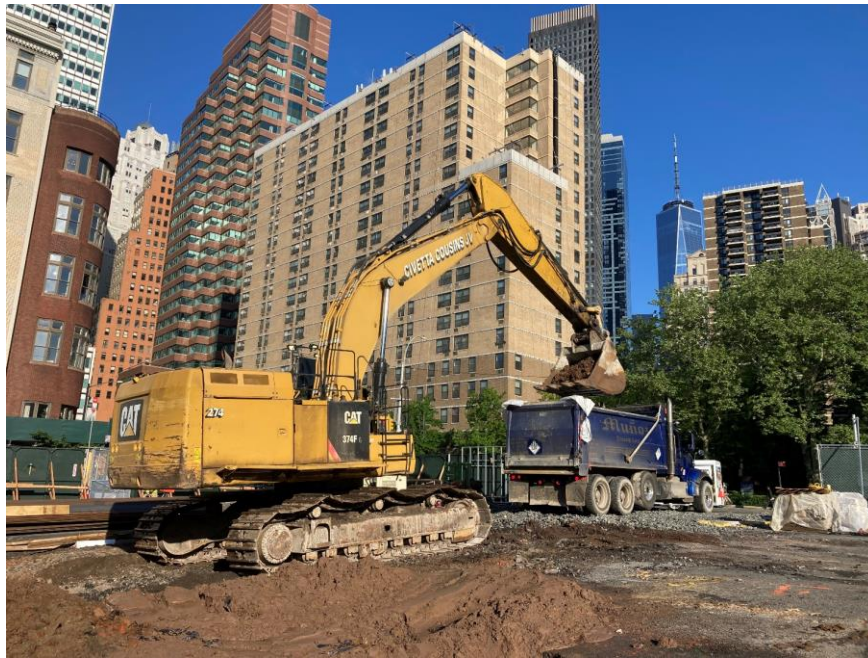
Photo 1: View of CCJV live-loading a permitted, tri-axle truck with hazardous lead-impacted soil/fill for off-site disposal (facing northwest)
