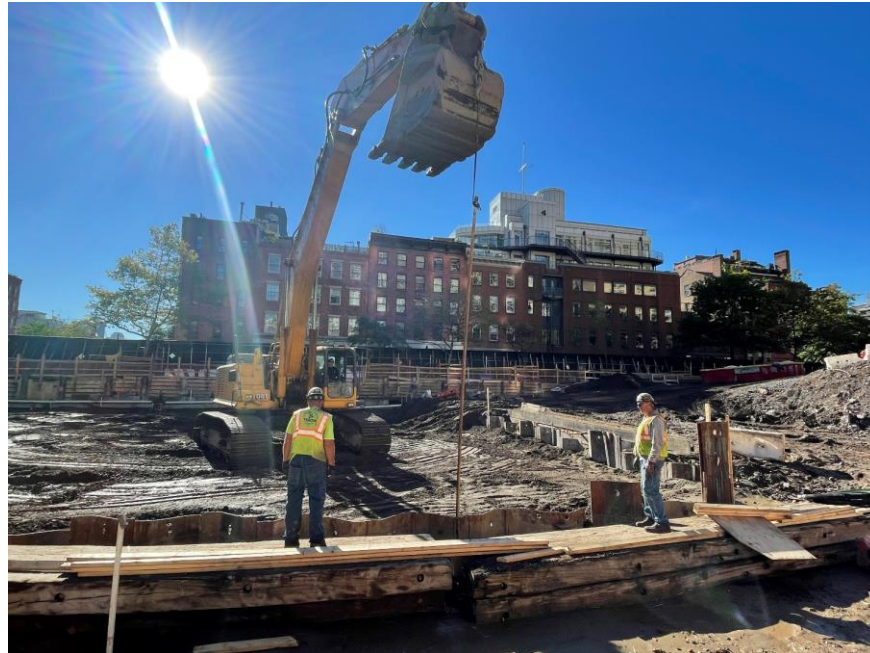
Photo 1: CCJV removing a dewatering well for disassembly of the dewatering system (facing south)
