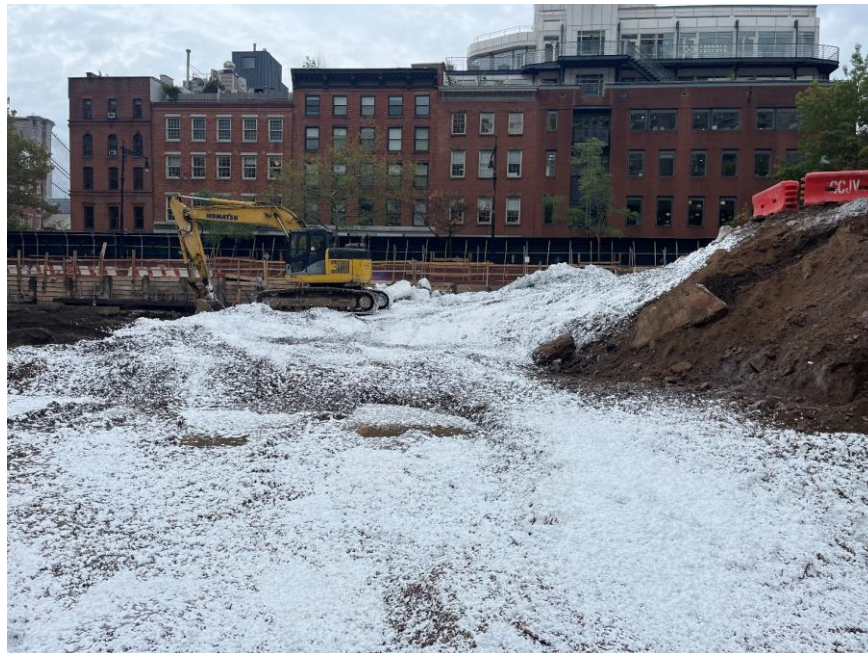
Photo 2: Atmos® AC-645 dust/vapor suppressing foam applied to exposed soil/fill for the temporary overnight cover (facing south)
