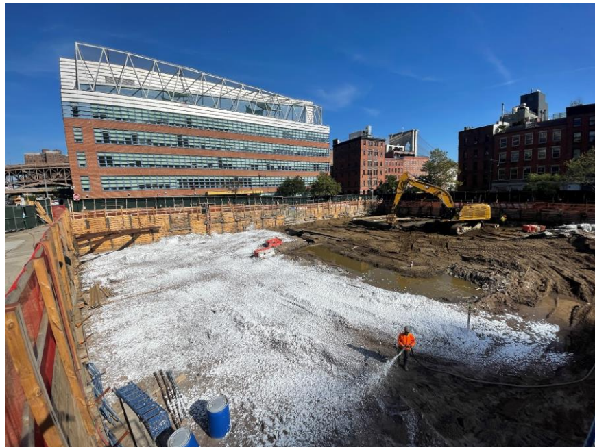
Photo 2: CCJV applying Atmos® AC-645 dust/vapor suppressing foam to exposed soil/fill for the temporary overnight cover (facing southeast)
