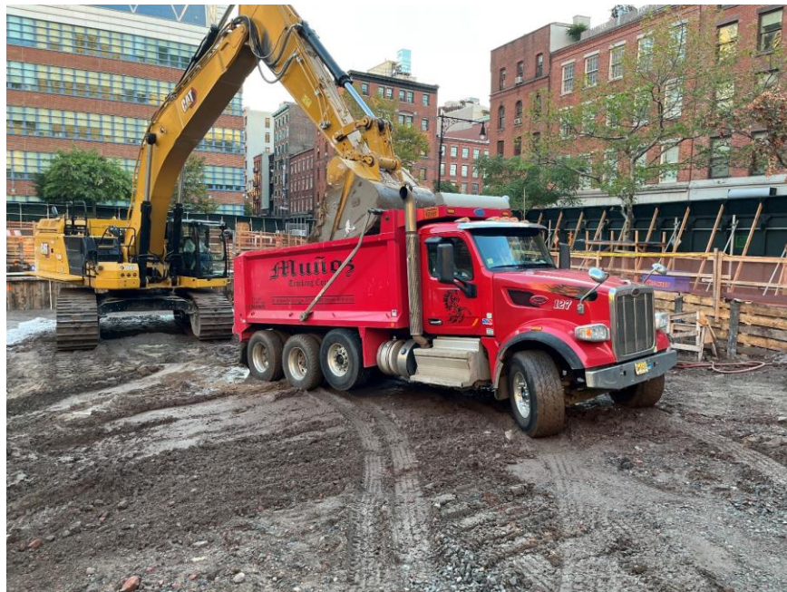
Photo 2: CCJV live-loading petroleum-impacted soil/fill into a tri-axle dump truck for off-site disposal (facing southeast)
