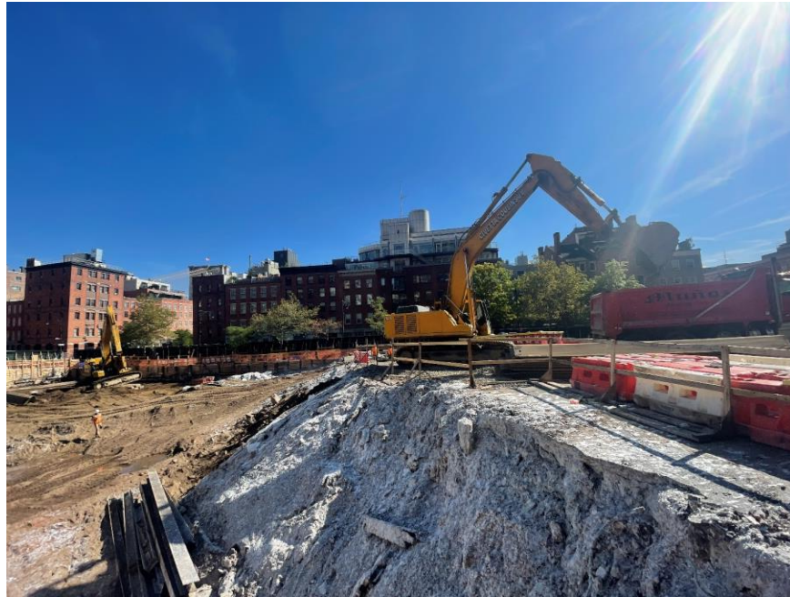
Photo 1: CCJV live-loading a dump truck with non-hazardous soil/fill for off-site disposal (facing south)
