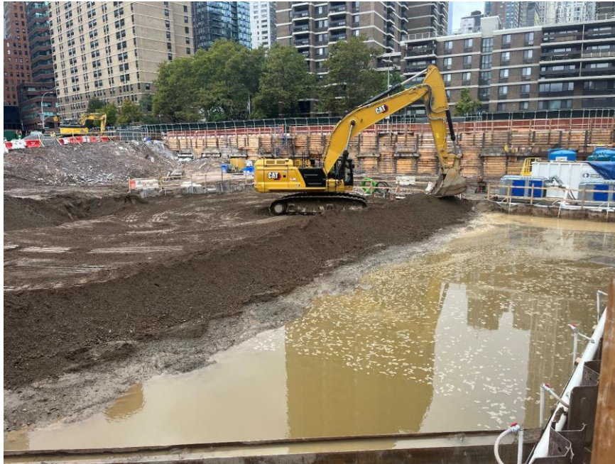
Photo 1: CCJV backfilling imported general fill in the southeastern part of the site (facing northwest)
