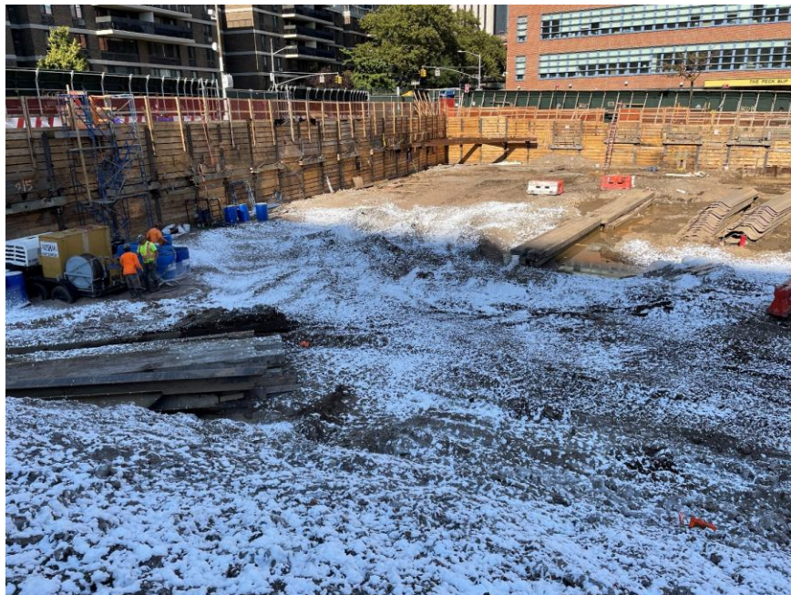
Photo 2: Exposed soil/fill covered in Atmos® AC-645 dust/vapor suppressing foam for the temporary overnight cover (facing northeast)
