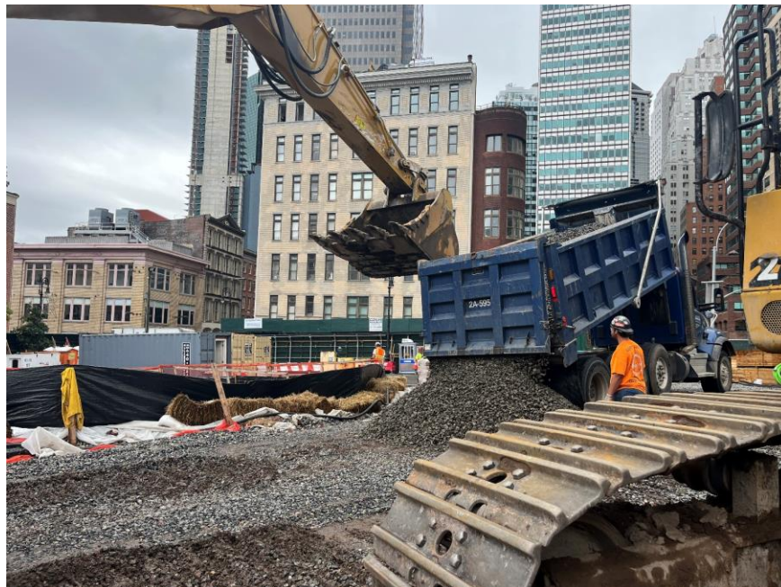
Photo 2: CCJV importing 1.5-inch clean bluestone for maintenance of the tracking pad in the northwestern part of the site (facing northwest)
