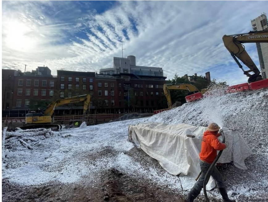
Photo 1: CCJV applying Atmos® AC-645 dust/vapor suppressing foam for reinstatement of the temporary overnight cover (facing southwest).
