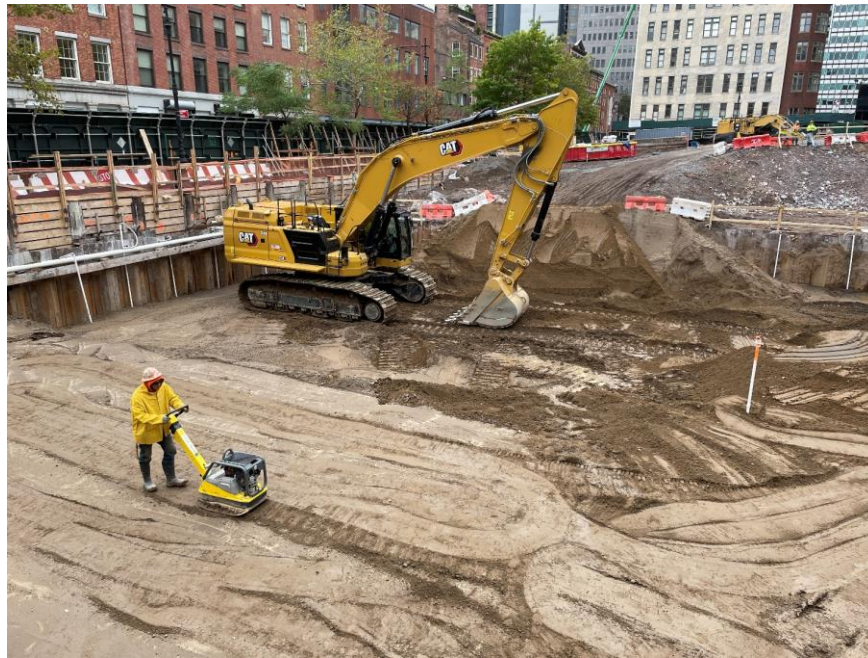
Photo 1: CCJV backfilling and compacting imported general fill in the southeastern part of the site (facing southwest)
