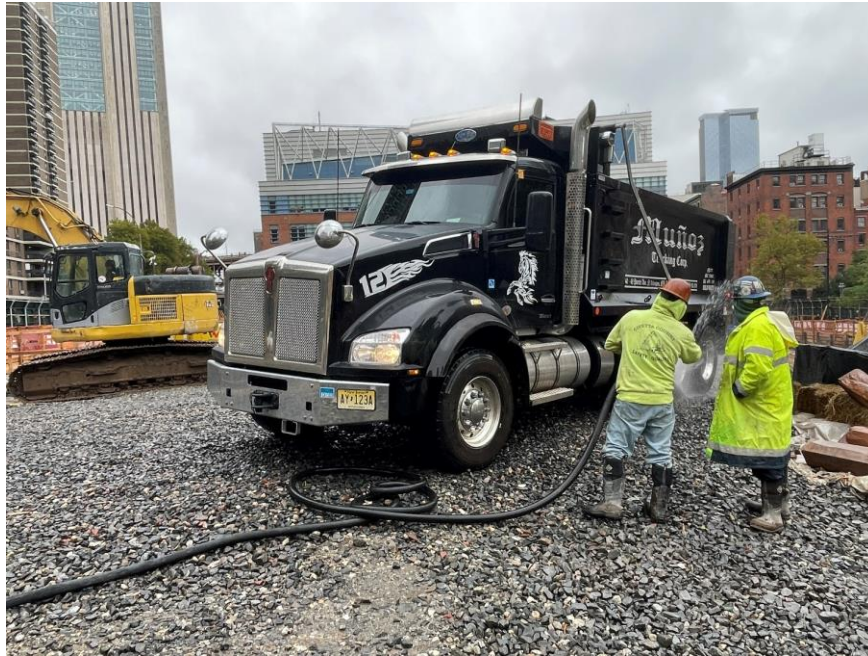
Photo 1: CCJV washing and inspecting truck prior to exiting the site (facing east)
