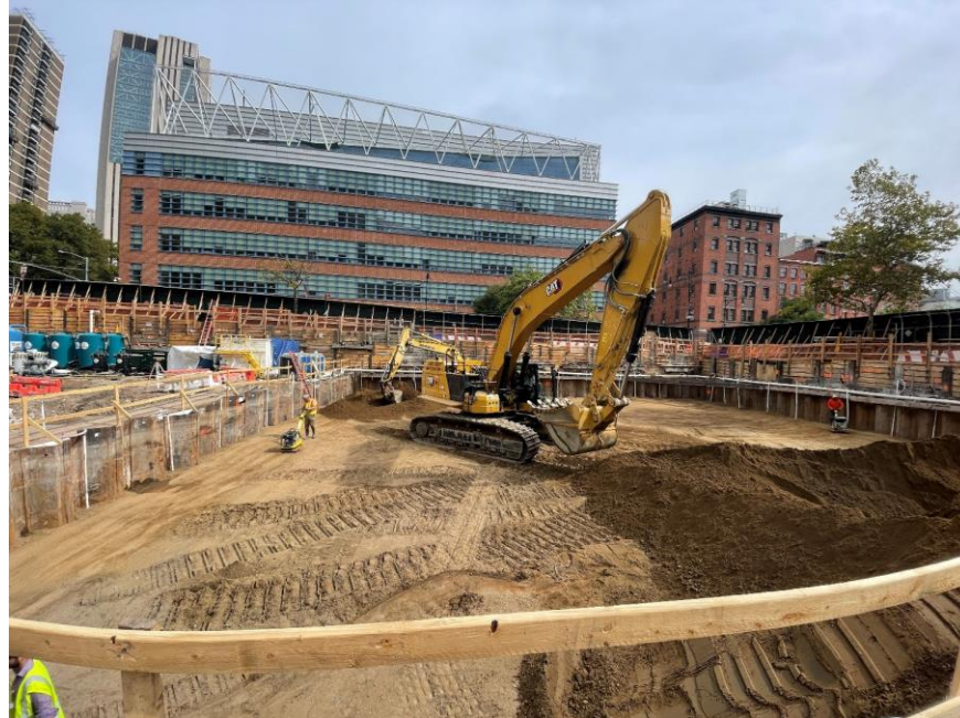
Photo 1: CCJV backfilling and compacting general fill in the southeastern part of the site (facing east)
