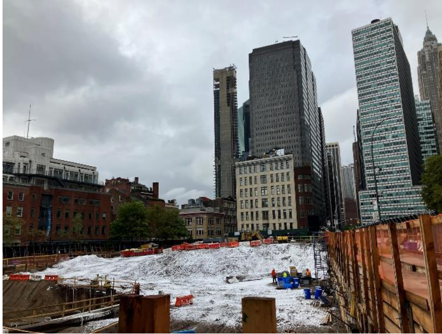
Photo 1: CCJV applying Atmos® AC-645 dust/vapor suppressing foam to exposed soil/fill to create a temporary overnight cover (facing west).
