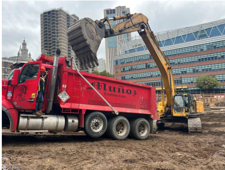
Photo 1: CCJV live-loading a dump truck with hazardous lead-impacted soil/fill for off-site disposal (facing east)
