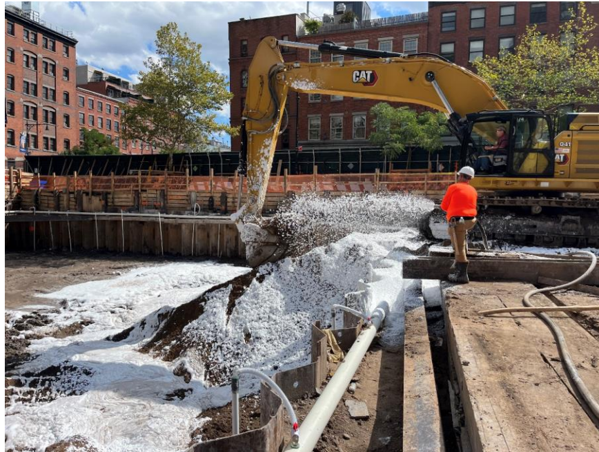
Photo 1: CCJV actively applying Atmos® AC-645 dust/vapor suppressing foam to exposed soil/fill during excavation and loading activities (facing south)
