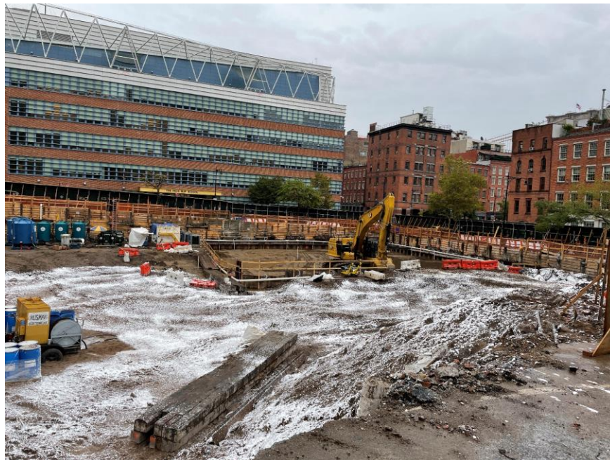
Photo 2: Exposed soil/fill covered in Atmos® AC-645 dust/vapor suppressing foam for the temporary overnight cover (facing southeast)
