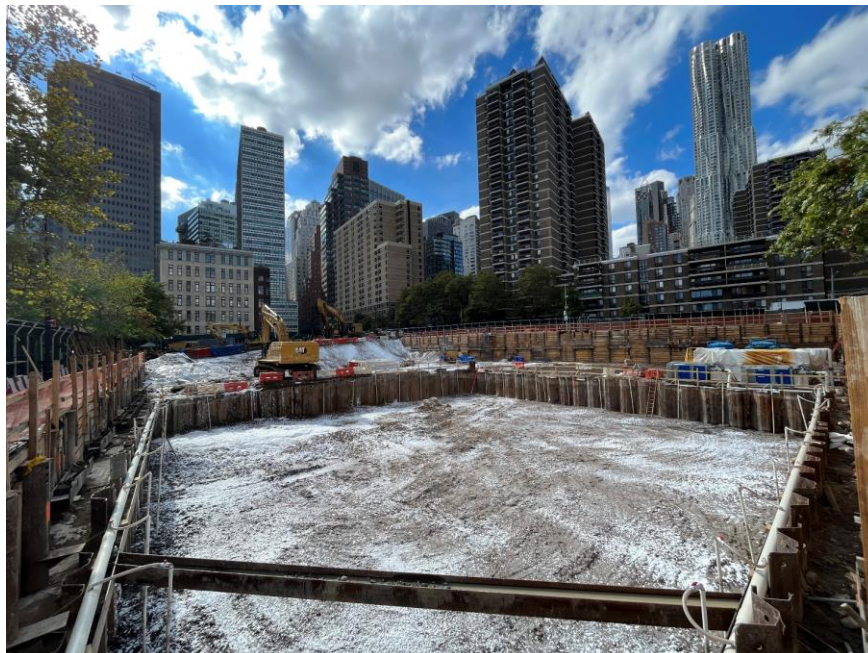
Photo 2: Excavation progress in the southeastern part of the site (facing northwest)
