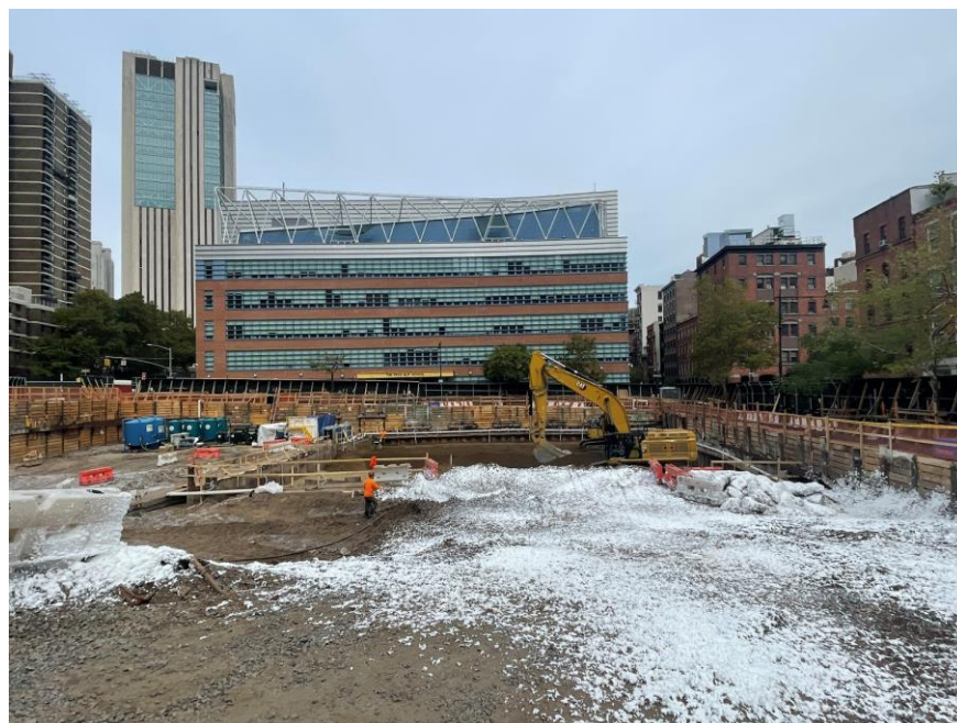
Photo 2: CCJV applying Atmos ® AC-645 dust/vapor suppressing foam to exposed soil/fill to create a temporary overnight cover (facing east)
