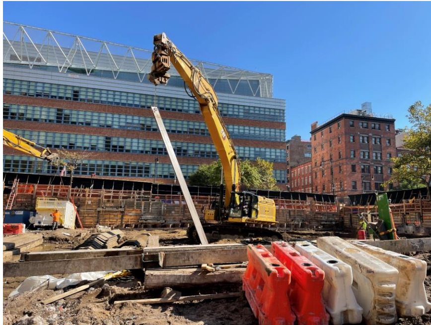
Photo 1: CCJV removing previously installed steel sheet piles in the southeastern part of the site (facing east)
