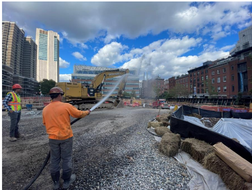
Photo 2: CCJV implementing dust suppression along the truck tracking pad in the northwestern part of the site (facing east)
