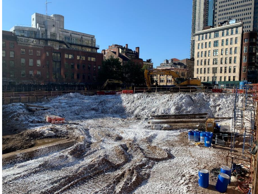
Photo 1: Atmos® AC-645 dust/vapor suppressing foam applied to exposed soil/fill for the temporary overnight cover (facing southwest)
