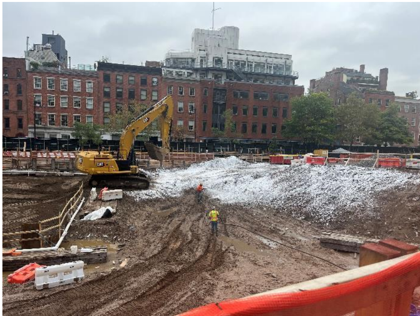
Photo 2: CCJV applying Atmos® AC-645 dust/vapor suppressing foam to exposed soil/fill to create a temporary overnight cover (facing south)
