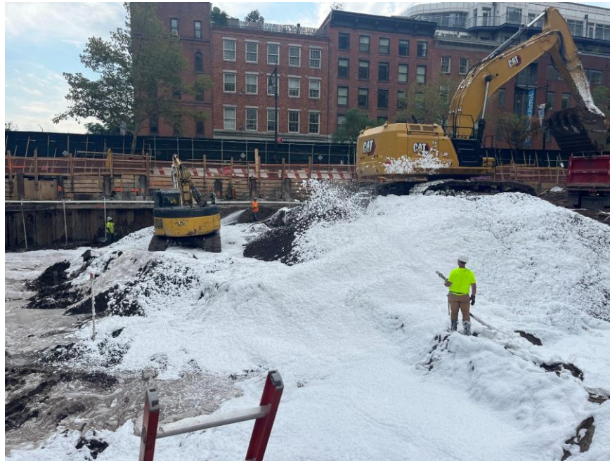
Photo 1: CCJV actively applying Atmos® AC-645 dust/vapor suppressing foam during excavation/loading in the southeastern part of the site (facing south)
