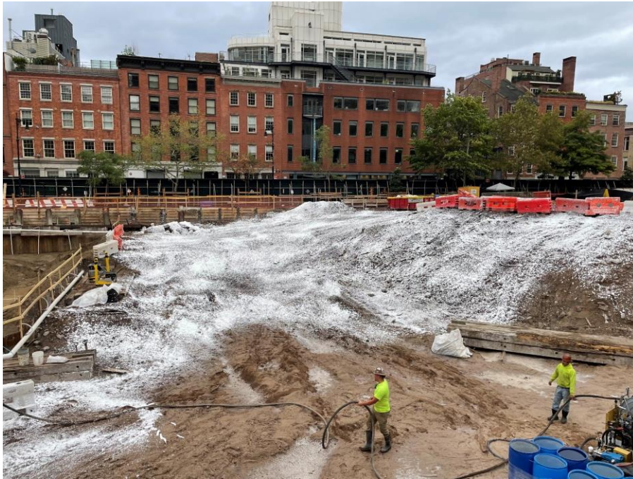
Photo 1: CCJV applying Atmos® AC-645 dust/vapor suppressing foam to exposed soil/fill to create a temporary overnight cover (facing south).
