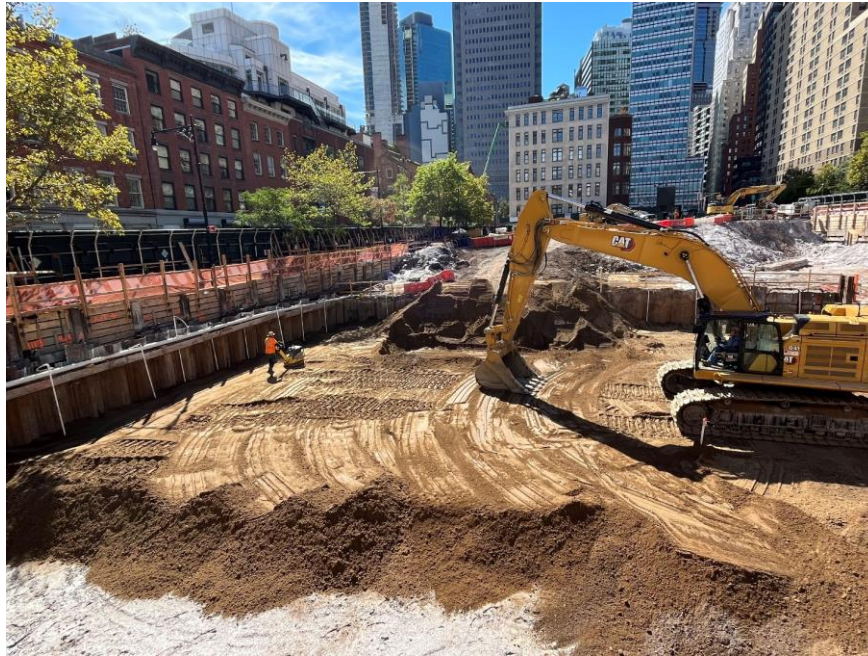
Photo 1: CCJV grading and compacting the backfilled general fill in the southeastern part of the site (facing west)
