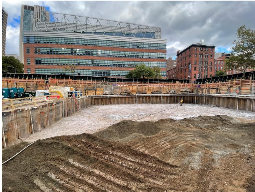
Photo 1: Backfill progress in the southeastern part of the site and CCJV applying Atmos ® AC-645 dust/vapor suppressing foam to exposed soil/fill to create a temporary overnight cover (facing east)
