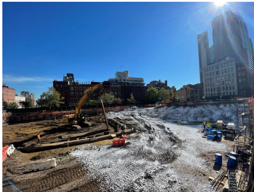
Photo 2: CCJV applying Atmos ® AC-645 dust/vapor suppressing foam to exposed soil/fill to create a temporary overnight cover (facing southwest)
