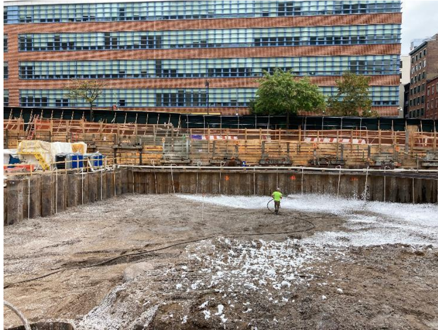
Photo 1: CCJV applying Atmos® AC-645 dust/vapor suppressing foam for reinstatement of the temporary overnight cover (facing east).
