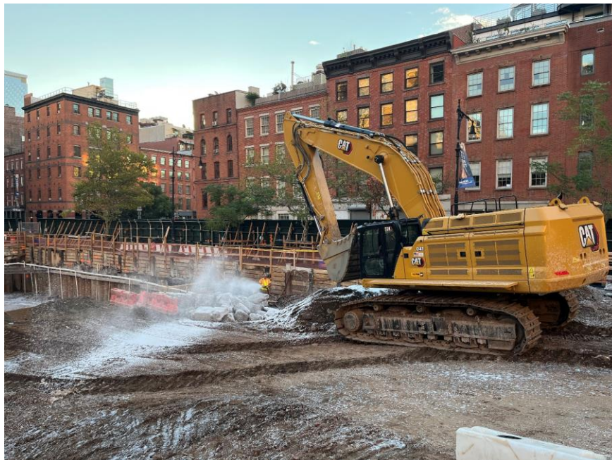
Photo 2: CCJV actively applying Atmos® AC-645 dust/vapor suppressing foam during excavation and loading of previously stockpiled hazardous lead-impacted soil/fill (facing southeast)
