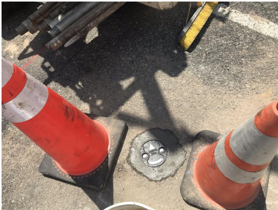
Photo 2: Monitoring well MW25 installed by AARCO
