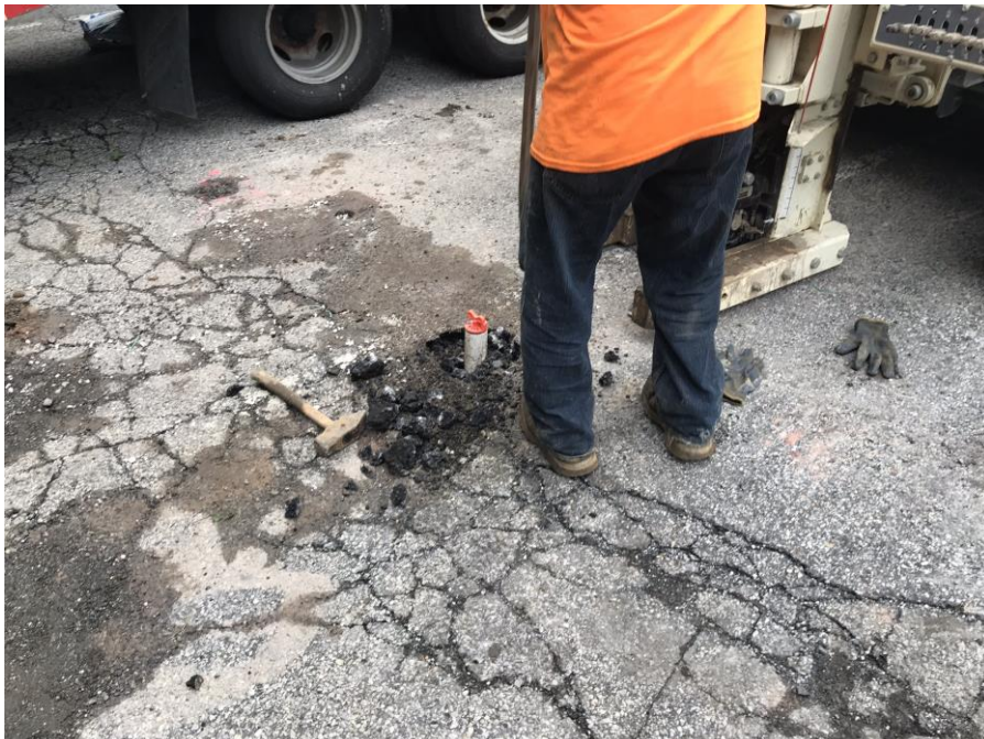
Photo 2: AARCO installing monitoring well MW17 (facing northwest)
