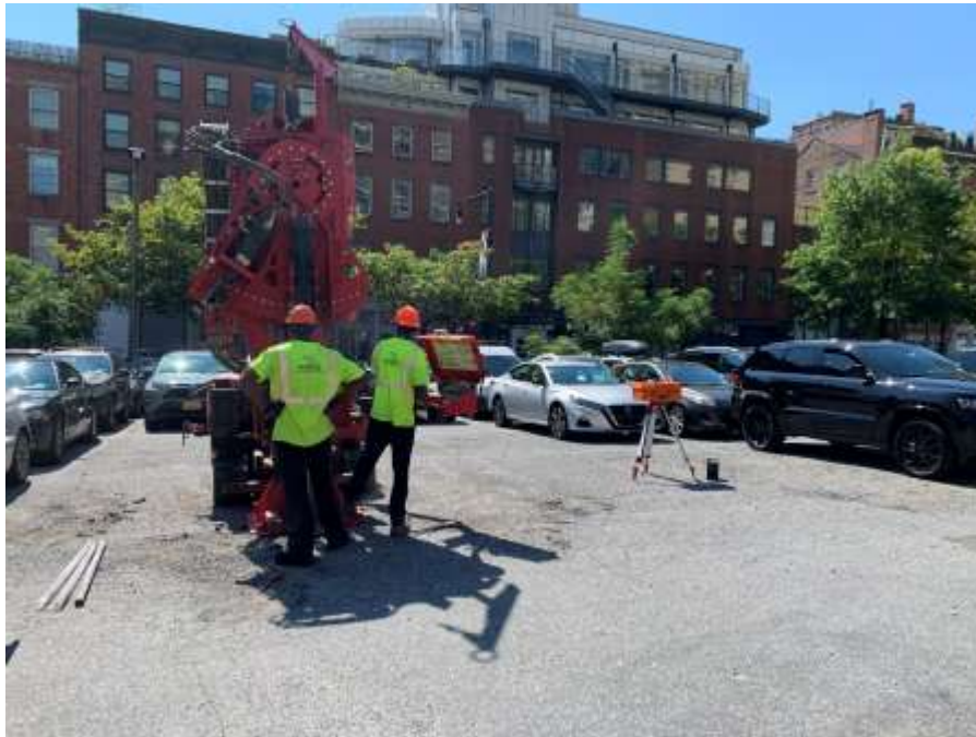
Photo 3: AARCO drilling boring SB26 (facing southeast)
