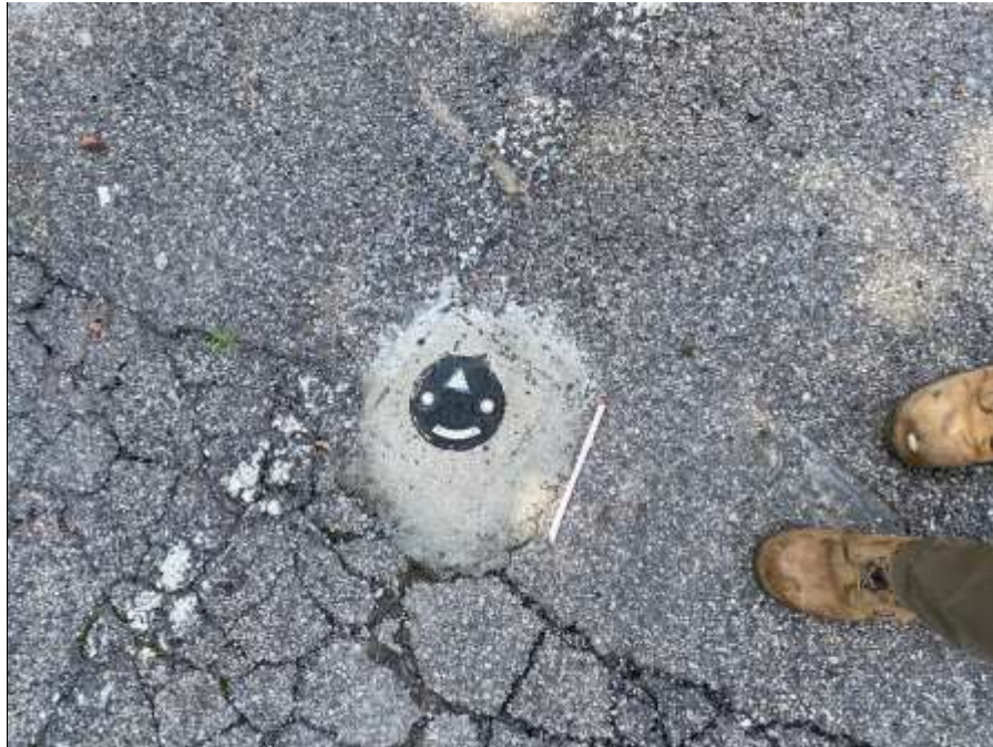
Photo 1: Monitoring well MW17
