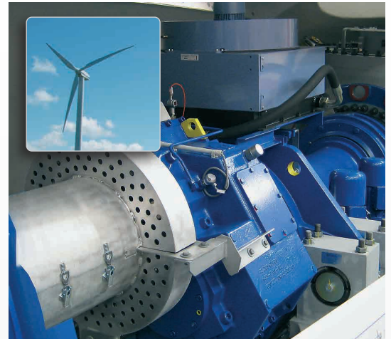
Easy-Laser® is used to align generators and gearboxes in wind turbines of a number of sizes and makes. Special brackets are available (accessories) for alignment with locked rotors, which increases the safety for the operator.
