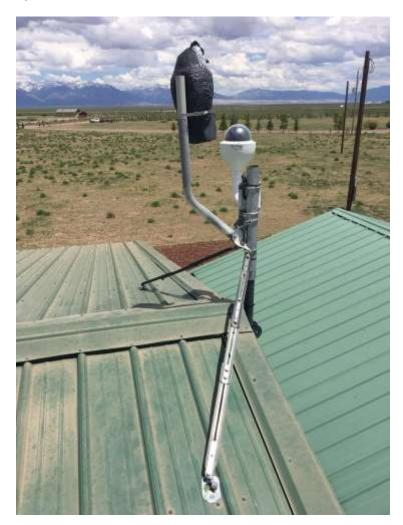
The optional addition of the owl can sometimes be helpful to prevent birds from landing on the dome, leaving behind residue that can obscure the view. Outdoor installations in environments known for potential lightening action should provide for proper surge suppression. One way to accomplish this is to use a goodquality surge suppressor near the MSDAU/Camera and another at the entrance to the structure where the Ethernet cable will attach to the router. One such suppressor is shown below.
