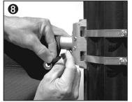
Using Duct Tape (K), temporarily hold casting(s) in place against utility pole at desired height. The word "TOP" on the Main Pole Casting (A) must be pointing up at ALL times for both Main Castings at both upper and lower locations.
