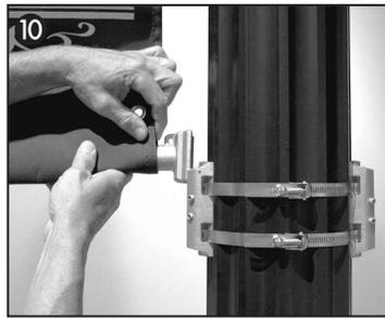
**8** Feed the Nylon Cable Tie (L) [or 18 gauge or larger galvanized wire] through the banner grommet and through the “eye” hole in the Arm Casting. This attachment is required to prevent the banner from sliding off.
