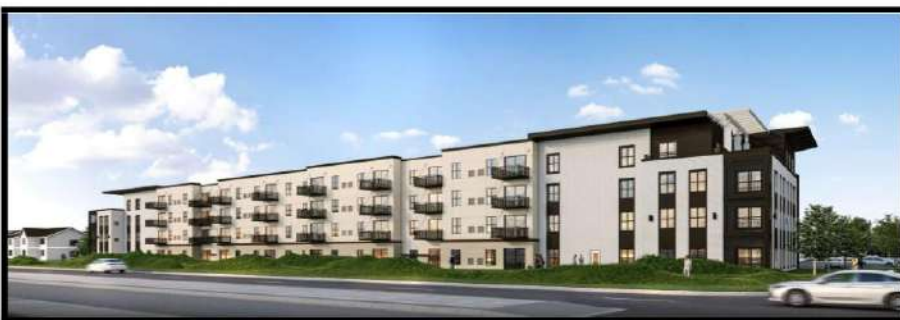
View from Bielenberg Drive
