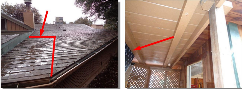
Location: South Rear of Garage
