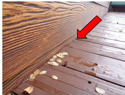
Comment: FLASHING MISSING BETWEEN DECK AND SIDING – this helps reduce dry rot.
