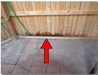
Location: South Rear of Garage
