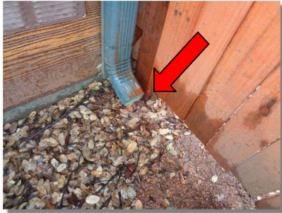
Location: West Right of Building
