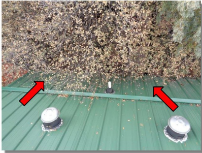
Location: Roof, Southwest Corner of Building
