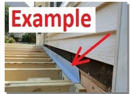
Comment: FLASHING MISSING BETWEEN DECK AND SIDING – this helps reduce dry rot.
