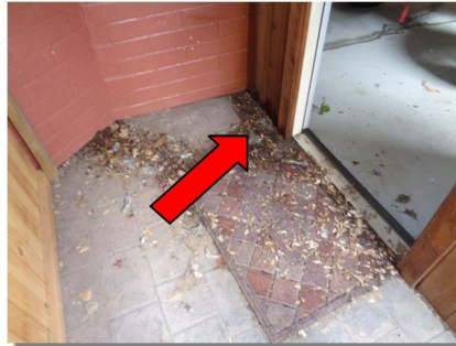
Location: Backside of garage
