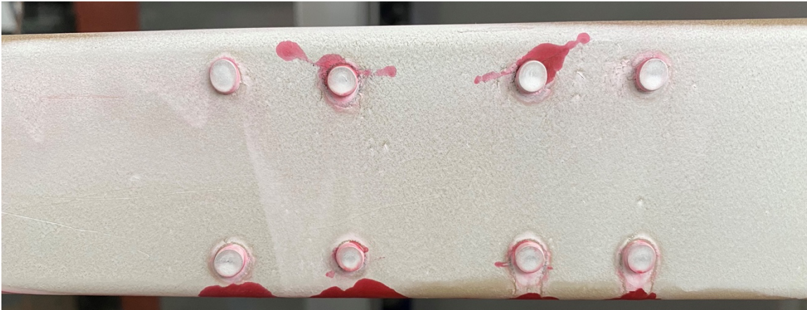
FIGURE 4 - EXAMPLE 2 - CRACK LOCATIONS - FWD SIDE OF SPAR
